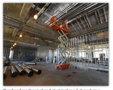
Overhead mechanical and electrical conduit are being installed. Interior framing on this level is nearly complete.
