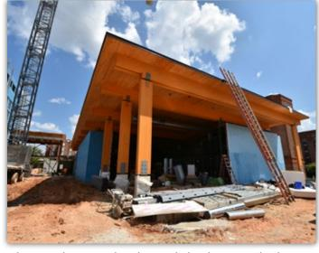
The cross-laminated timber and glue-laminated column and beam structure of the Hey Day Market nears completion.
