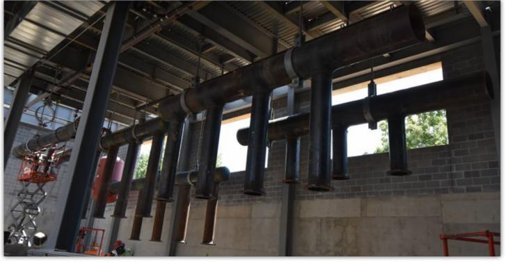
Piping for the new chiller units is in place awaiting chiller installation.
