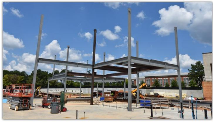
Steel erection has begun for the locker room, equipment storage and main utility areas.
