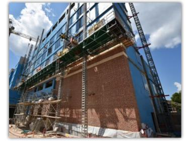
Brick work has begun on the outside of the Center, and windows have been installed.
