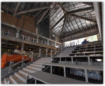
Framing for the atrium is being completed while a set of stairs has been placed leading to the upper floor.
