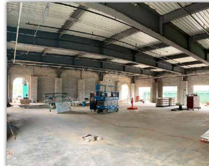
Mechanical, electrical and plumbing work continues inside the new facility.
