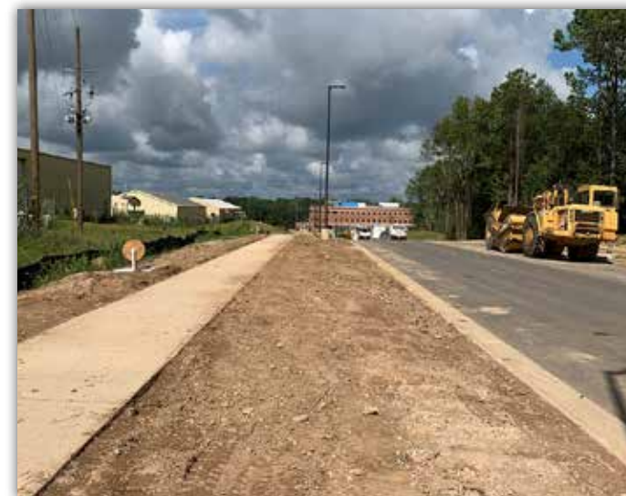
Sidewalks and light poles have been installed.
