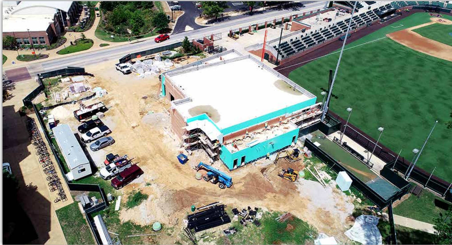
The Plainsman Park Player Development Building is located just outside of right field.
