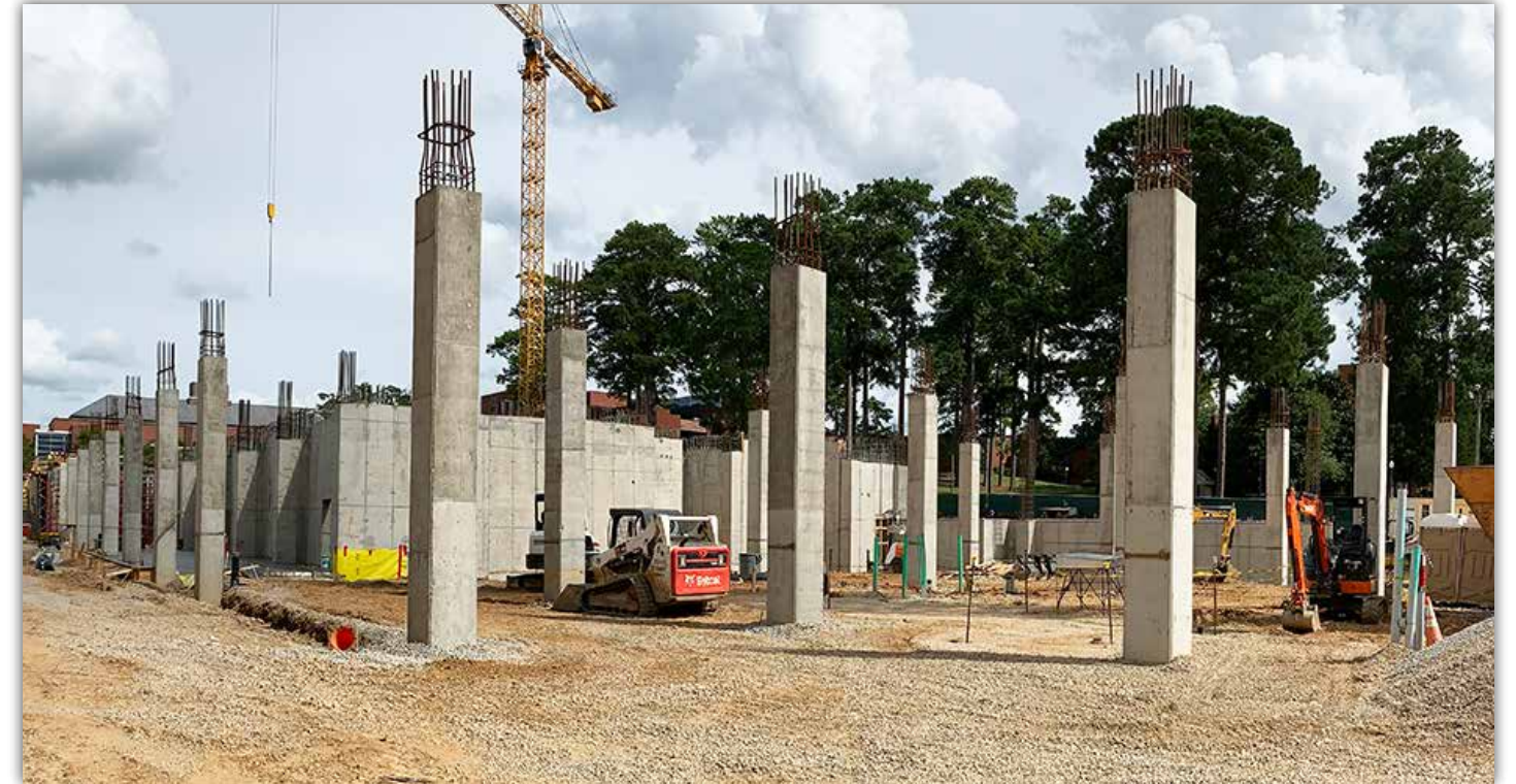
These concrete columns will support the first floor.
