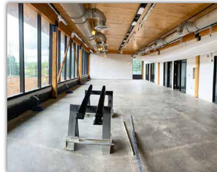
The windows and cross-laminated timber (CLT) ceiling have been installed in the open office area. This is the first building on campus to include a CLT structure.
