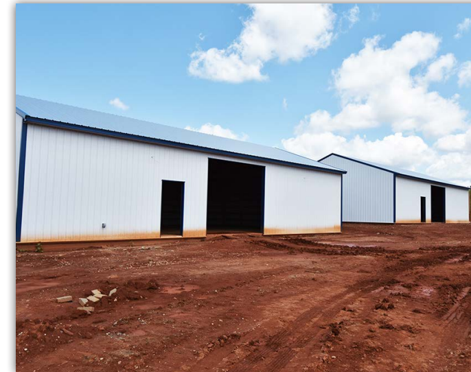
An exterior view of two pole barns.
