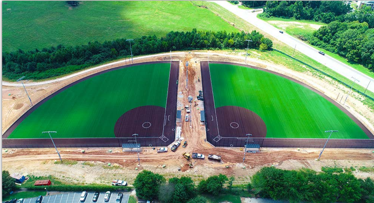
The two softball fields located next to Wire Road are complete.
