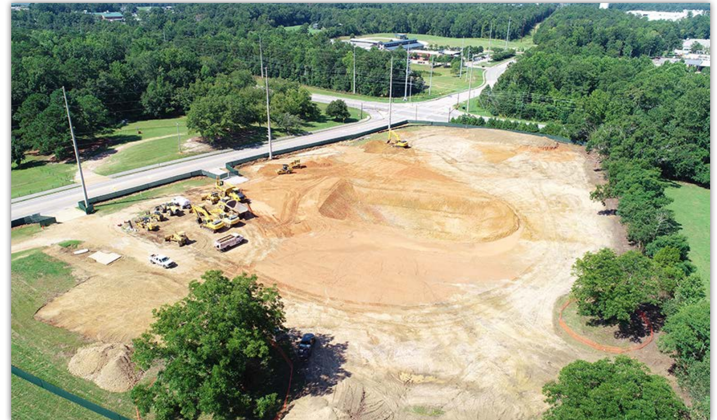
Site work is now underway for excavation of the basement level.
