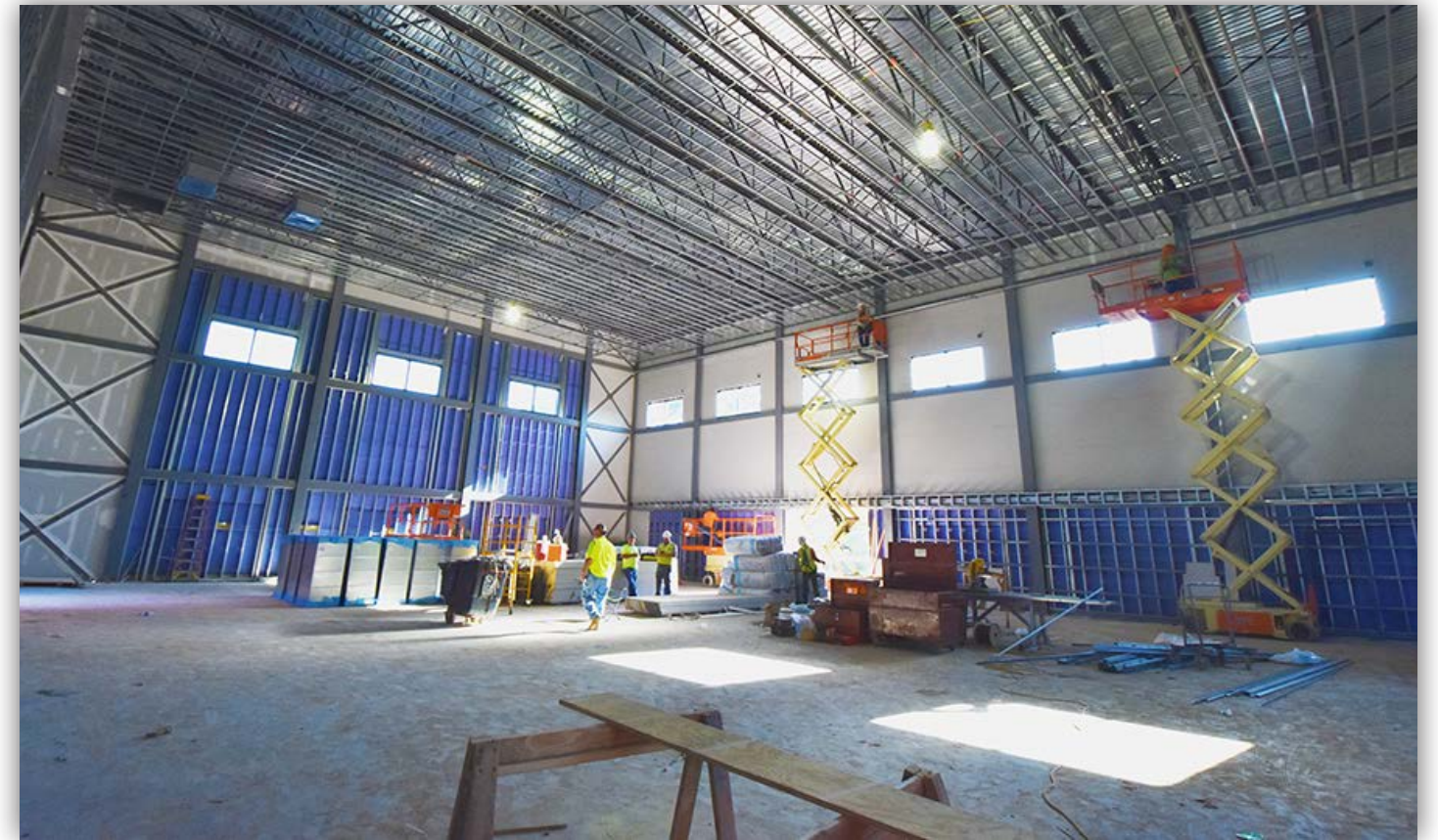
The main rehearsal hall walls and ceilings are fully framed.
