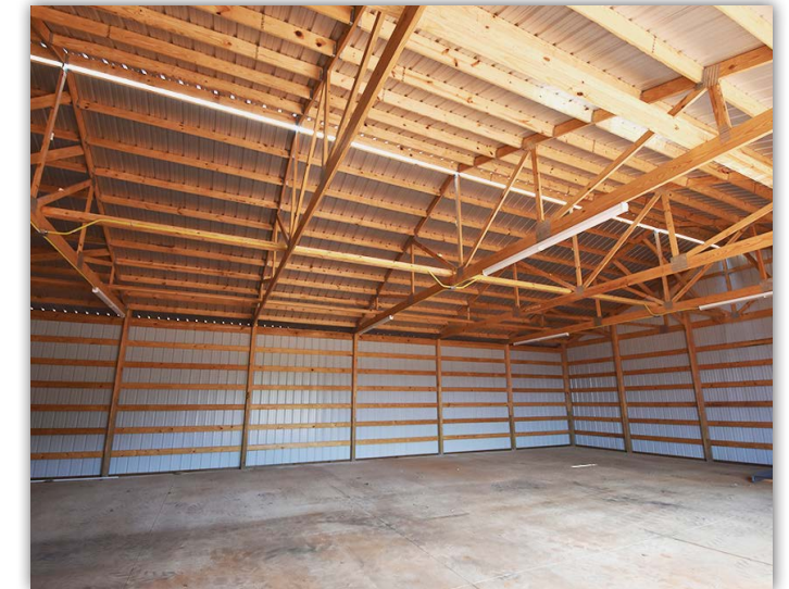
The walls and roofs are complete for each pole barn.
