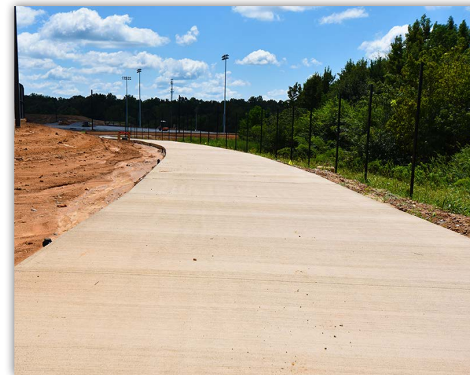
The perimeter sidewalk, that will wrap around the park, is ongoing.
