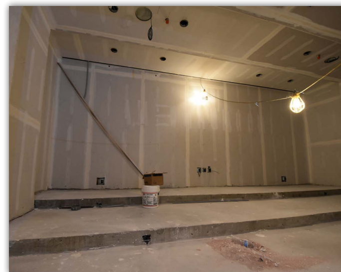
The team meeting room is framed and ready for paint.
