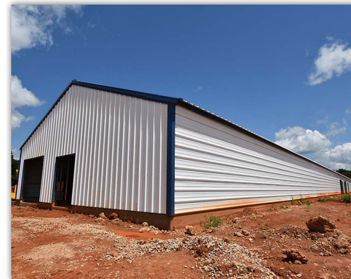
An exterior view of the battery house.
