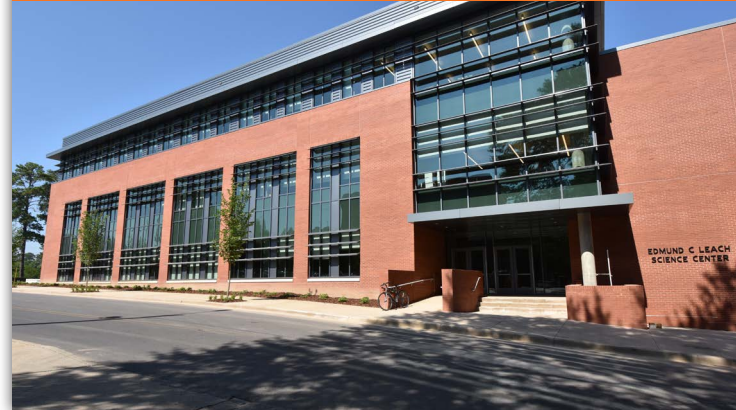
Leach Science Center Addition
