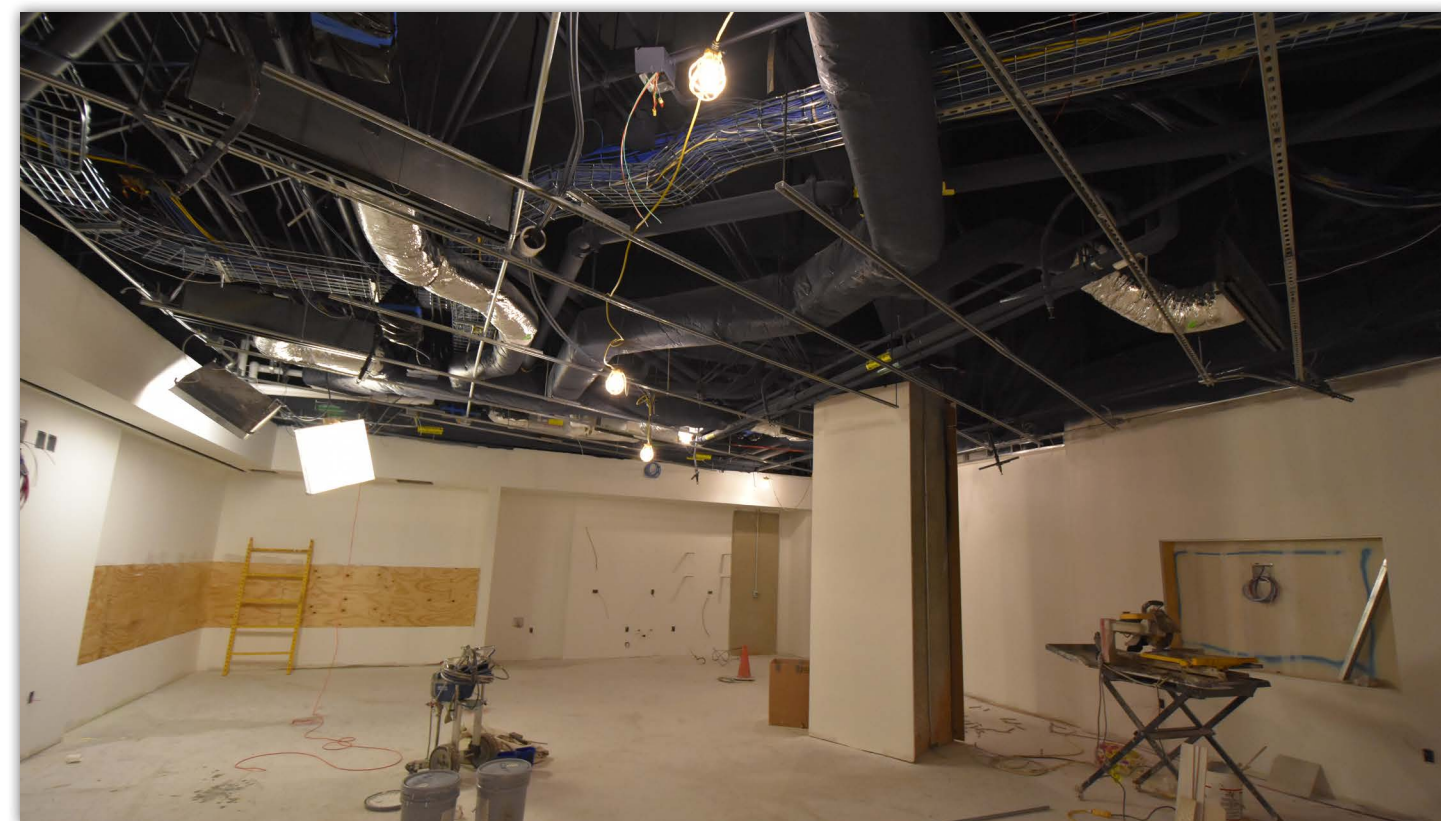
Painting is underway in the team lounge.
