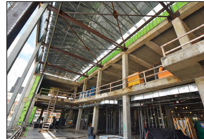
The metal roof now covers the entrance area.
