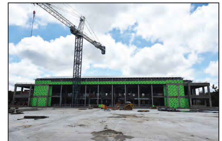
A view of the building as seen from the courtyard area.
