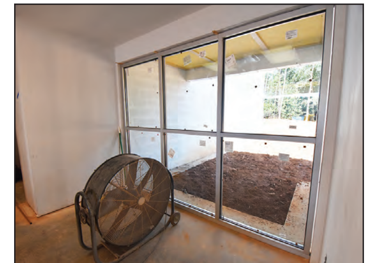
A view to the outside through newly installed windows.
