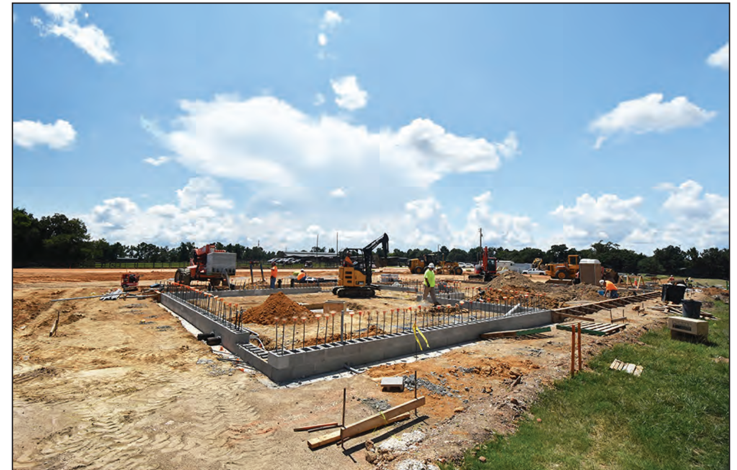
Forming of the team support building's concrete block foundation has begun.
