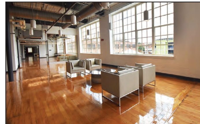
Furniture is being installed in the open study spaces.
