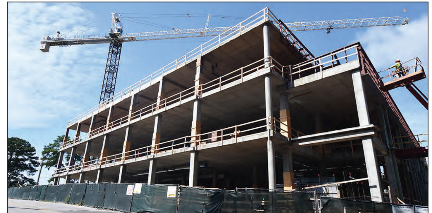
A view of the concrete structure as seen from Duncan Drive.
