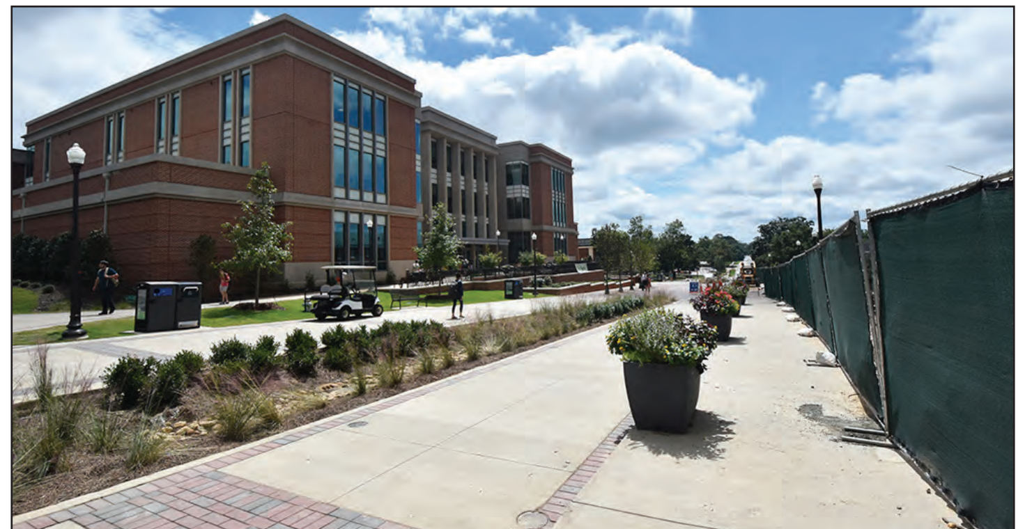
Self-watering planters and an eco swale help make the concourse green and sustainable.
