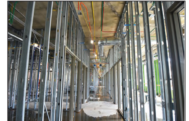
Metal wall framing on the first floor.
