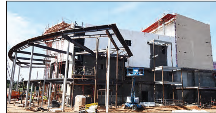
Steel framing has begun for the atrium.
