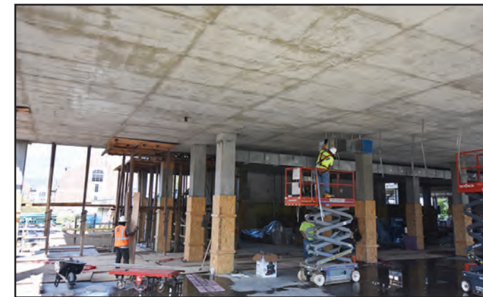
Contractors are installing overhead mechanical and electrical systems.
