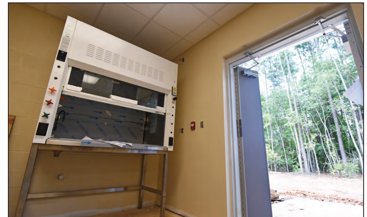
A fume hood is being installed in one of the laboratories.
