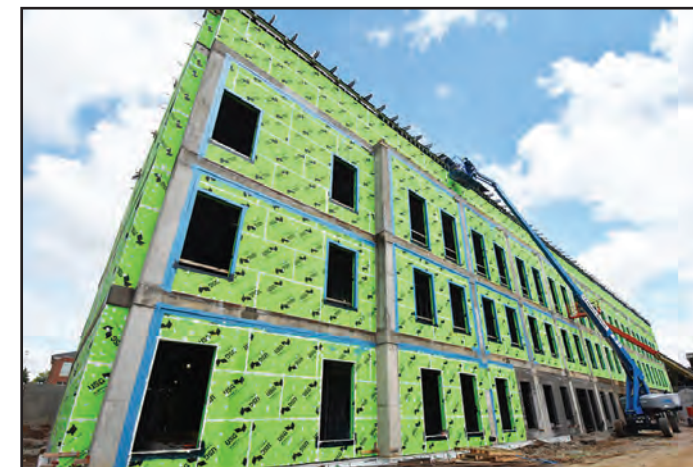
Green insulation covers the building's exterior.
