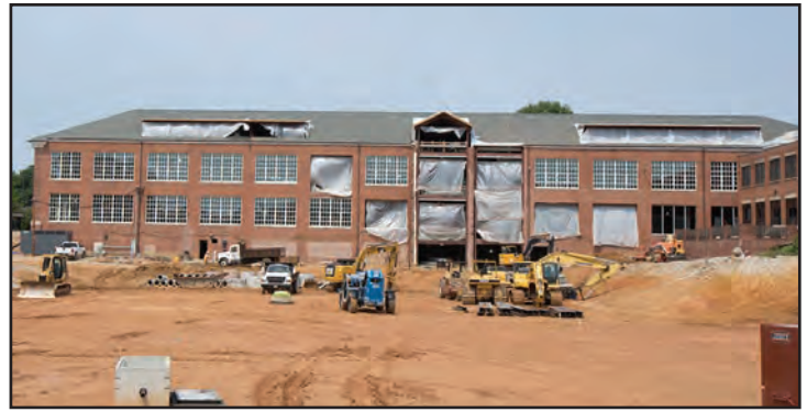
Construction of the new roof dormers and gable (center) have begun.
