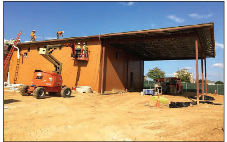
The safe room addition can be seen from behind the building.
