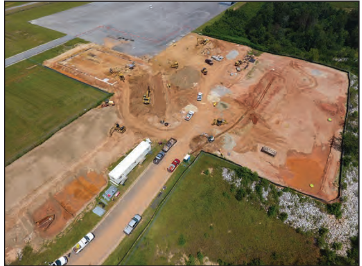
Aerial view shows site work has begun.
