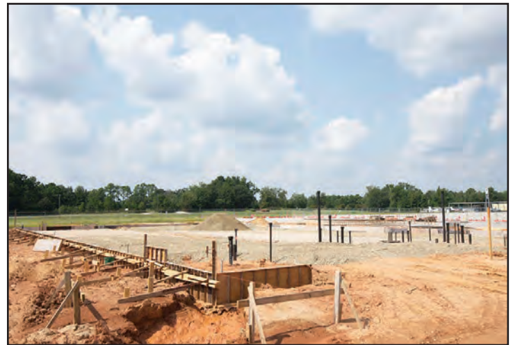
Building foundations are in place for the new maintenance hangar.
