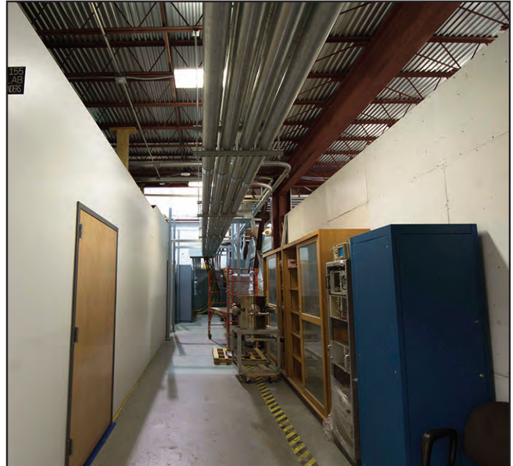
New electrical conduit is being installed in the ceiling.
