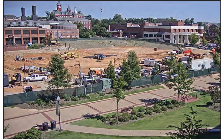
View of the Brown-Kopel construction site from the Shelby Center webcam.
