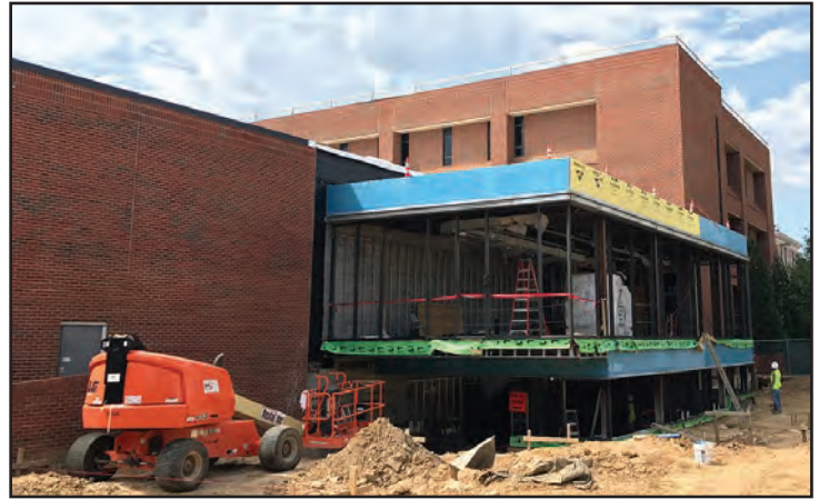
The pavilion structural steel has been erected.
