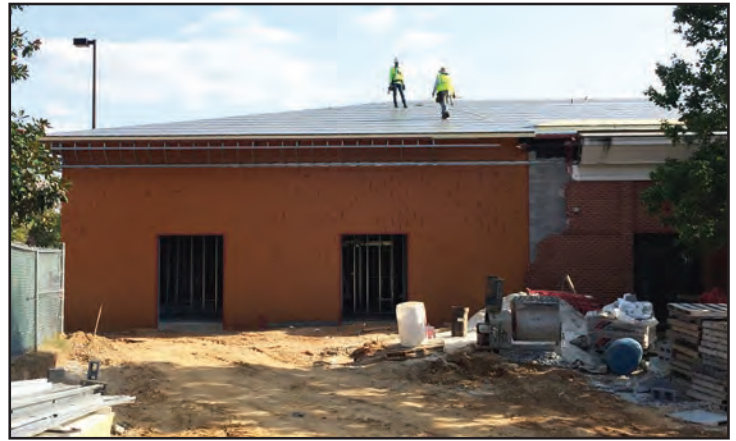
View of the Campus Safety Building expansion from Magnolia Avenue.
