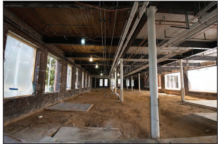
Demolition of the structurally unsound concrete slabs/foundation.
