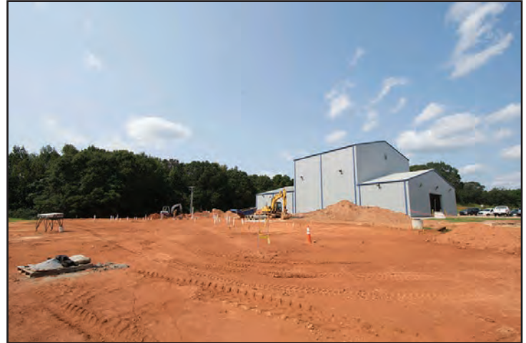
Below grade utilities are being installed at the site.
