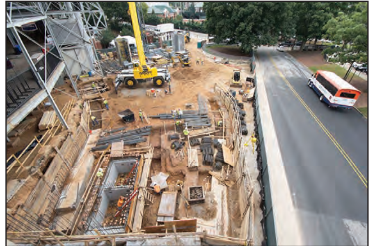
Concrete foundations have been poured in preparation for structural beams.
