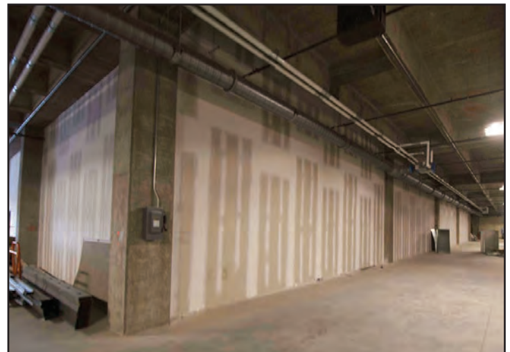
Exterior walls of the renovation project.
