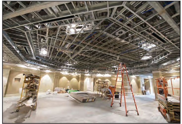
New structural steel installation in the Conference Center lobby.
