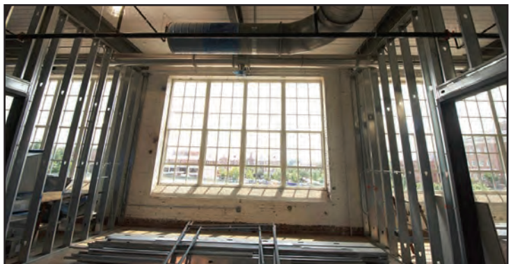
Installation of the building's new windows is almost complete.
