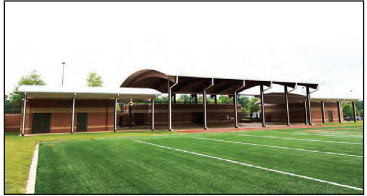
The women's (left) and men's (right) dressing rooms.
