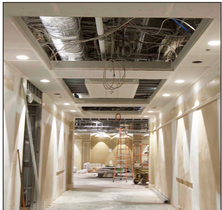
Above ceiling work continues in the main hallway.
