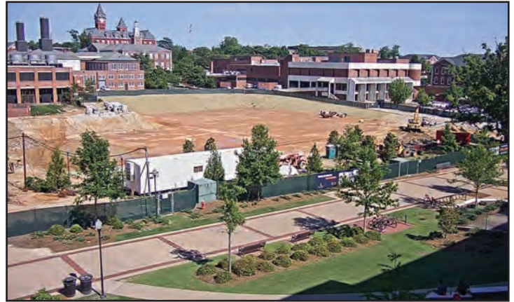
Site work nearing completion after demolition of the building.
