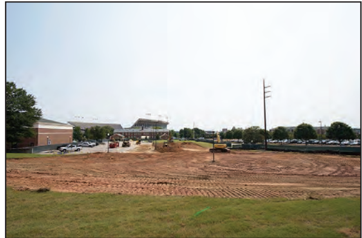
Site work has just begun for the new building.
