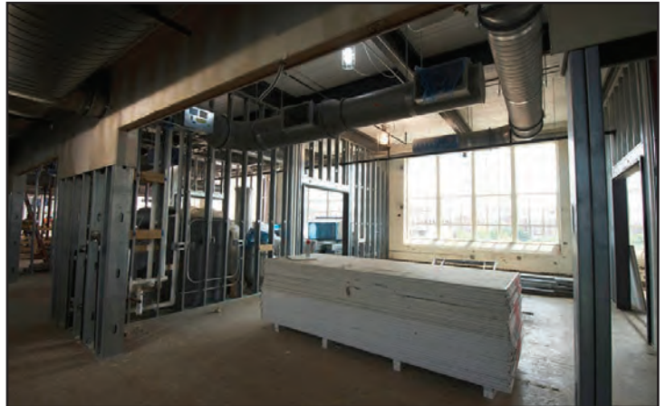
Drywall will soon be installed on the second and third floors.
