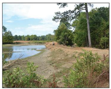
Compactor works to repair the pond dam.
