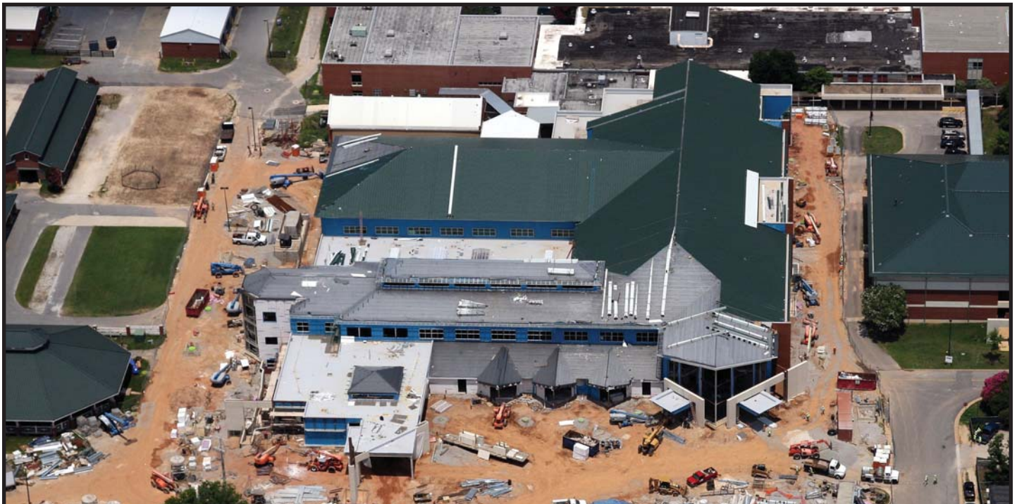
Aerial view of Small Animal Teaching Hospital - Phase II
