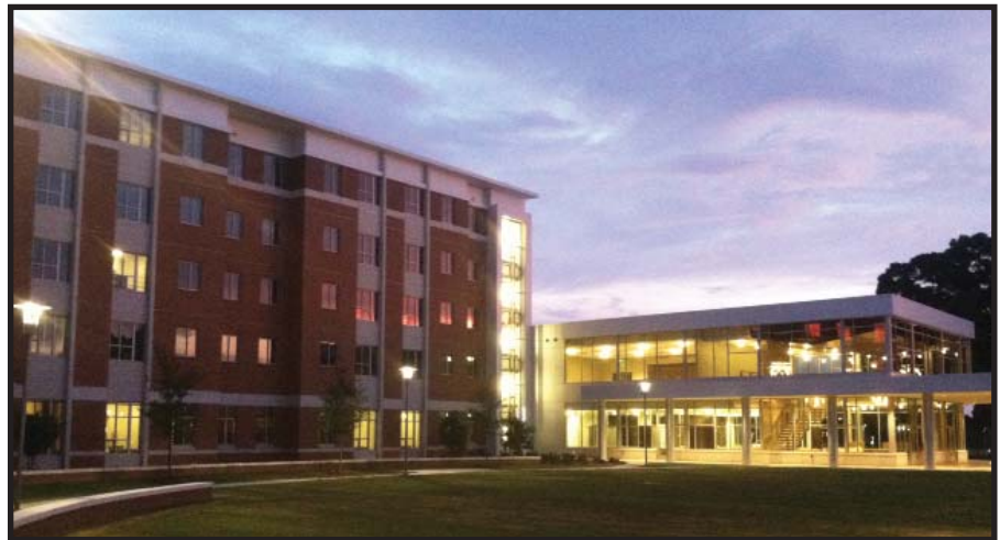
North elevation inside courtyard
