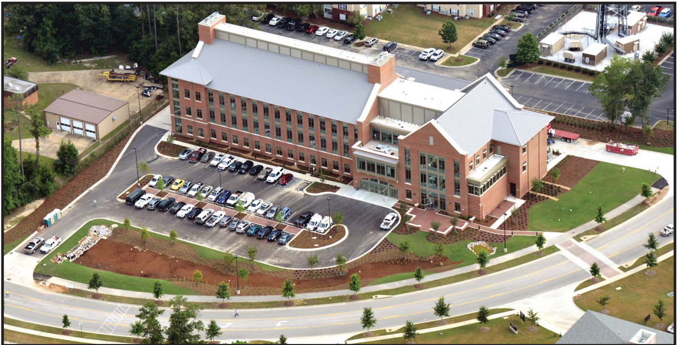
Aerial view of Center for Advanced Science Innovation and Commerce
