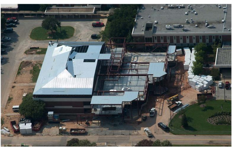
Small Animal Teaching Hospital - Overton-Rudd Classroom Addition Steel Erection and Roof Installation (Note: CVM Main Entrance is on the Far Right of the Picture.)
