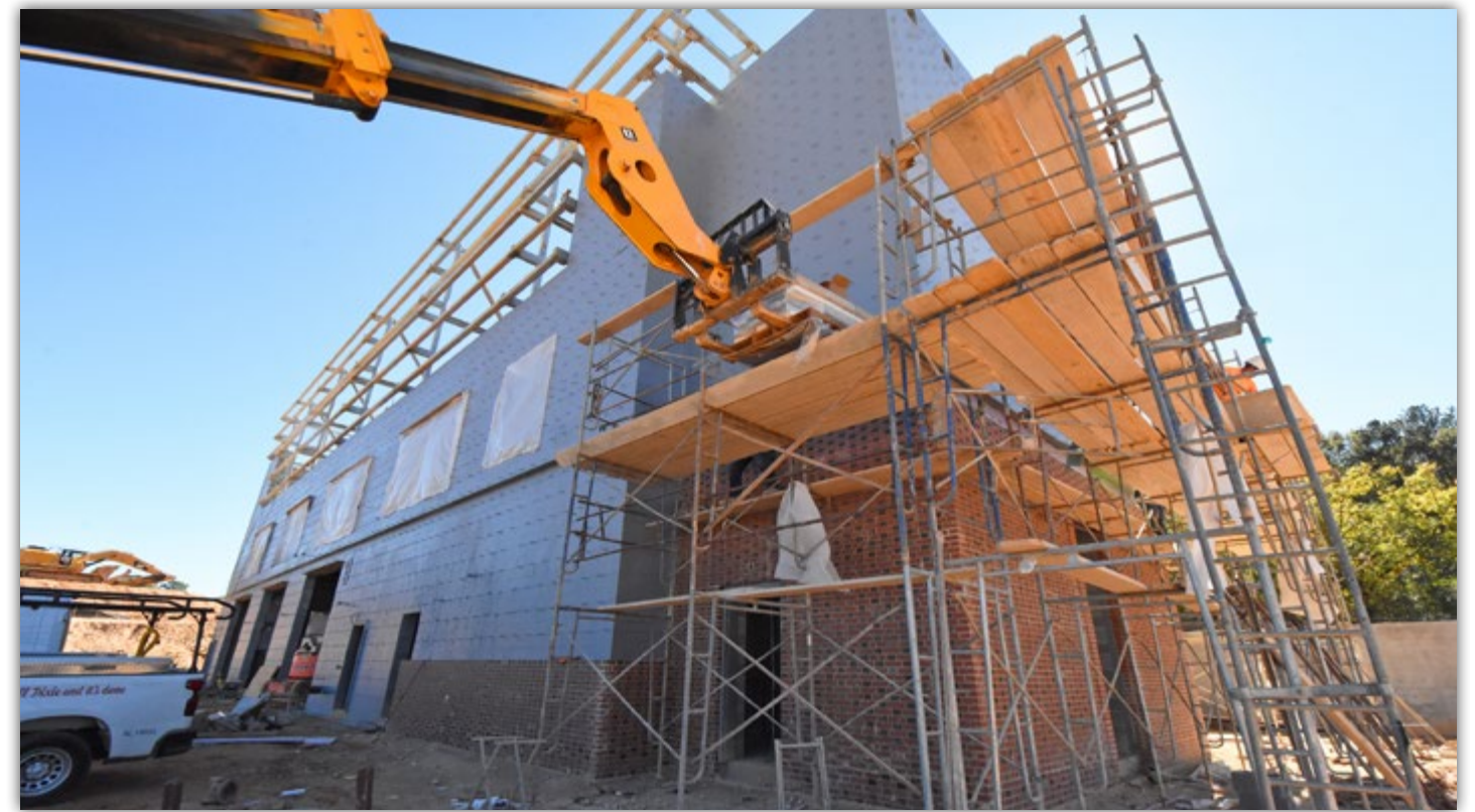
Brick work has begun on the northeast side of the plant.
