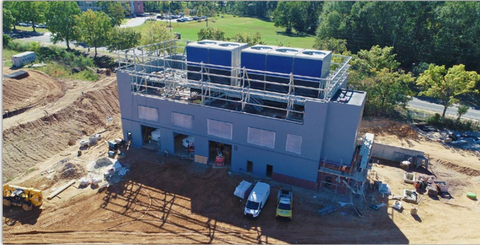
An aerial photo of the Chilled Water Plant structure located on Lem Morrison Drive.
