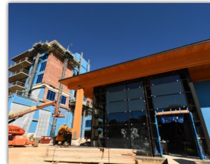
Window installation for the Hey Day Market nears completion.
