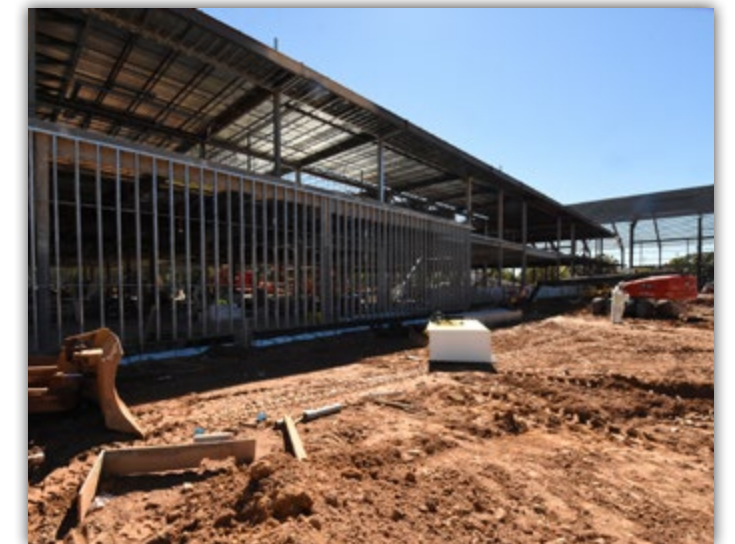
Exterior wall framing continues outside of the locker room.
