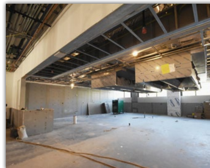
First floor culinary lab duct work is nearing completion.
