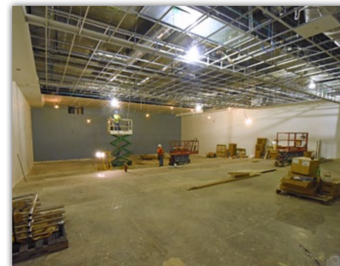
Overhead ceiling installation has begun in the first floor lecture halls.
