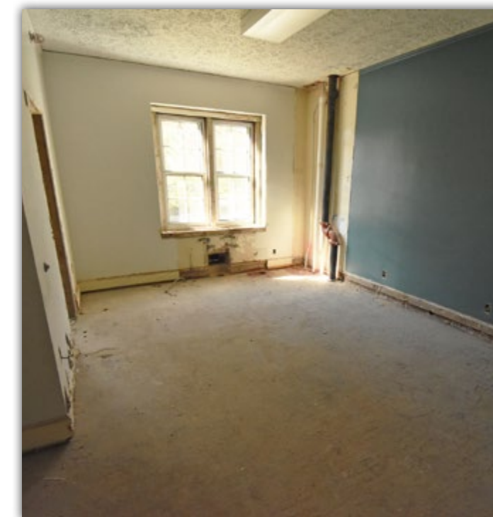
A bedroom inside Broun Hall is almost ready for its facelift.
