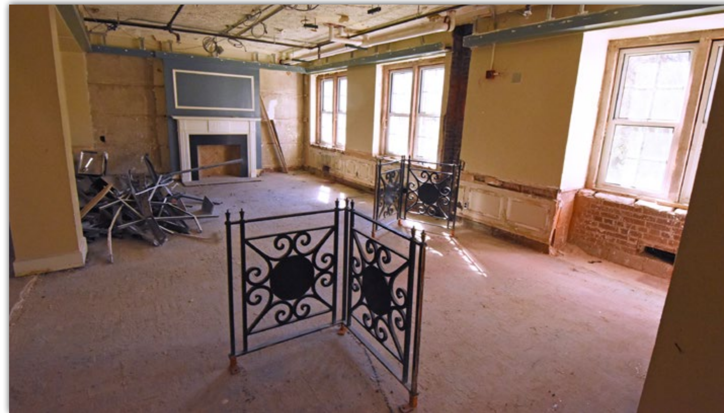
Demolition is well underway for the student area in Broun Hall.
