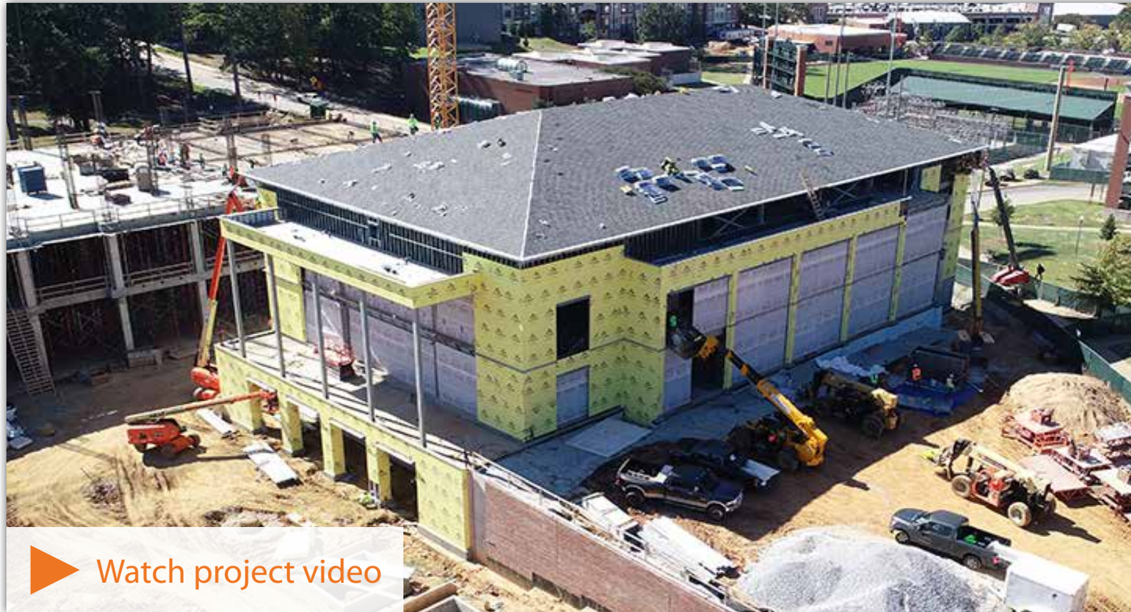
The yellow shown on the exterior of the Central Dining Hall is the completed waterproofing.
