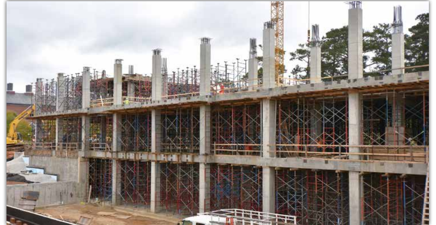
Concrete columns, built to support the third floor, are complete.
