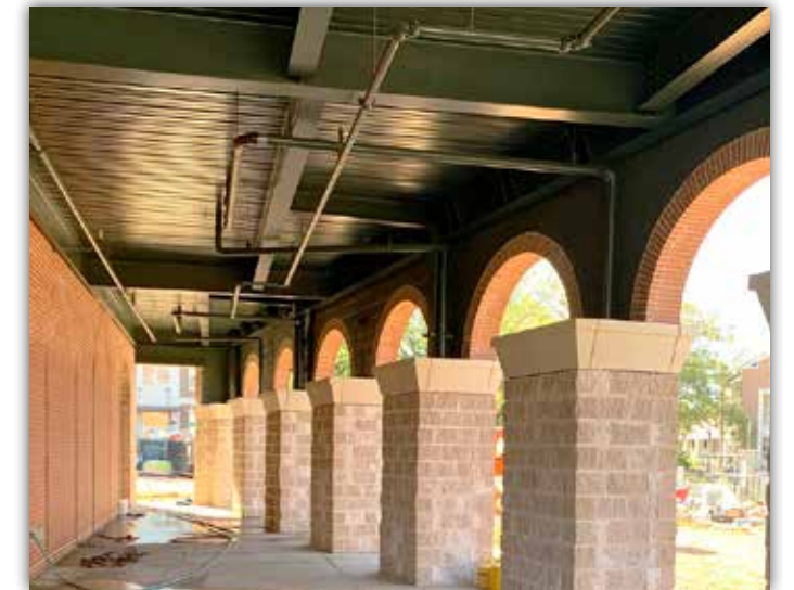
The arched column design, along the front of the building, matches the existing Plainsman Park design.
