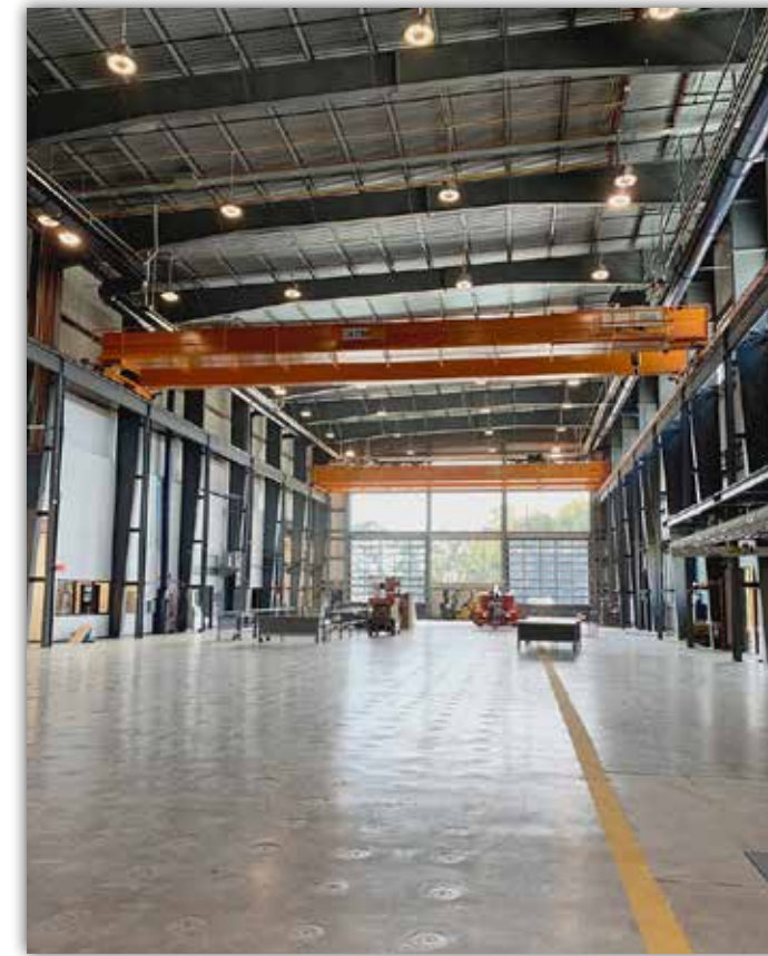
The Civil Engineering Department will soon move equipment into the high bay test laboratory.
