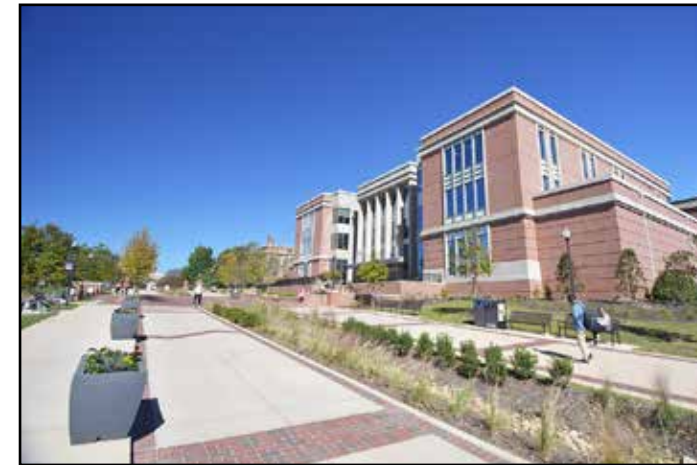
Self-watering planters and an eco swale help make the concourse green and sustainable.
