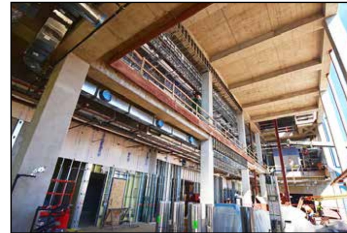
This area will become a glassed atrium facing the Lowder Courtyard.
