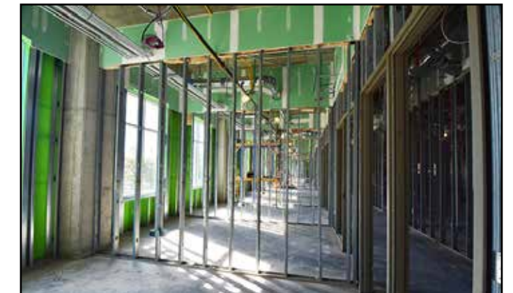
Metal wall framing shapes offices located inside the Brown-Kopel Engineering Student Achievement Center.
