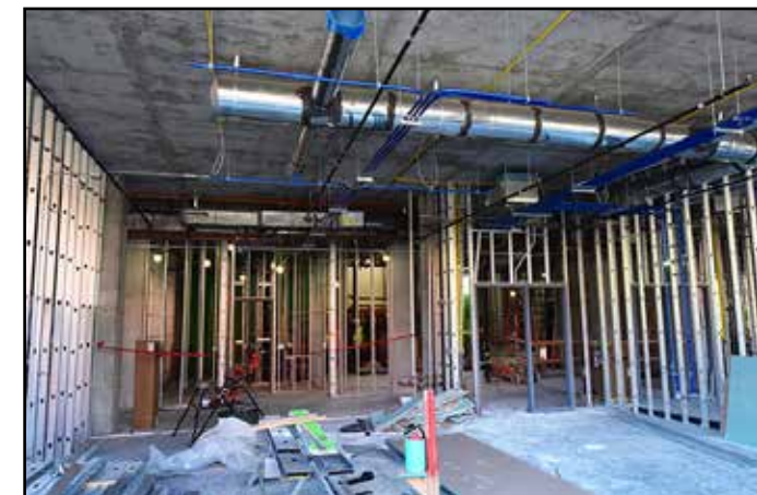
Interior metal wall framing begins to outline offices and classrooms.
