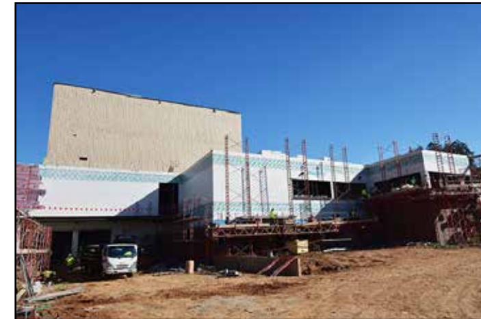
Brick installation continues on the back of the house area.
