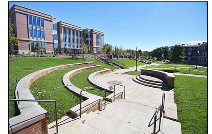
Concrete seating areas outlines the new Theater III outdoor learning space and event venue.
