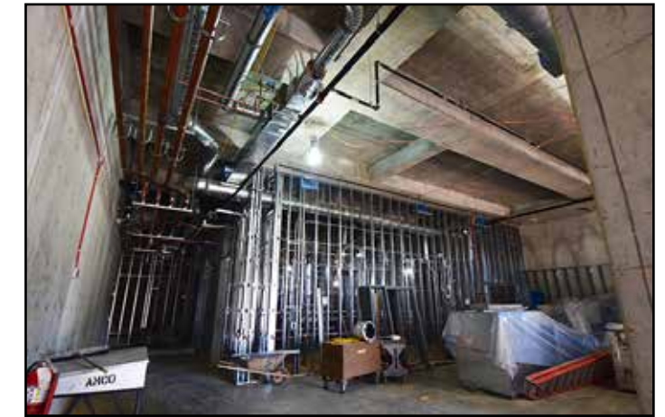
Metal wall framing outlines offices and study space within the building.
