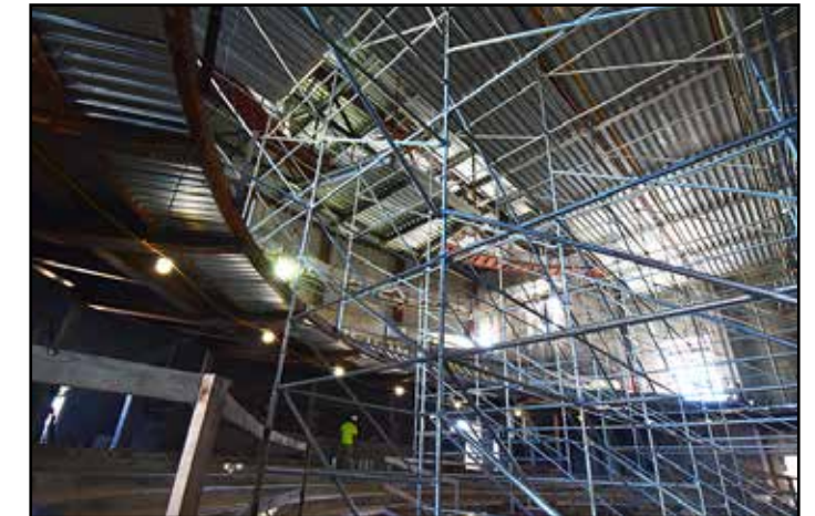
Theater seating support systems are in place.
