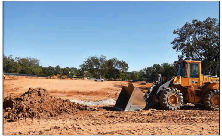
The building pad is beginning to take shape.
