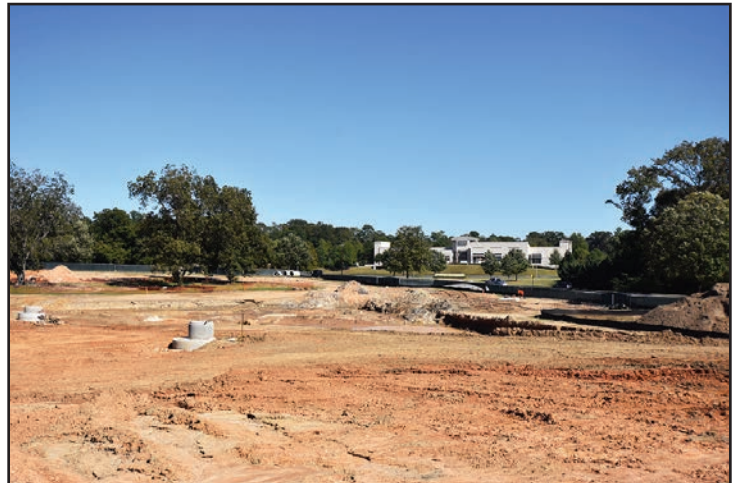
Excavation work for the pond is underway.
