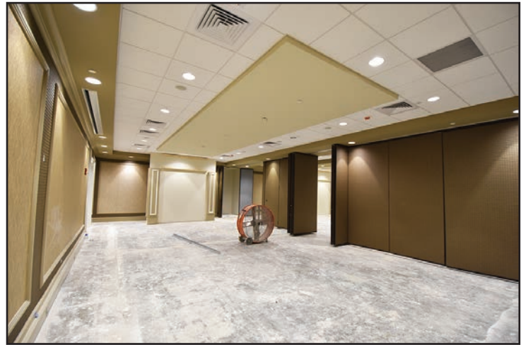
Wall dividers are being installed in one of the ballrooms.
