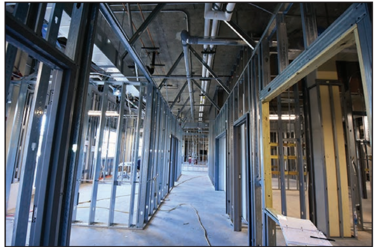
Drywall will soon be installed to frame the office space.
