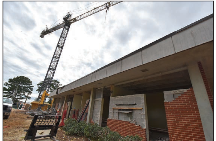
The original section of the building will be demolished.
