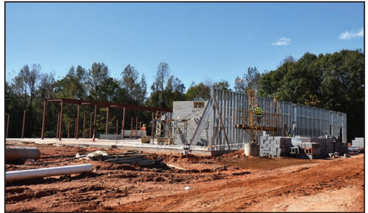
Framing for the Research and Education Center is well underway.
