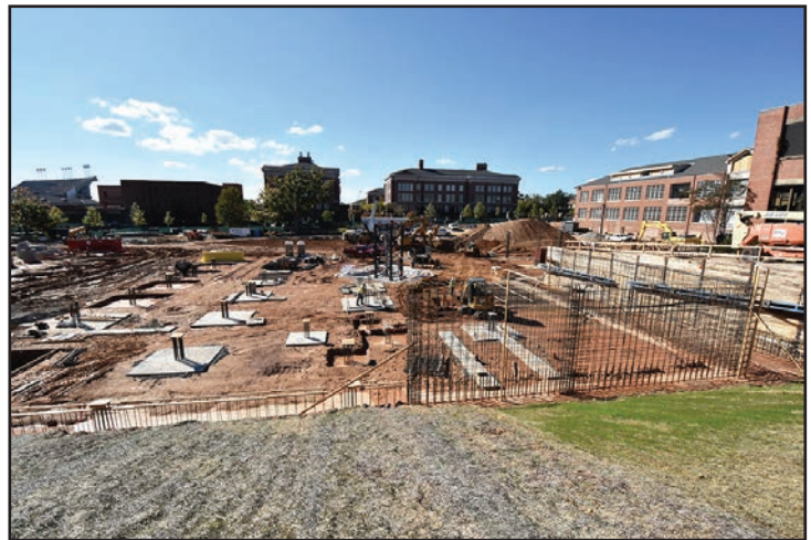
Alternate view of the site looking west toward the Shelby Center.
