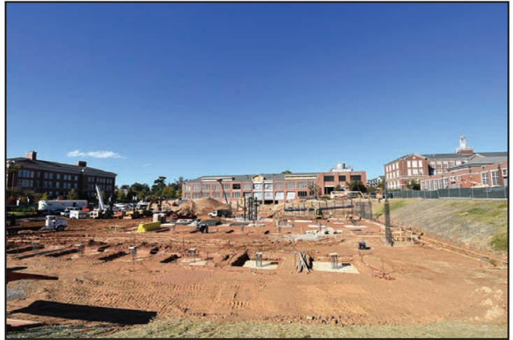
Concrete footing installation has begun.
