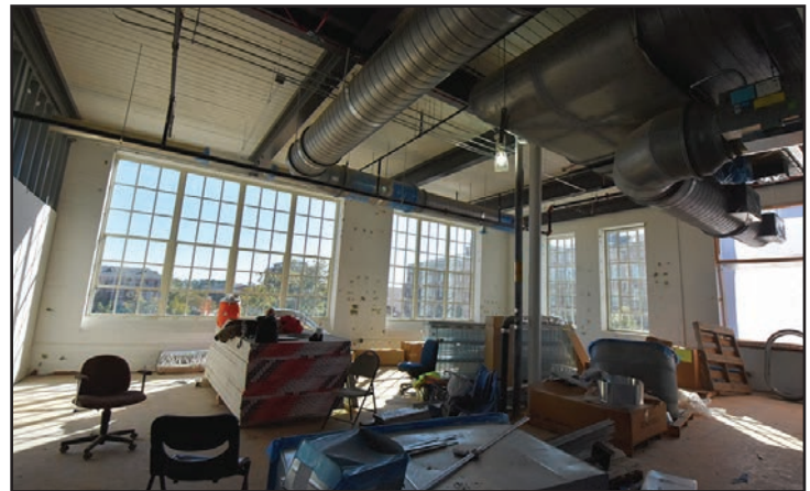
New window installation is 90 percent complete for this project.
