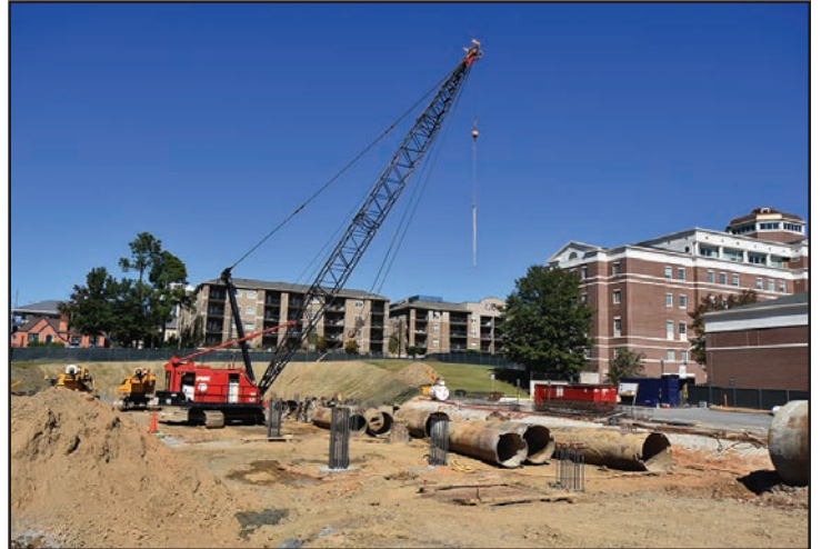
Drilled pier deep foundation work is underway.
