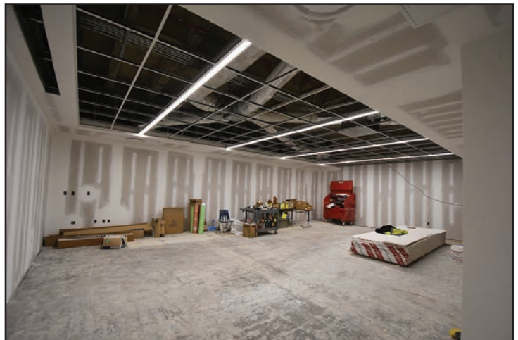
Work continues in one of the new first floor classrooms.
