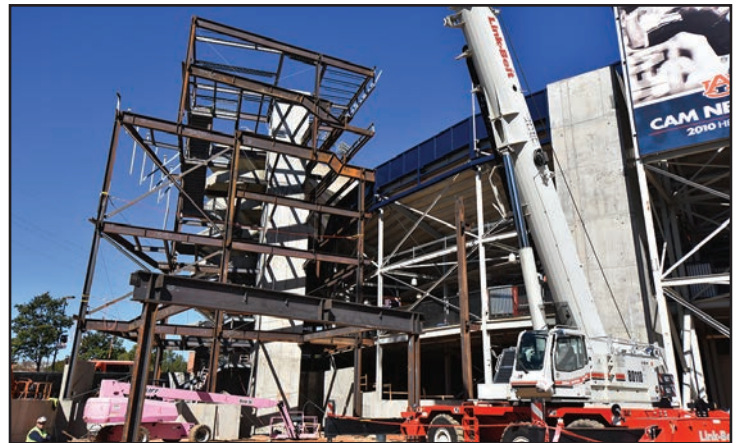
Erection of the facilities' structural steel frame continues.
