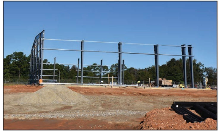
Structural steel framing is being erected for the maintenance hangar.
