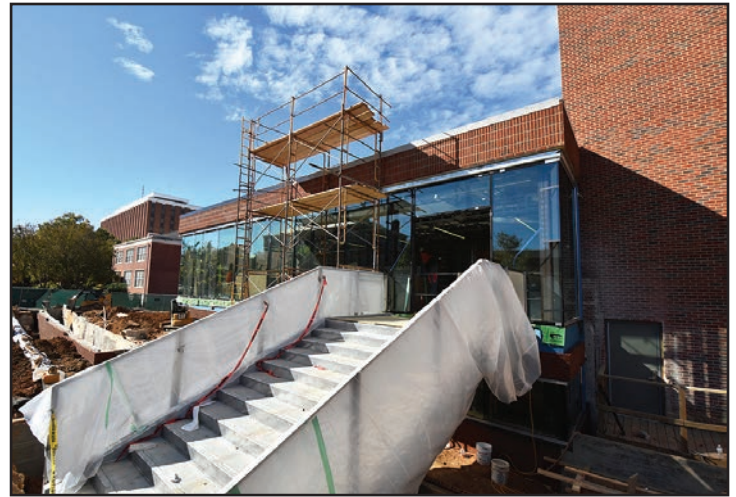
The new entryway and plaza nears completion.
