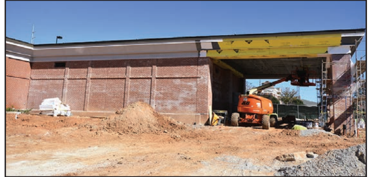
The Emergency Operations Center addition located behind the building.
