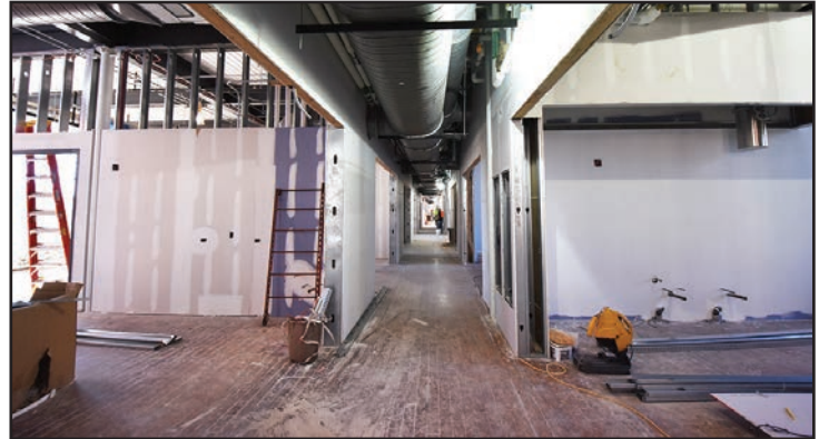
Interior work continues on the second floor.
