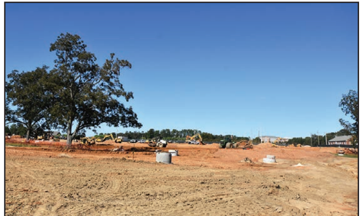
Installation of storm water and sewer infrastructure is underway.
