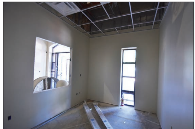
Drywall and ceiling tile installation continues in the receiving area.
