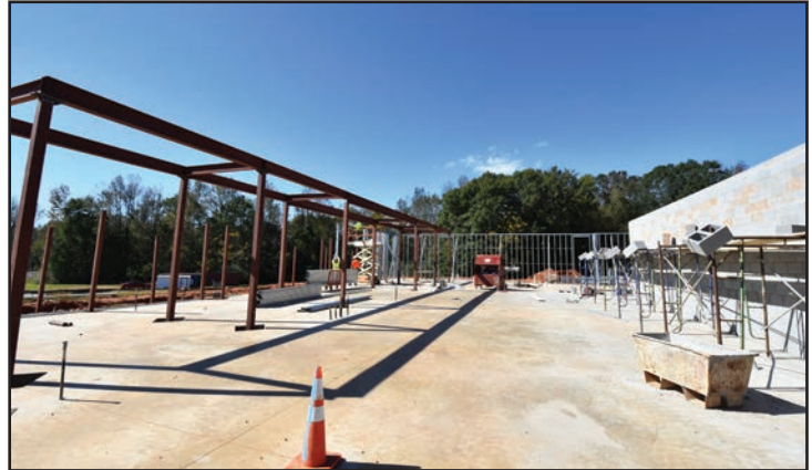
A close-up view of the building's steel and block frame.
