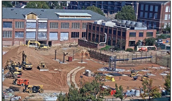
View of the construction site from the Haley Center webcam.
