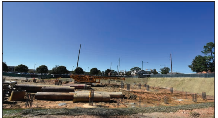
The site currently includes 56 drilled pier deep foundations.
