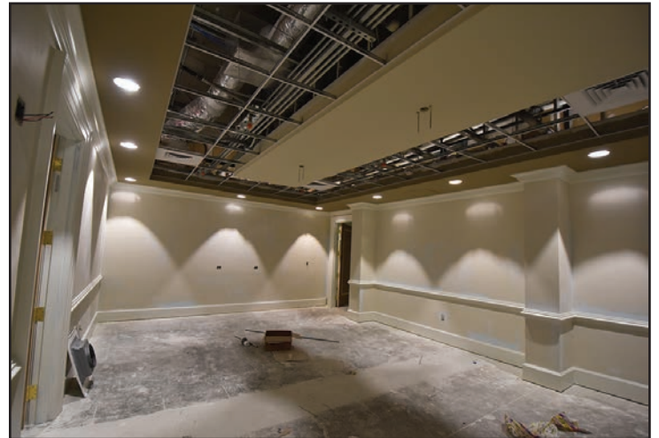
This meeting room is nearing completion.
