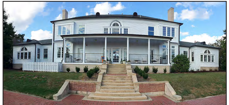
New siding and windows on the Quad side of Cater Hall.
