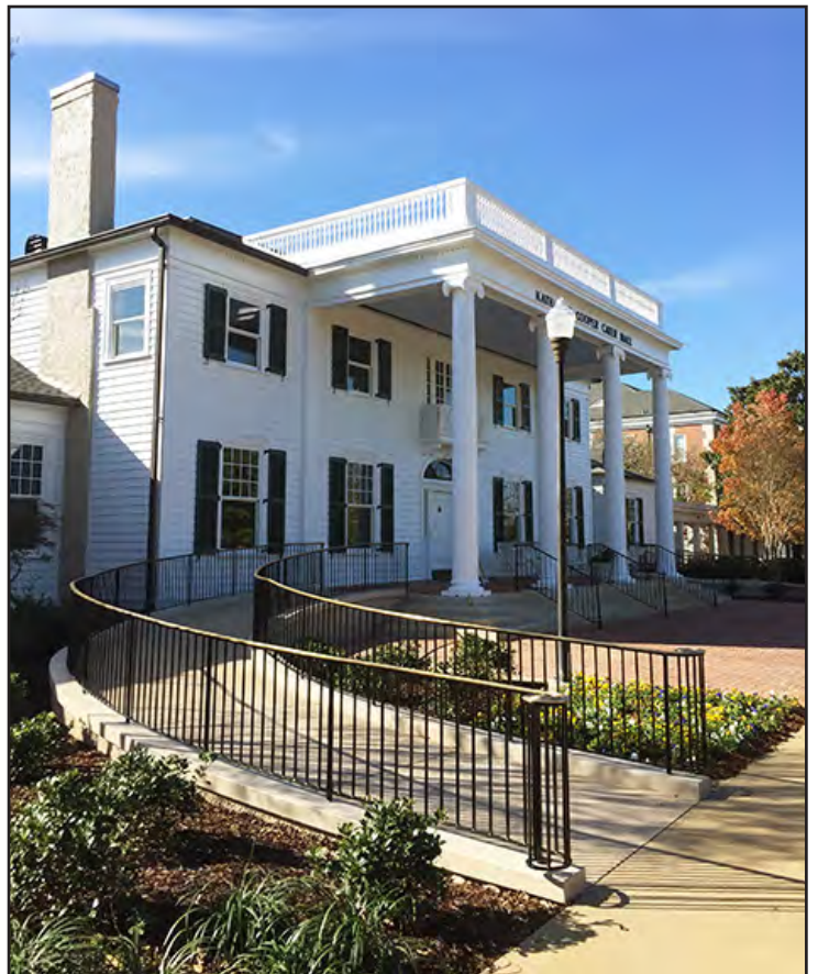
New handrailing and pedestrian ramp in front of Cater Hall.
