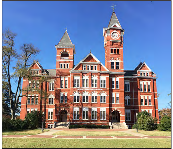
View of the new roof from Samford lawn.
