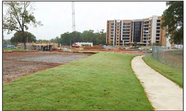
Additional site preparation work continues.
