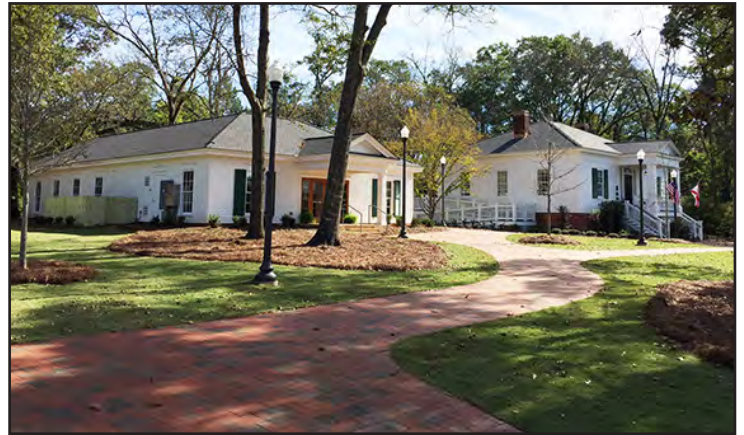
Brick walkways lead to the new building and remodeled house.
