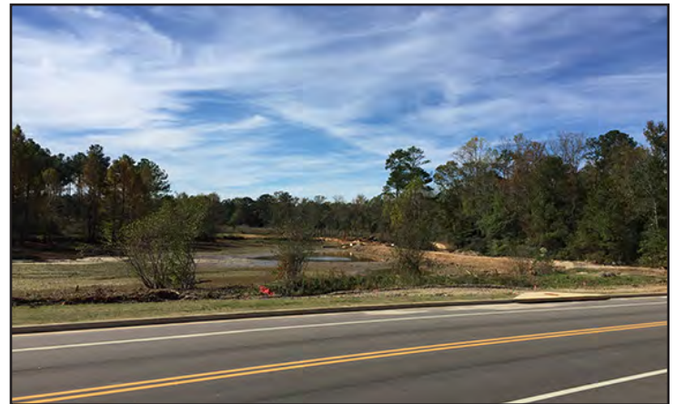
View of construction from Woodfield Drive.
