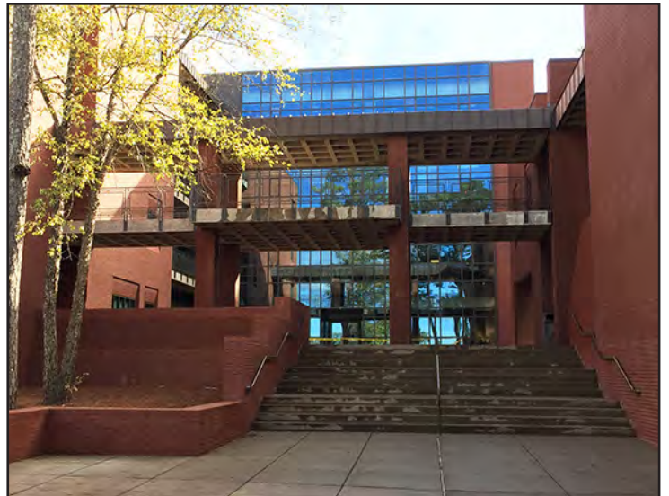
New steps lead up to the courtyard.
