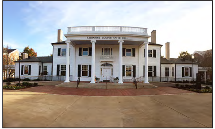
Window and siding installation is complete.
