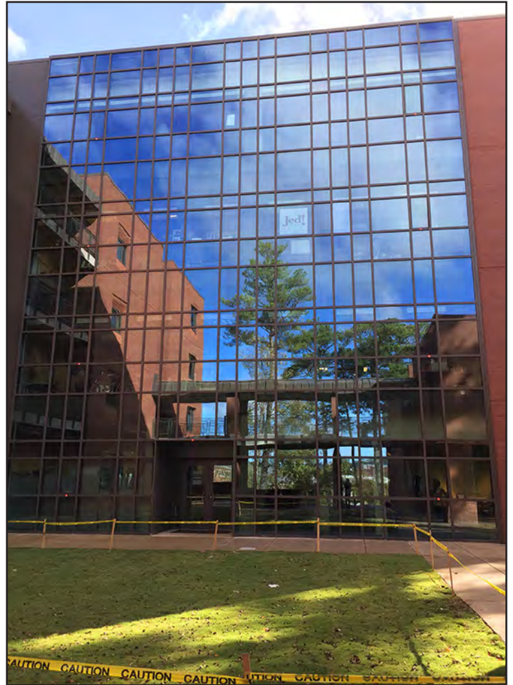
New window wall facing the courtyard.
