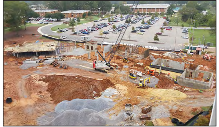
First floor structure is being placed.
