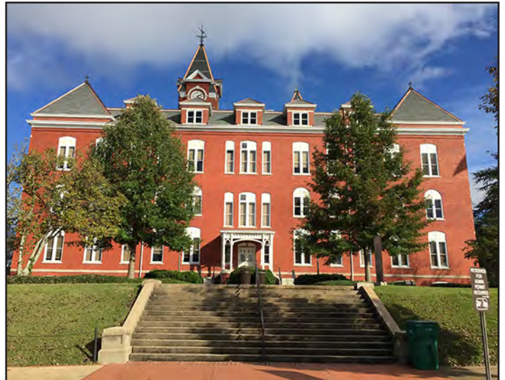
View of the new roof from Ross Square.
