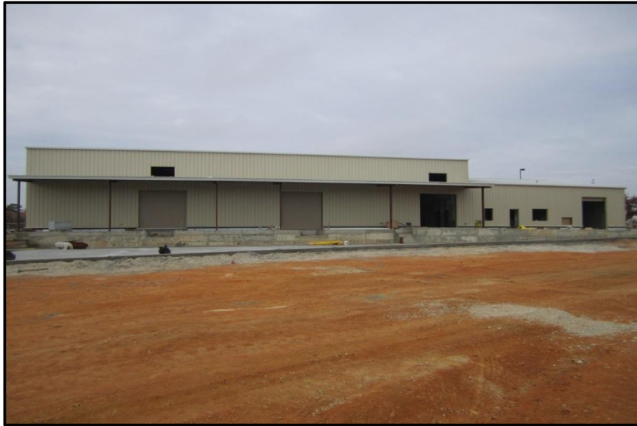
Building 6 Shop Material Warehouse –West View
