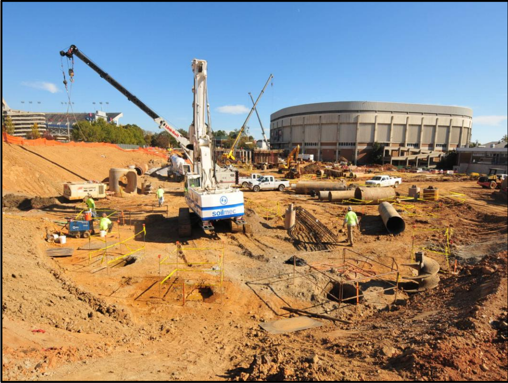
AU Recreation and Wellness Center – Drilled Foundation Pier Holes
