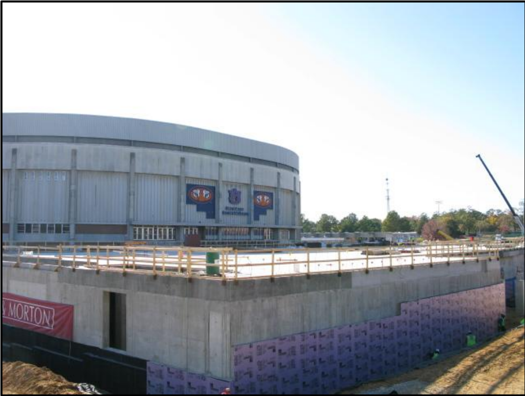
AU Recreation and Wellness Center – Northeast Corner – Elevated Slab
