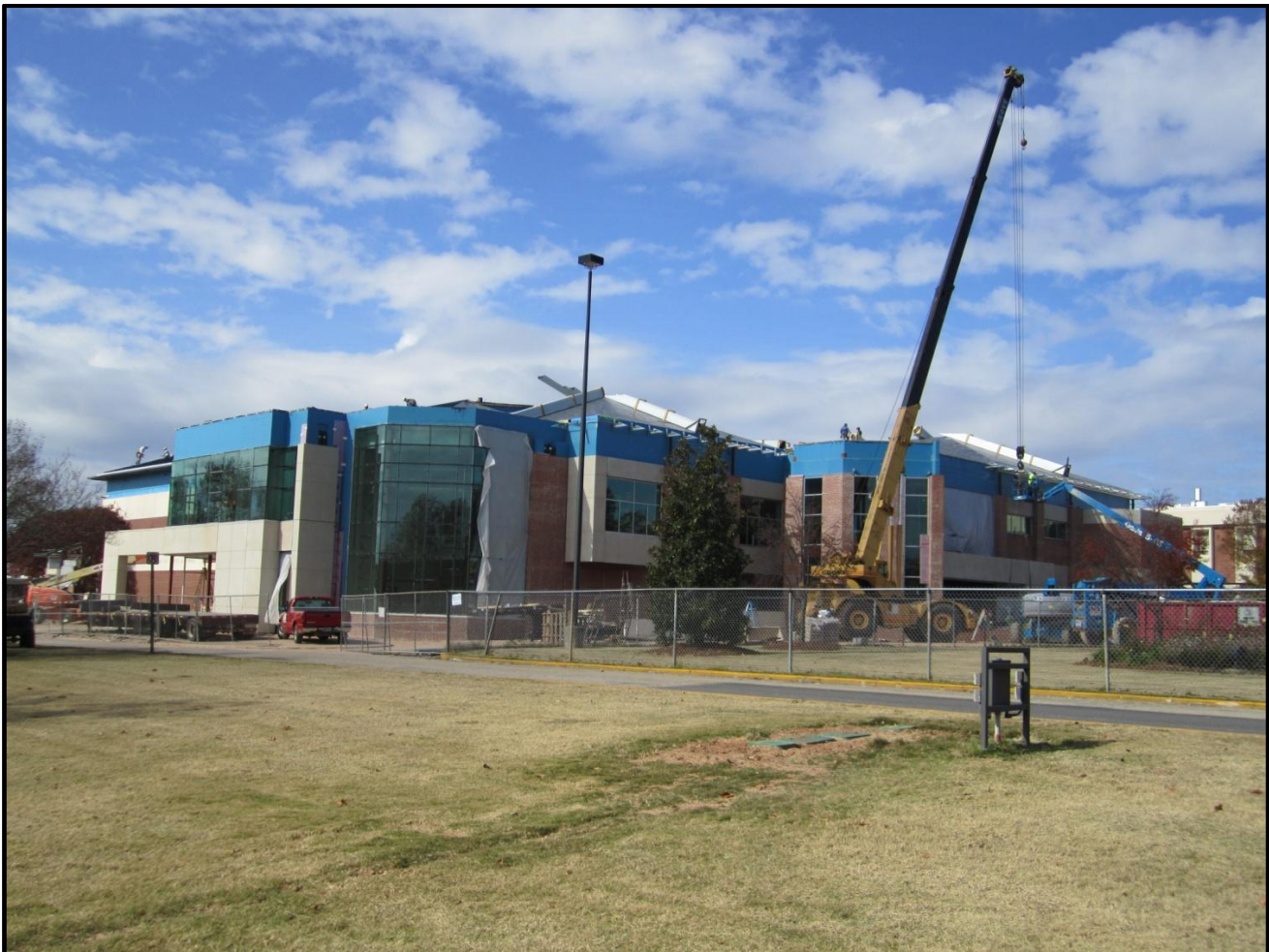
Small Animal Teaching Hospital - Overton-Rudd Classroom Addition (Southeast View)
