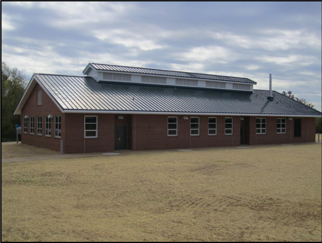
Small Animal Teaching Hospital – Research Lab Building - Northeast View
