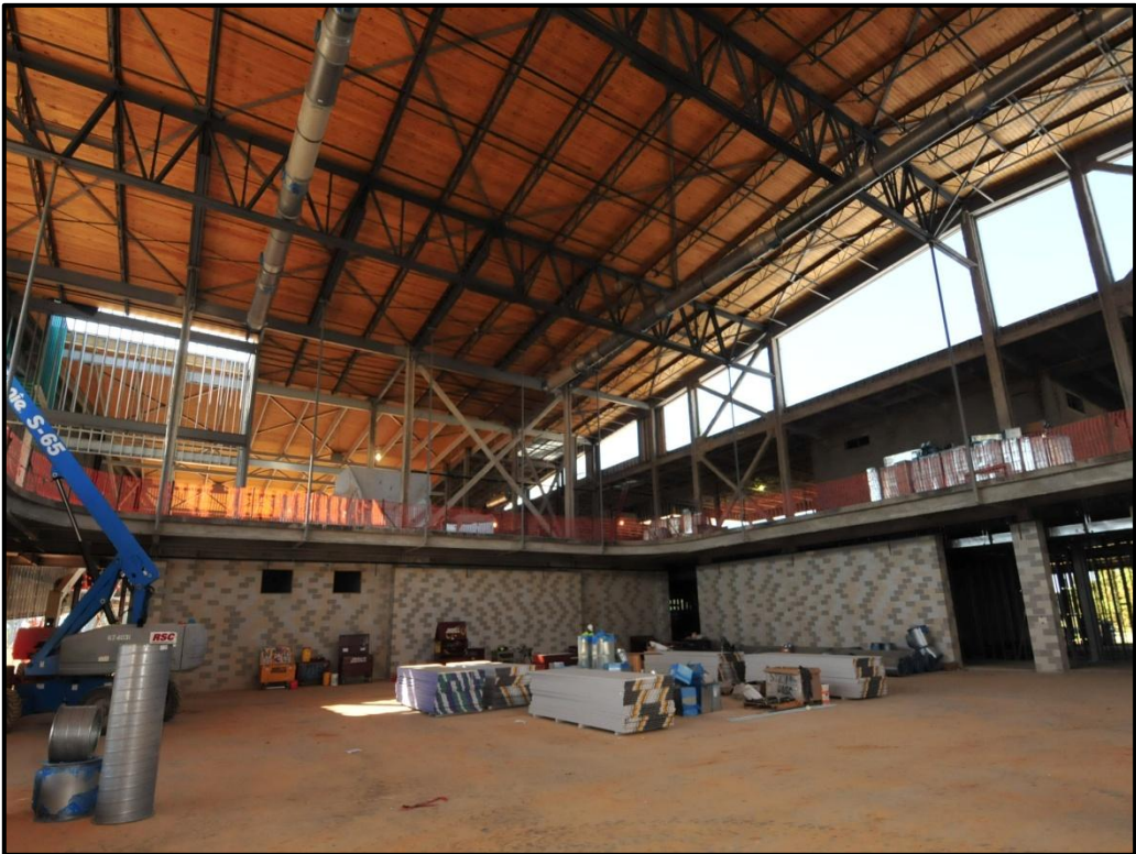
AUM Wellness Center – Courts Area and Elevated Running Track Around Perimeter
