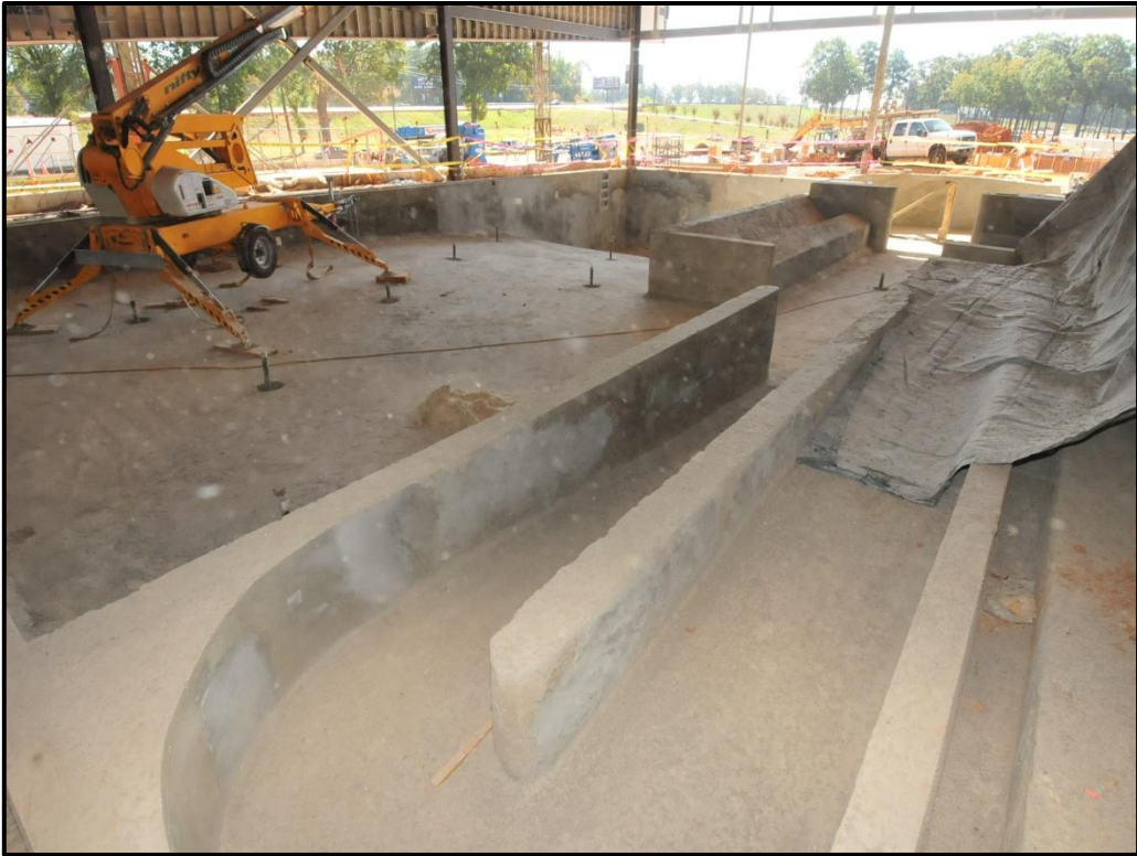
AUM Wellness Center - Interior Pool Construction
