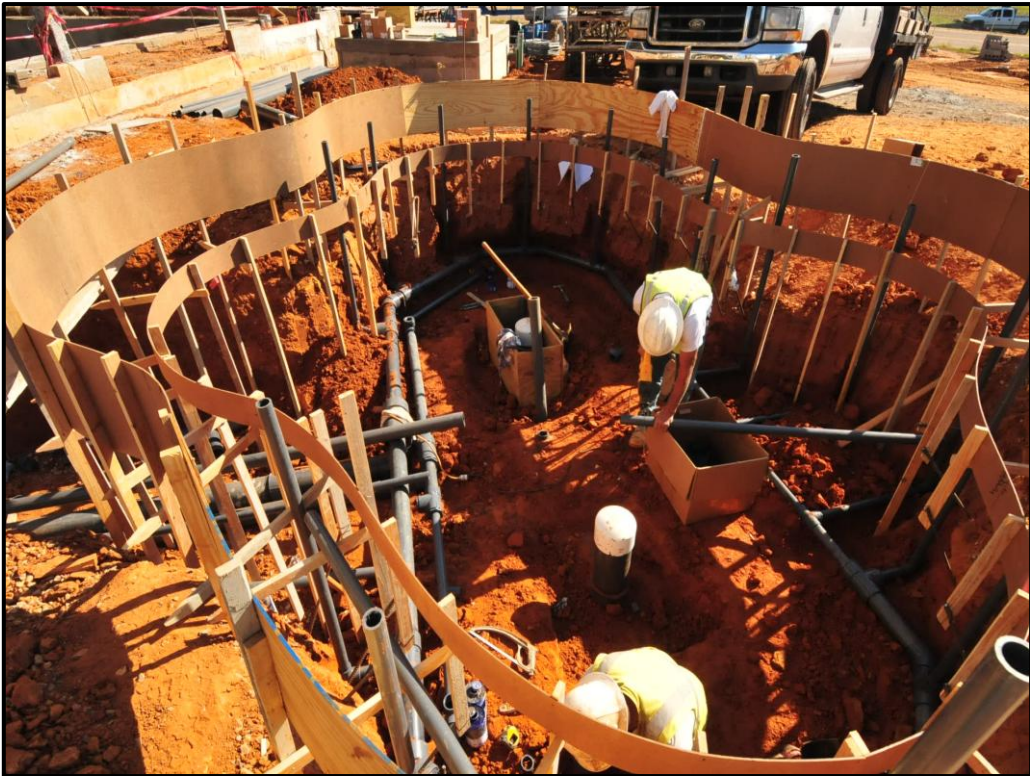
AUM Wellness Center - Exterior Spa Construction
