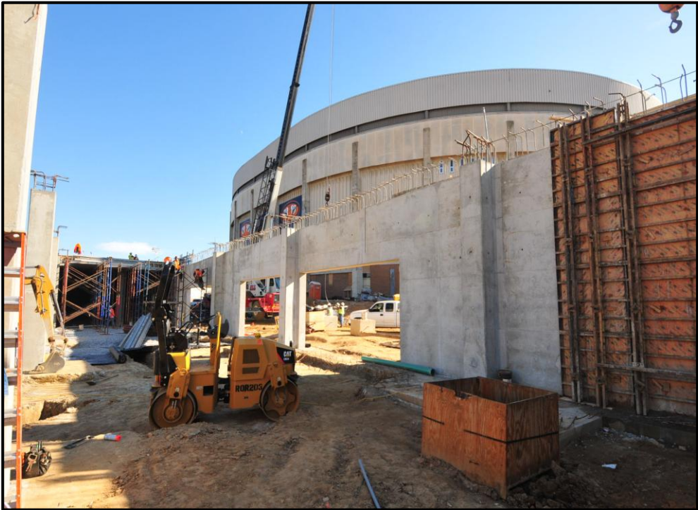
AU Recreation and Wellness Center – Interior View of Foundation Walls
