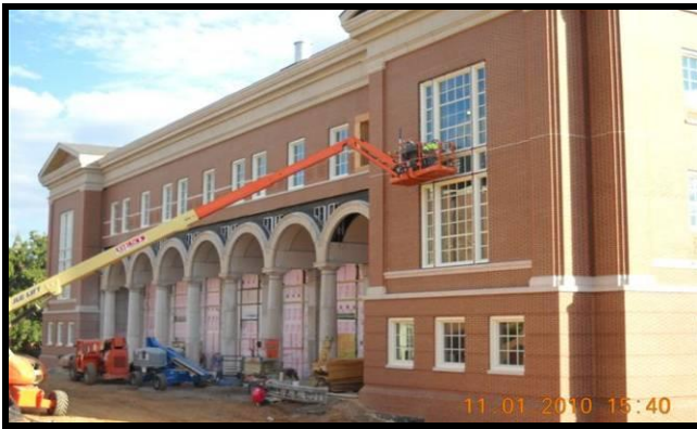
Northwest Elevation of Building F
