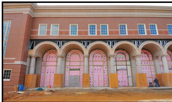
North Face of Building F
