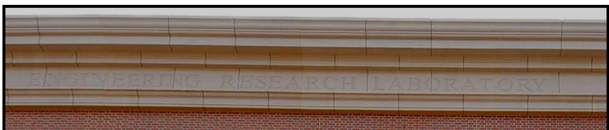
Exterior Building Cornice
