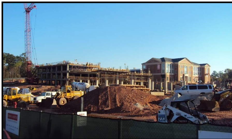
View from Lem Morrison of the South Quad Multimodal Transportation Facility
