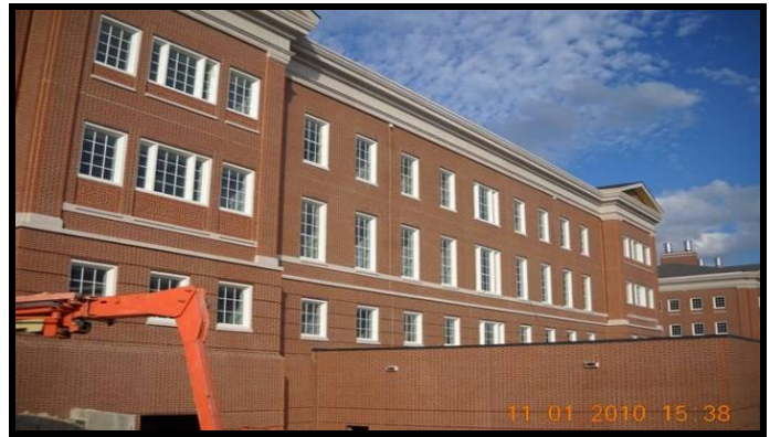
Southwest Corner of Building G
