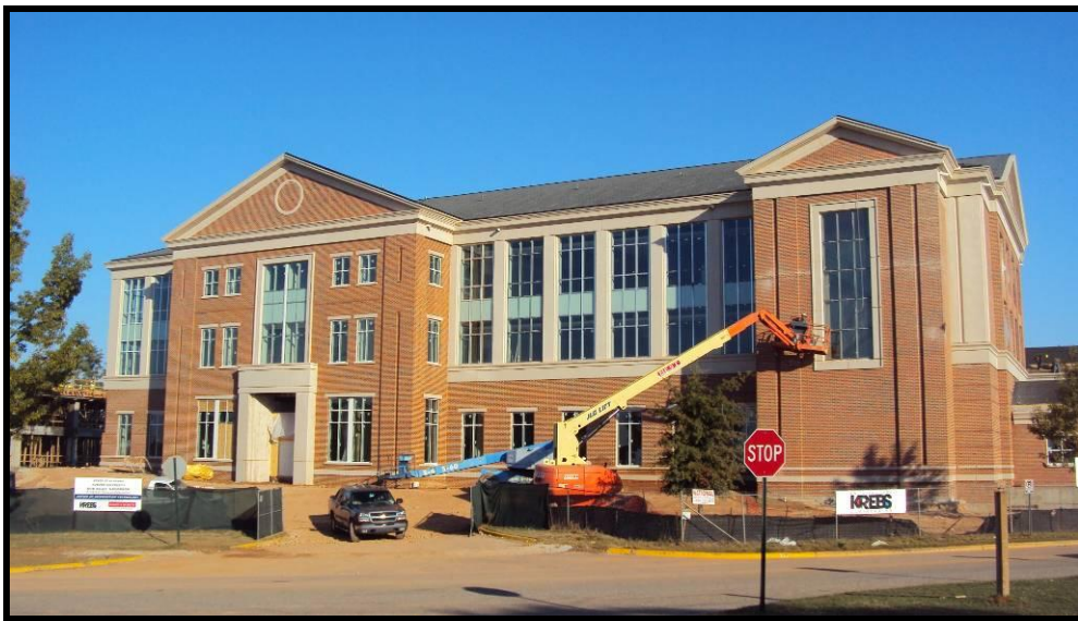
Front of Building
