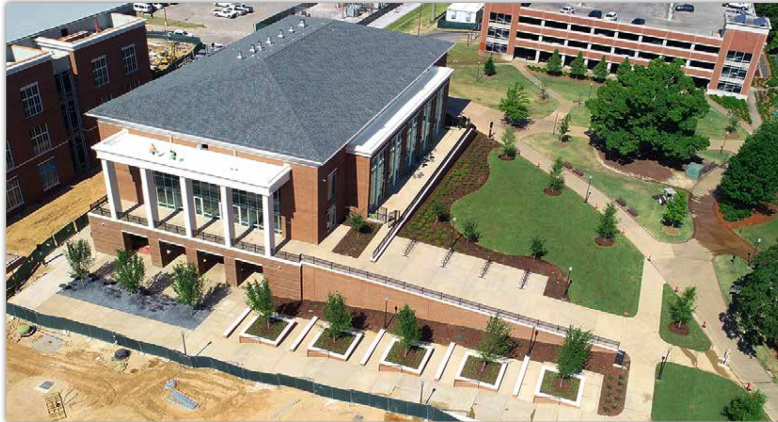
The Central Dining Hall exterior structure and landscaping is complete.
