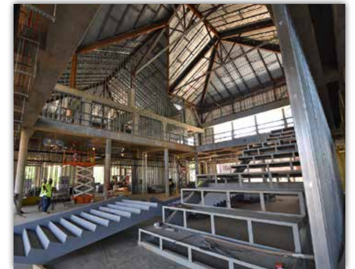
Framing for the atrium is coming together.
