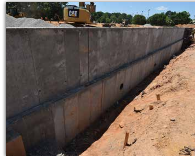
Foundation walls for the hydrotherapy pools have been poured in place.
