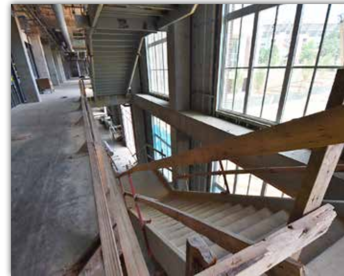
Installation of the stairs leading to each floor continues.
