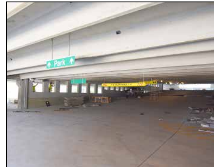
Interior directional signs have been installed.
