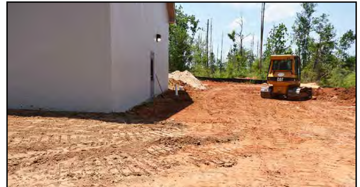
This section is being prepared for parking area gravel.
