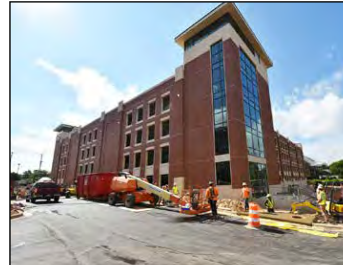
Final asphalt paving is taking place.
