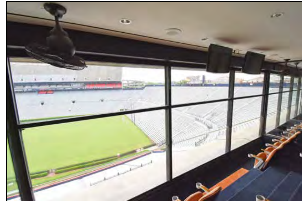
A view of completed work on the third level.
