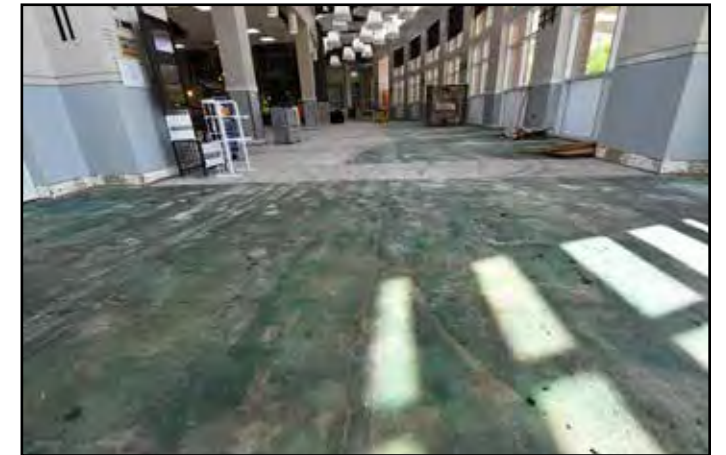
Demolition is complete in the dining area.
