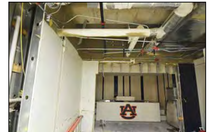
The hydrotherapy and treatment room renovation is well underway.
