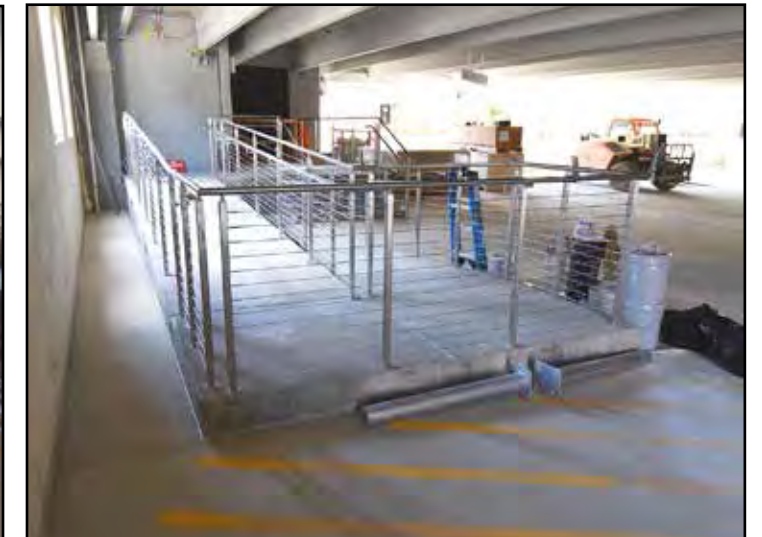
Accessible ramps inside the parking deck are complete.
