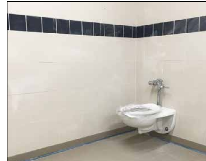
Wall tile and flooring in the new restrooms is complete.
