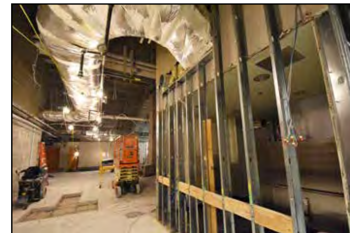
Wall framing is going up for the new team meeting room.
