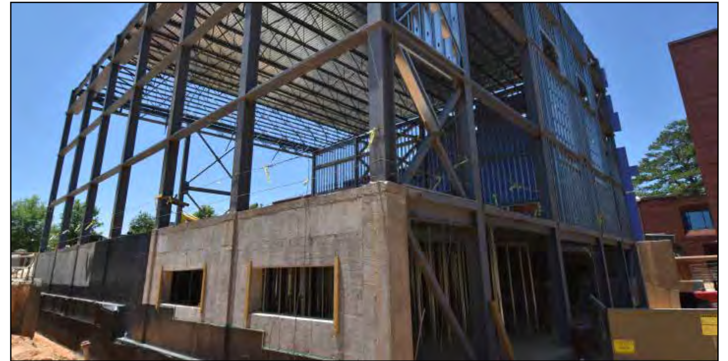
The concrete walls frame out the basement area.
