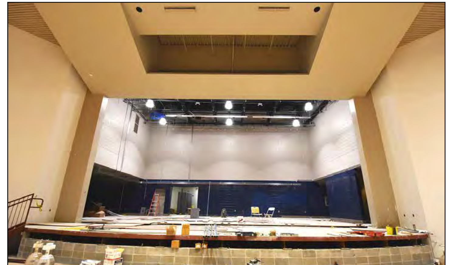
Drywall and painting around the new auditorium stage are well underway.
