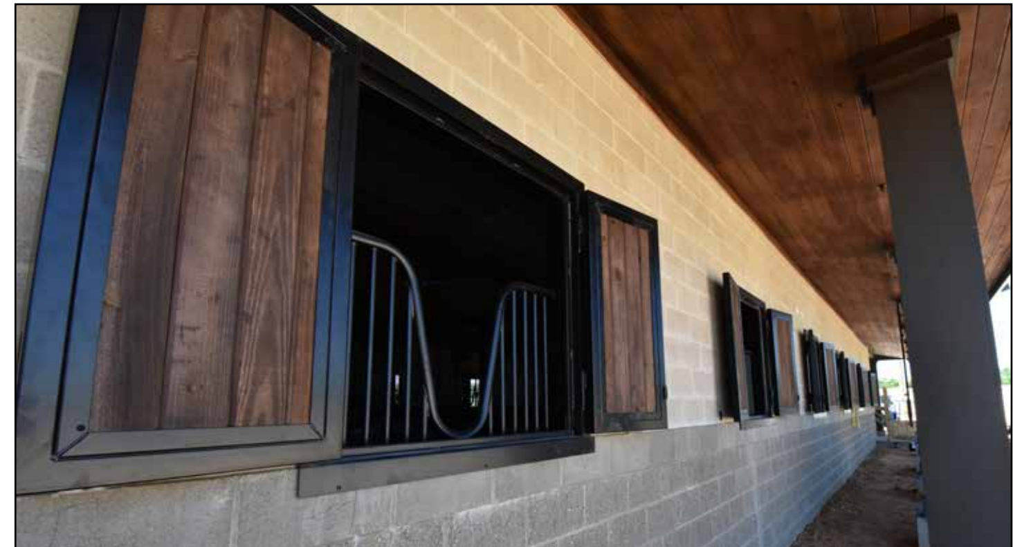
Exterior finish work on the barn nears completion.
