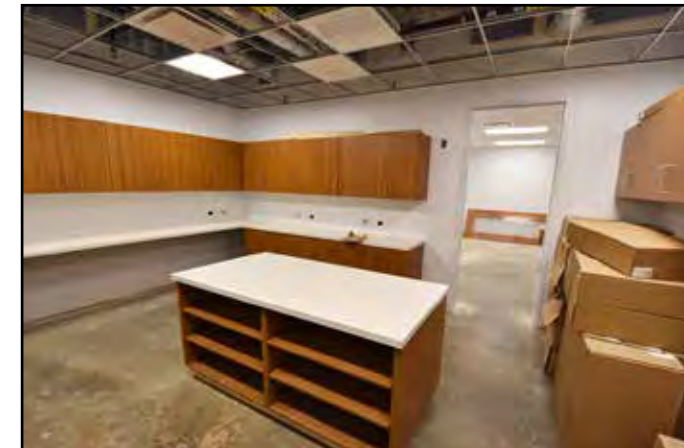
Cabinetry is being installed in an administrative area.
