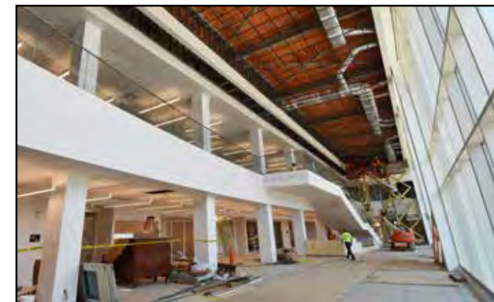
Interior finishes are being installed in the atrium.
