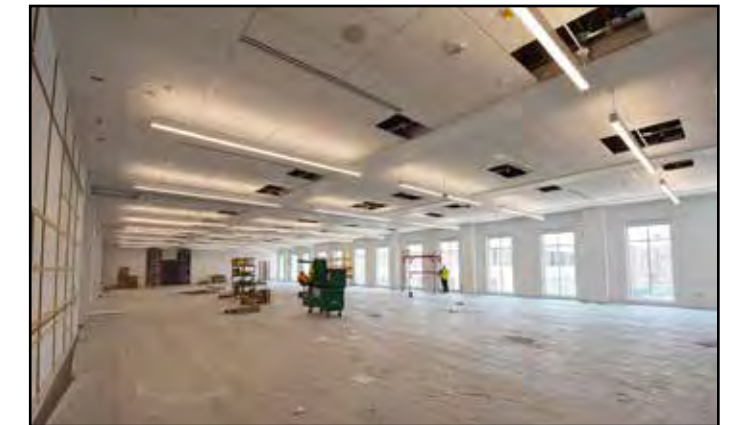
A large classroom located on the second floor.
