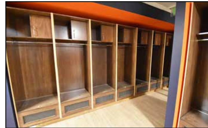
Lockers are being installed in the team support building locker room.
