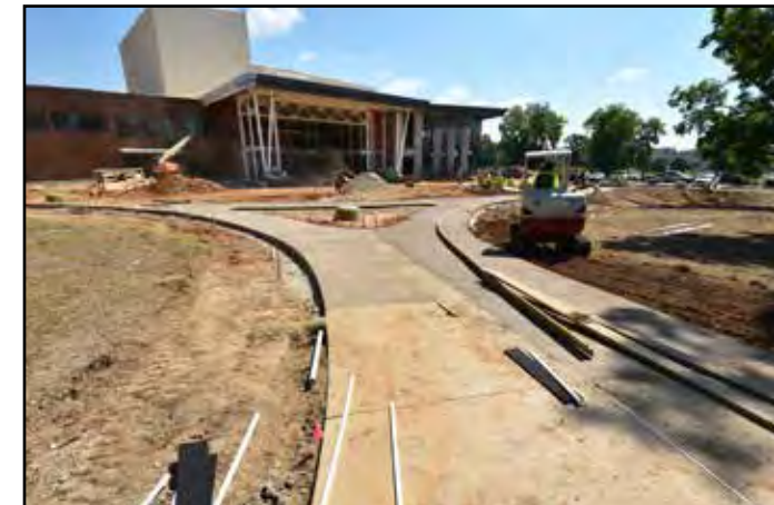
Sidewalk installation is underway leading to the outdoor event space.
