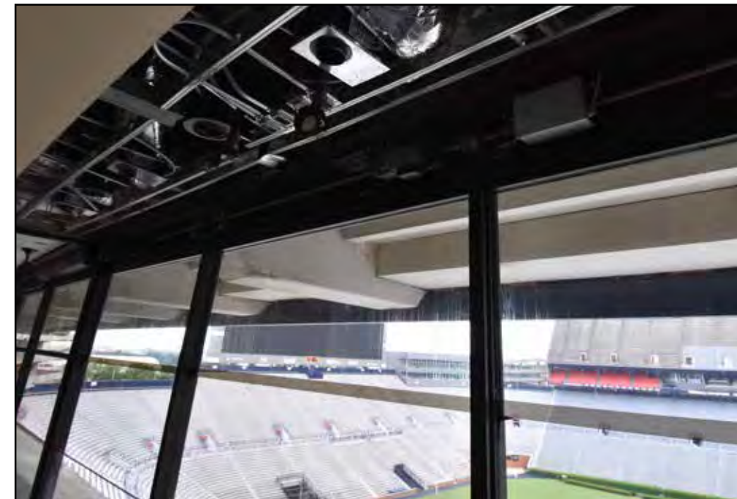
Overhead ceiling work continues on the fourth level.
