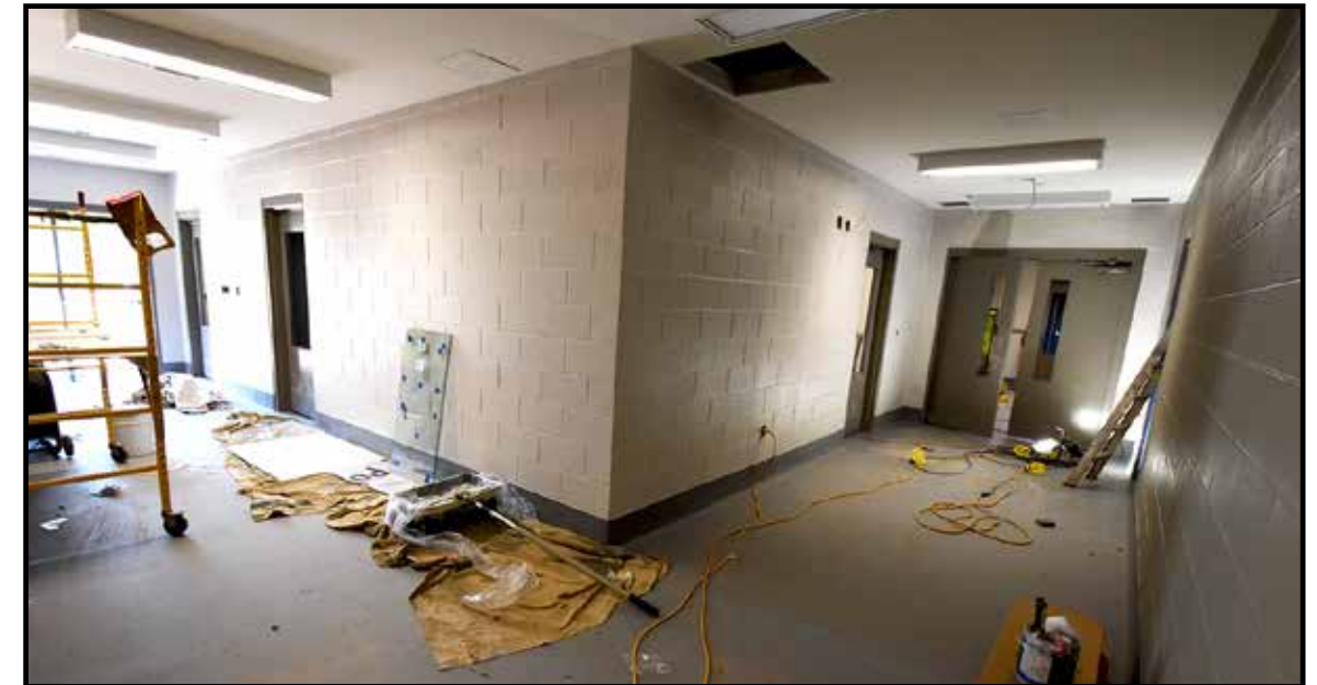
Painting is complete on the interior block walls.
