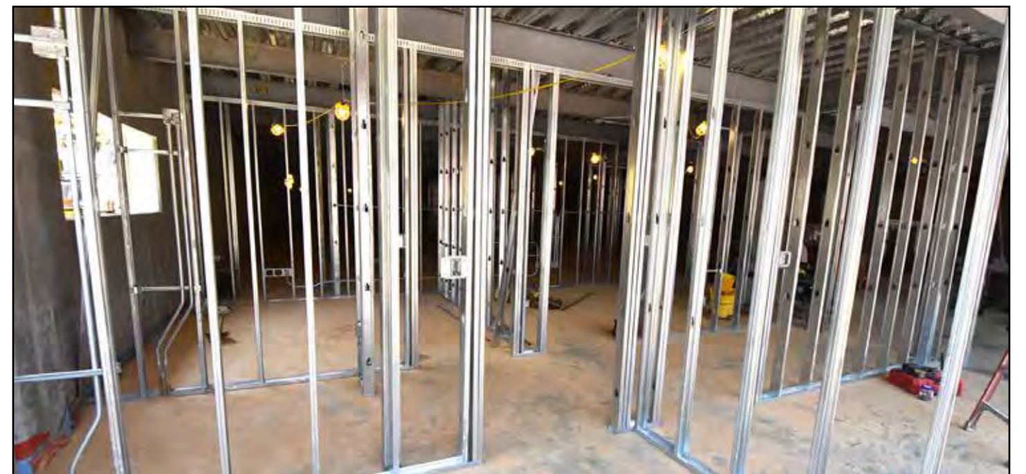
Metal wall framing has begun in the basement.
