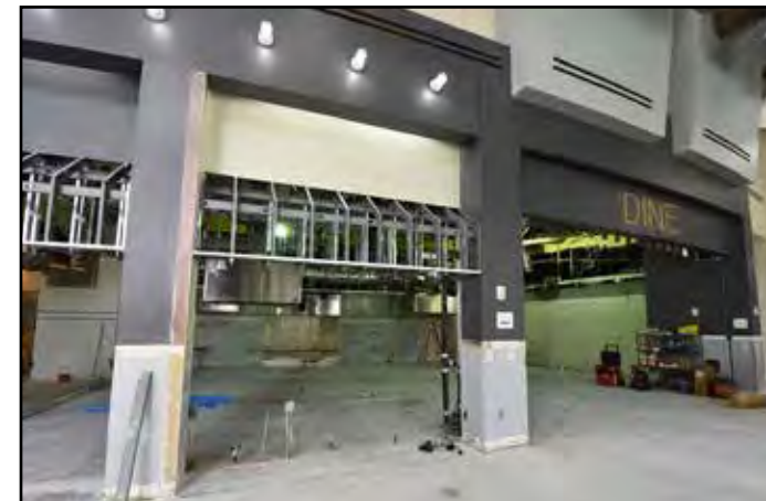
Demolition is underway on the current store front.
