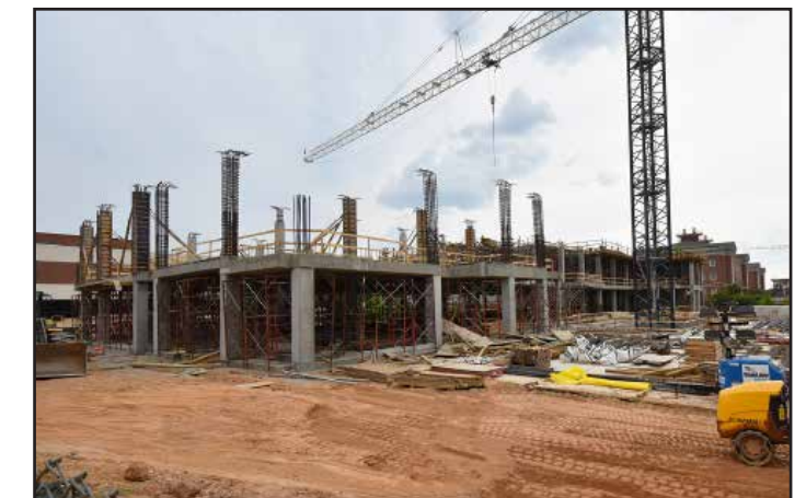
A view of the construction from the east.
