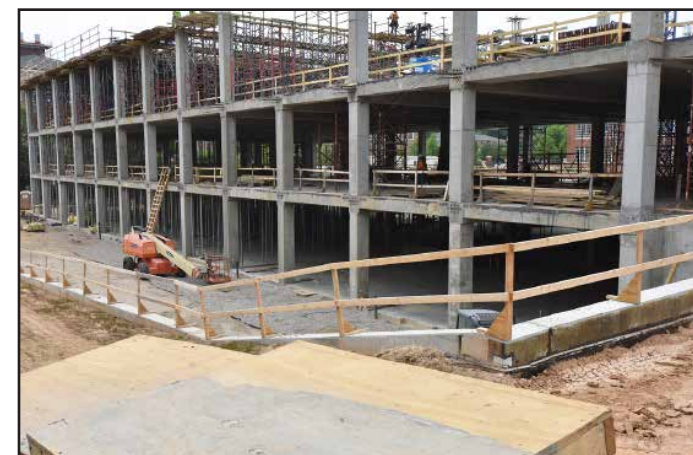
A side view of the first- and second-floor concrete structure.
