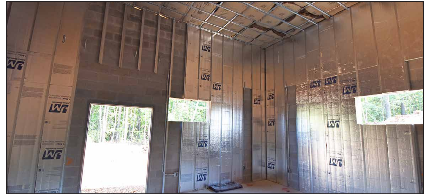
Side rooms have been lined with insulation in preparation for drywall.
