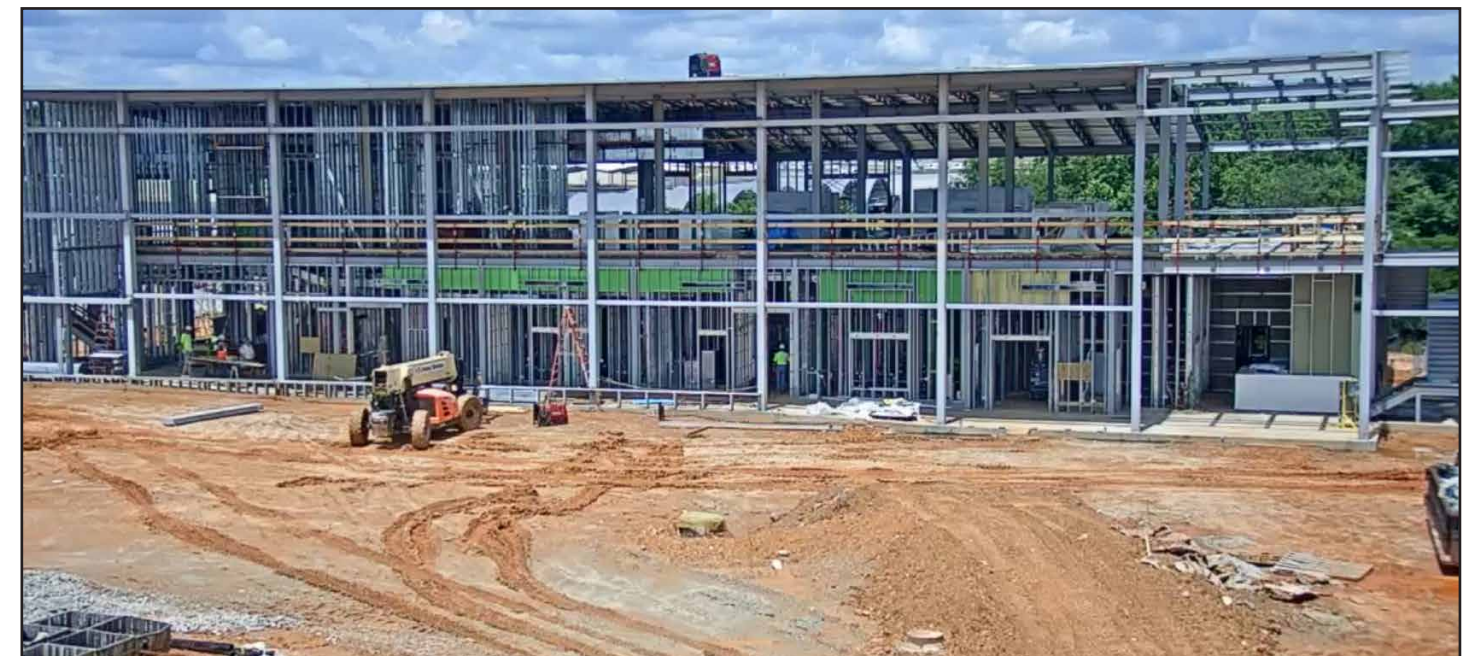
Interior metal wall frames now accompany the outer structural steel.
