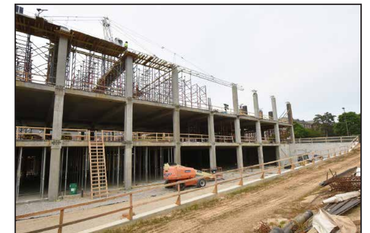
Work on the building's structural frame continues.
