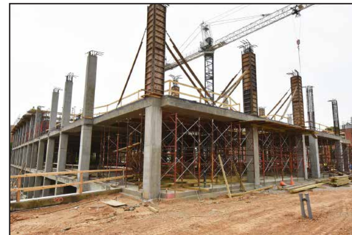
Concrete column construction is underway.
