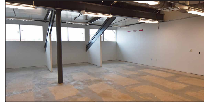
New attic office space is nearing completion.
