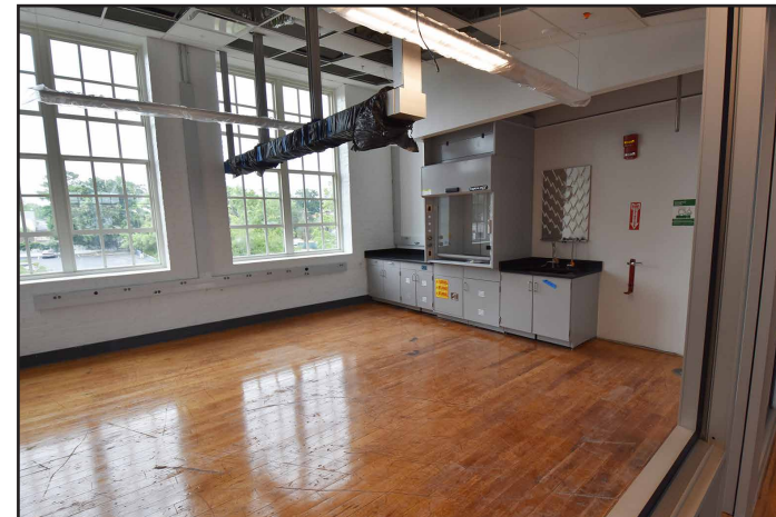
Wood flooring has been refinished throughout the laboratory.
