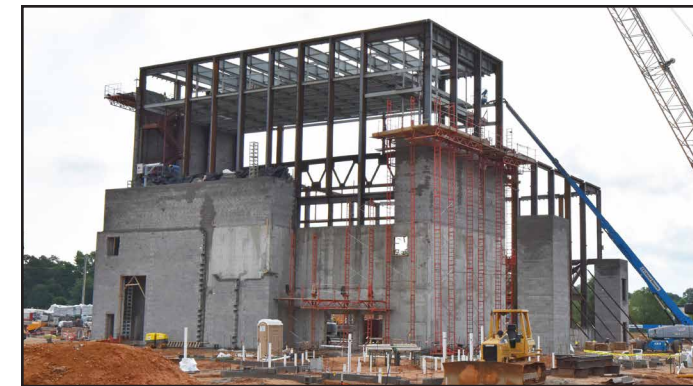
Structural steel is being placed for the auditorium.
