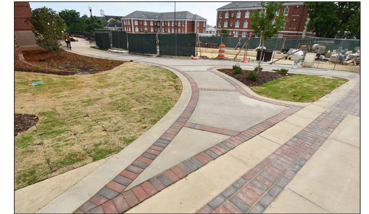
Some sidewalk areas have been completed on the Mell Corridor.
