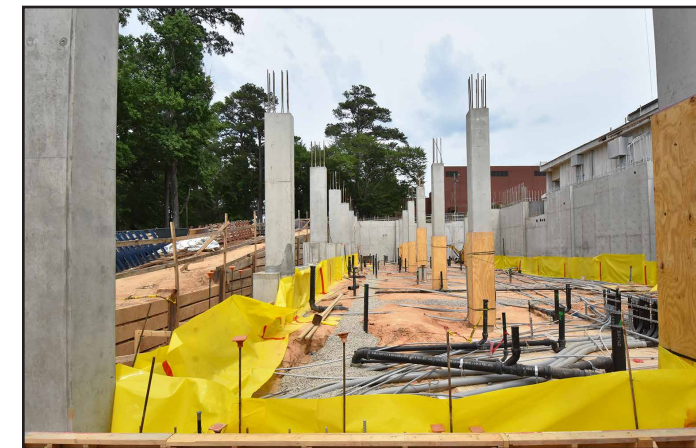
Concrete columns along the east side of the new addition.
