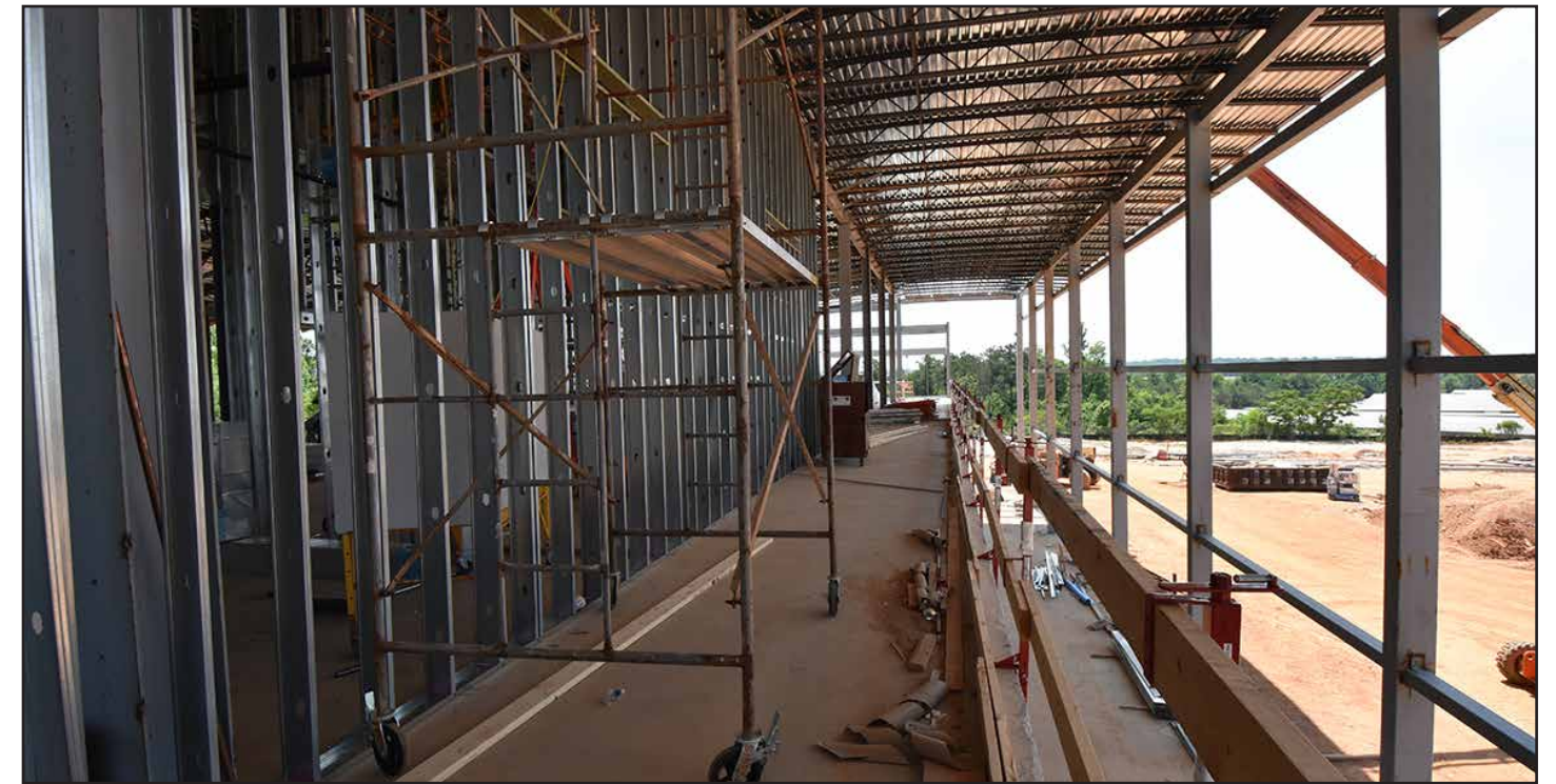
Interior work continues as electrical wiring is placed in the ceilings.
