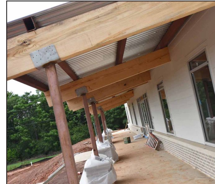
The front porch roof nears completion.
