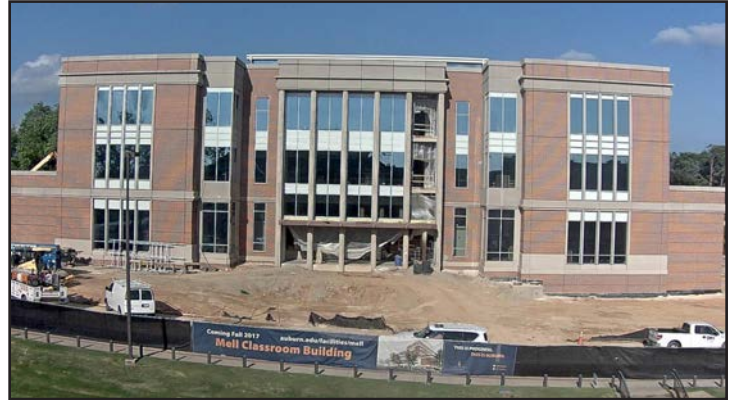
View of the Mell Classroom Building from the project webcam.
