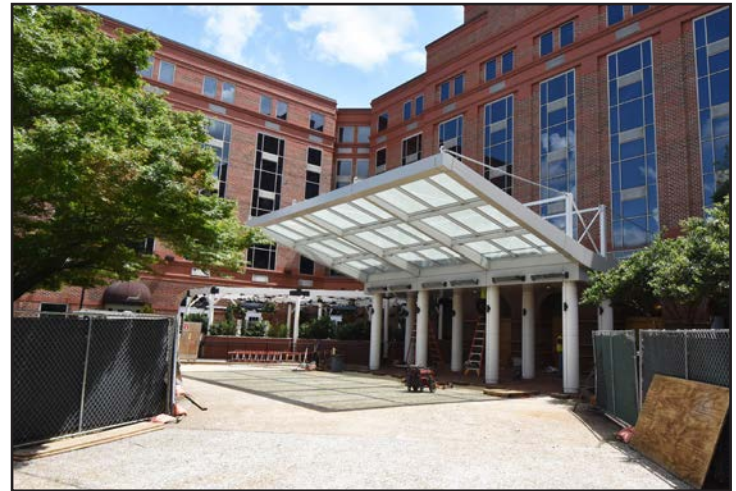
View of the porte cochere looking toward the northeast.
