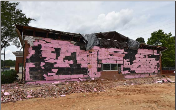
Demolition of the canopy is underway.
