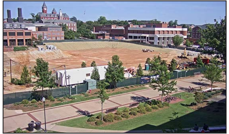
View of the demolition site from the Shelby Center webcam.
