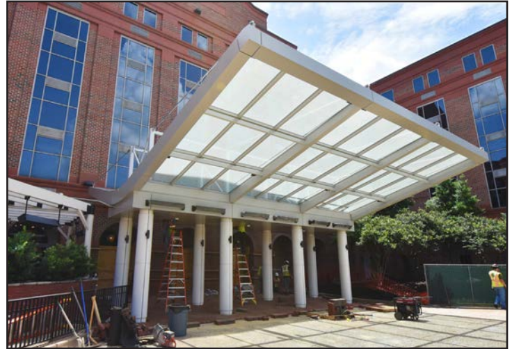
Glass and metal panel installation on the porte cochere is complete.
