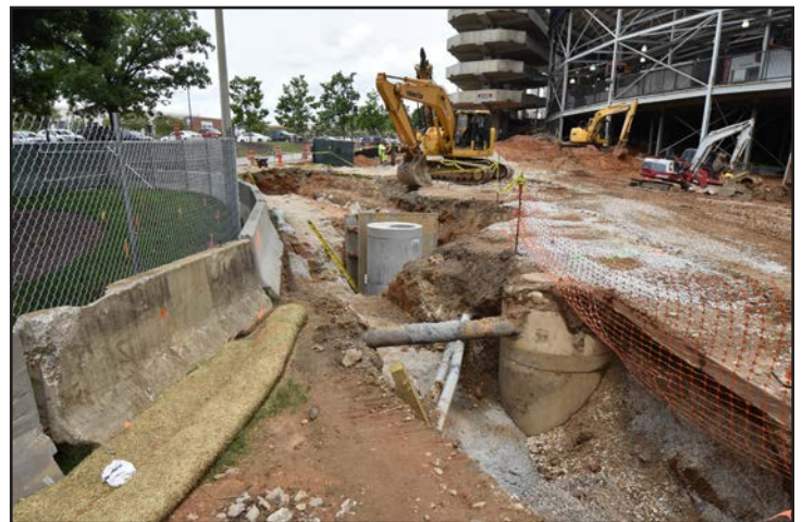
Underground utility work has started.
