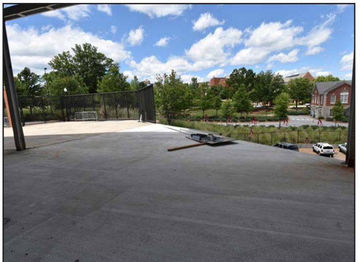
Custom metal railings are being created to accommodate the new concourse.
