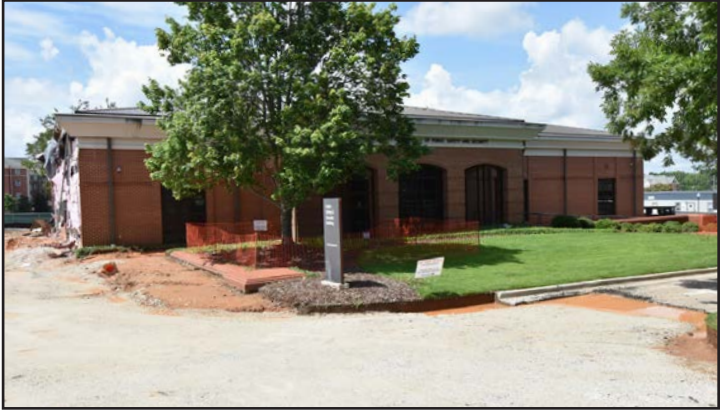
Front view of the Campus Safety Building expansion project.
