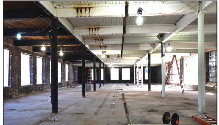
Second floor after demolition.
