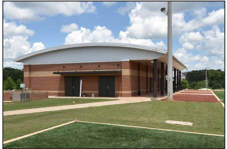
Landscaping is in progress around the storage building
