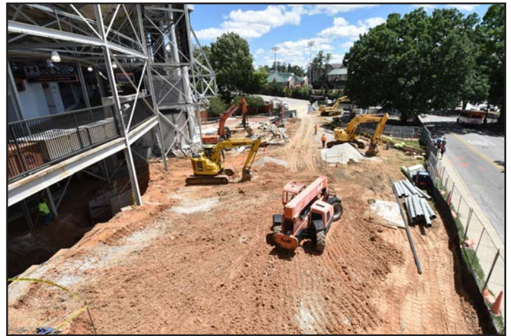
An alternate view of the parking lot demolition.
