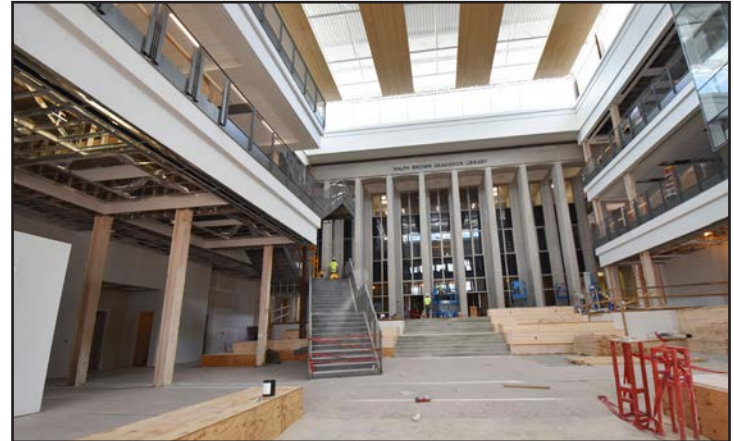
Hand rail installation is under way in the central atrium.
