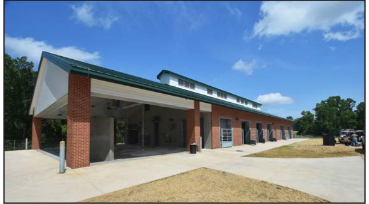
Exterior view of the Food Animal Research Facility.
