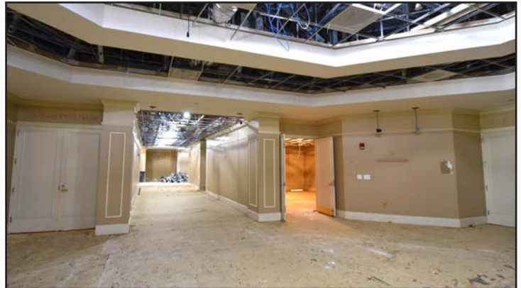
Conference Center demolition is underway.
