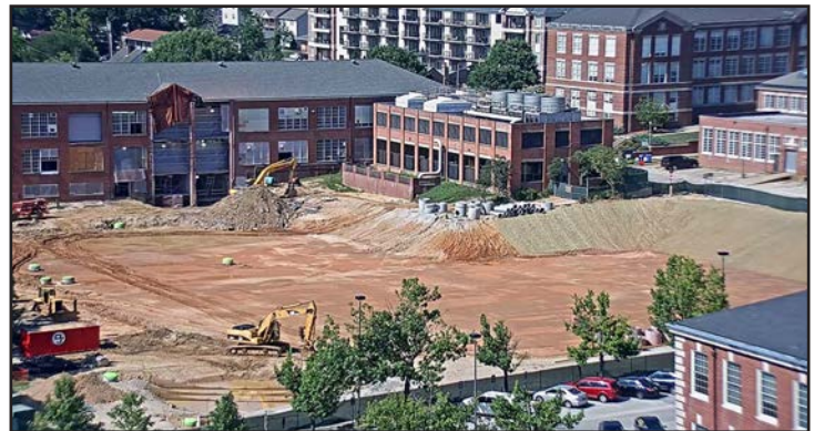
Grading for the Brown-Kopel Engineering Student Achievement Center is underway.
