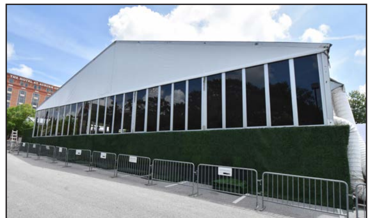
A temporary tent (marquee) has been built in the hotel's parking lot.
