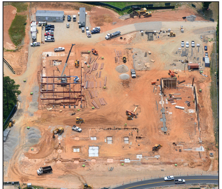
The Pharmaceutical Research Building site is located in the upper left.
