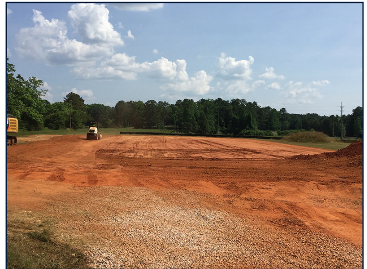
Site pad for Building C.
