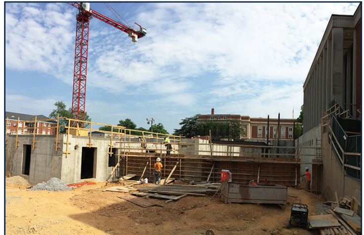
Construction of the lowest level basement wall has begun.
