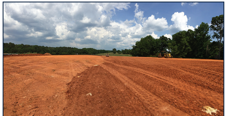
Site pads for Buildings A&B.
