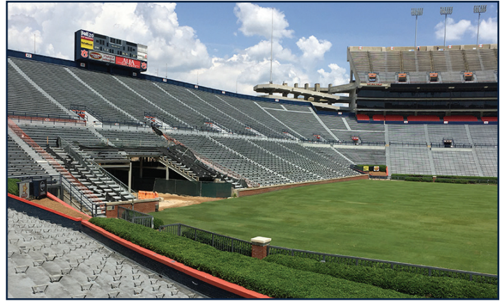
Stadium seating was temporarily removed for the infrastructure project.
