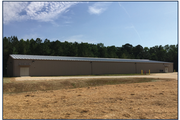
Exterior view of the OLAF facility.
