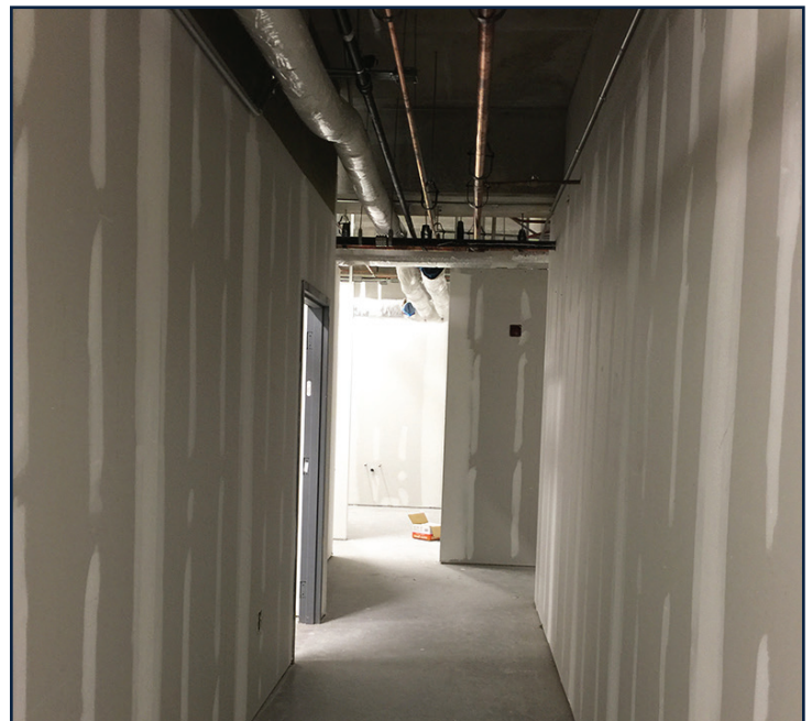
Drywall installation is complete.
