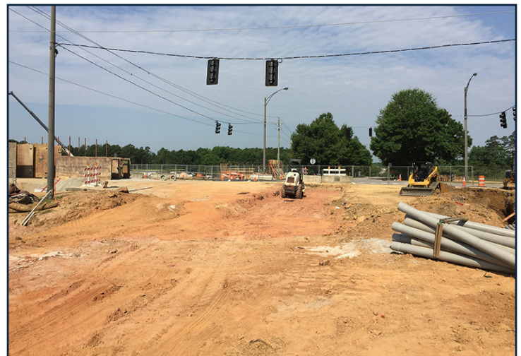
Crews work to run utilities under Lem Morrison toward South Donahue.
