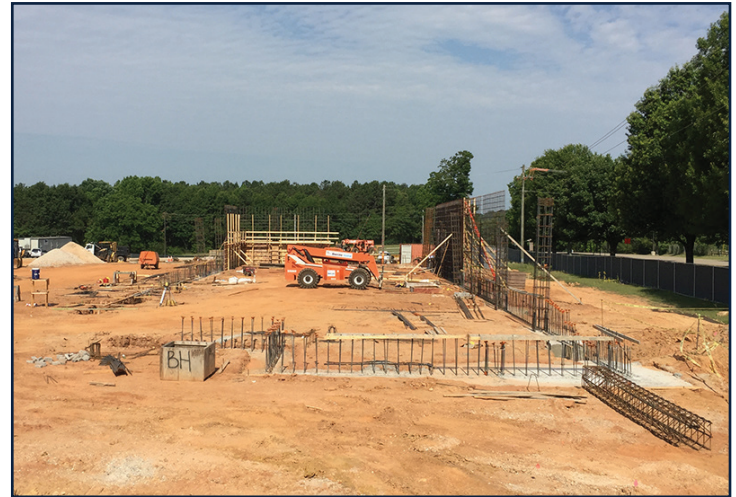
Footings are complete.
