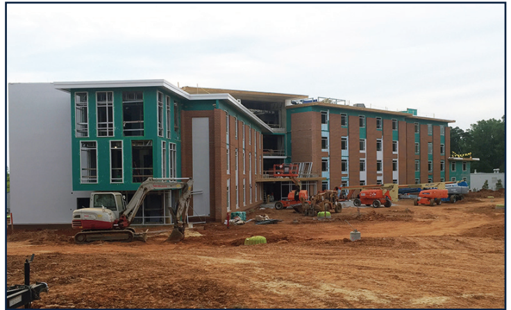
Exterior work nears completion.
