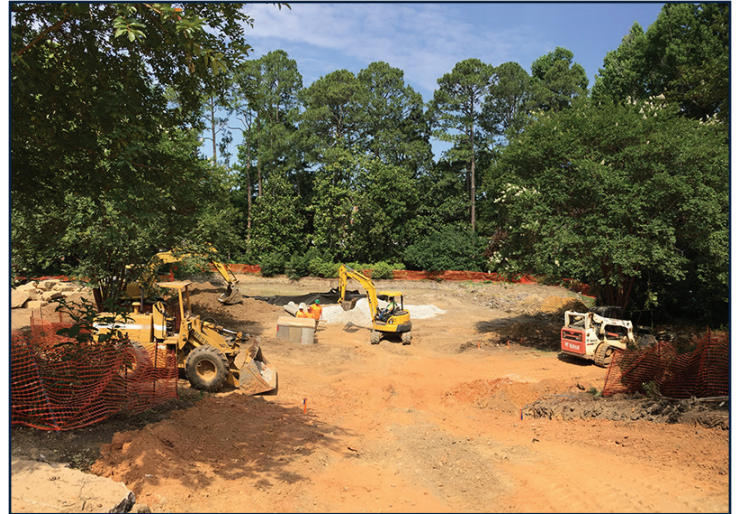
The former pond is being repaired and enlarged.
