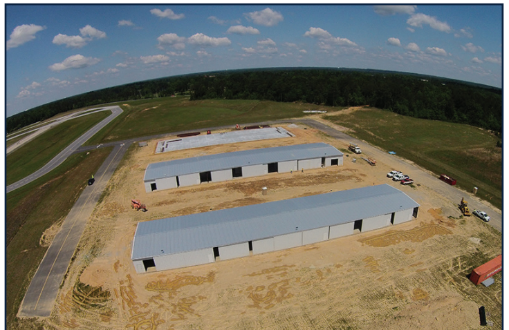
Aerial photo taken prior to construction of the third hangar.
