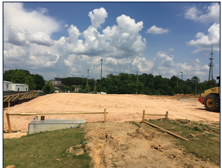
Site grading for the storage building is underway.
