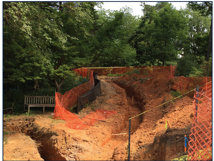
This is the footing for the lower plaza seat wall.
