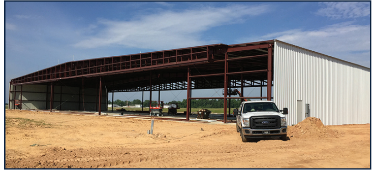
The largest hangar nears completion.
