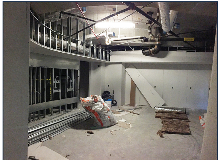
Interior support space.
