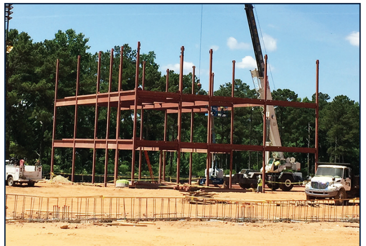
The structural steel frame is being erected.
