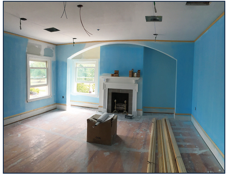
Interior renovations continue.
