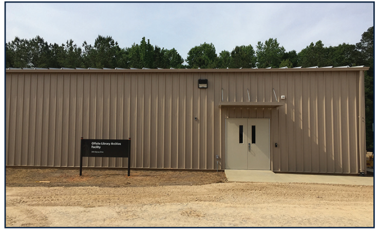
Front view of the OLAF facility.
