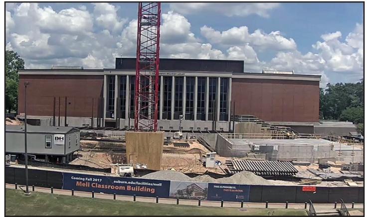
View from the Mell Classroom construction webcam.
