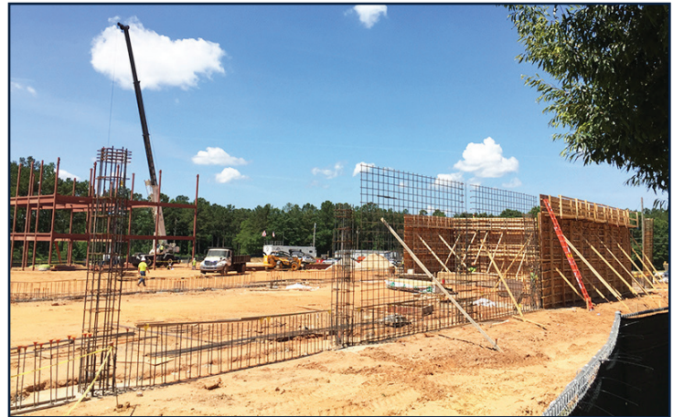
Storm shelter walls are being erected.
