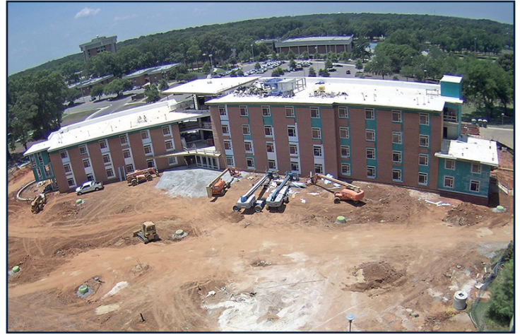
Aerial view of the AUM residence hall construction site.
