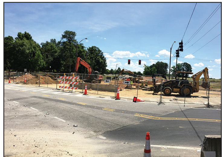
Utility work continues on the east side of South Donahue Drive.
