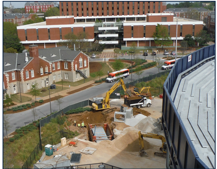
New box culvert extends into the north end zone parking lot.
