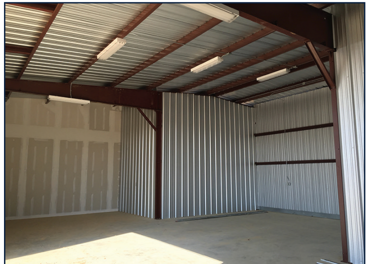
Inside view of one of the new hangars.
