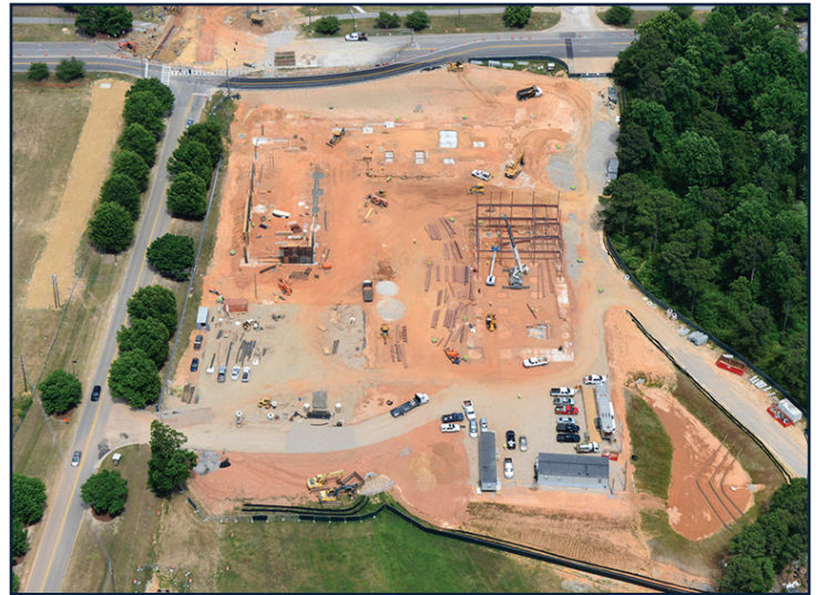
Aerial view of the site taken in early June.
