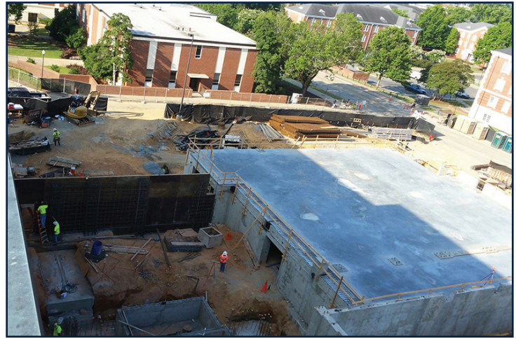
Basement walls are being formed.
