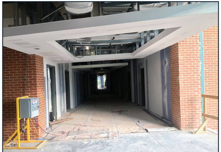
The walls are now framed and drywalled.
