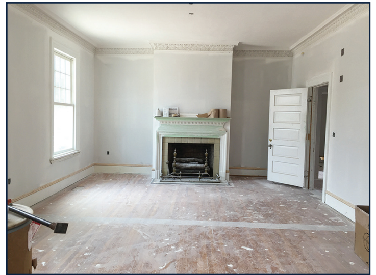
First floor interior work.
