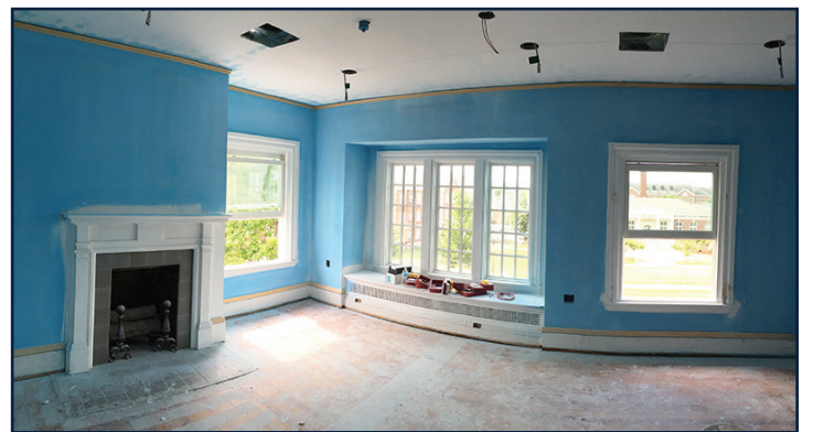
Second floor interior work.
