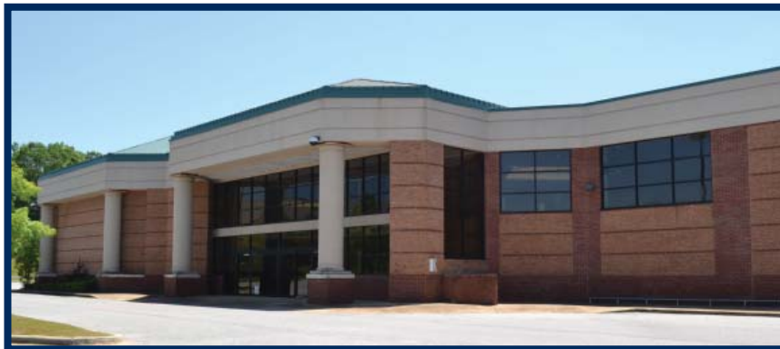
East Glenn Administrative Support Facility
