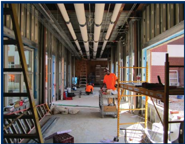
Connector Bridge - First Floor Space
