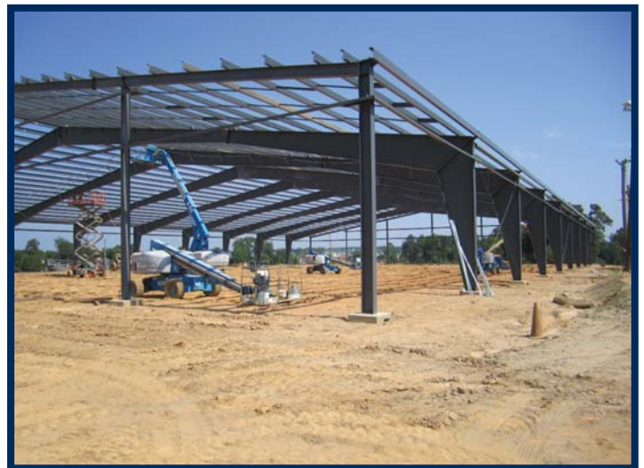
Equestrian Facility Bracing Installation 2
