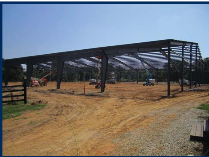
Equestrian Facility Bracing Installation 1
