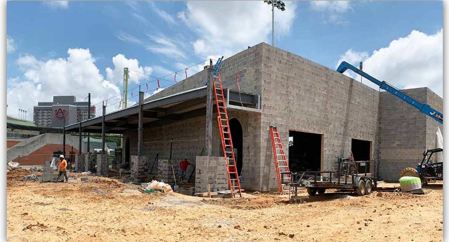
The exterior block installation is nearing completion.
