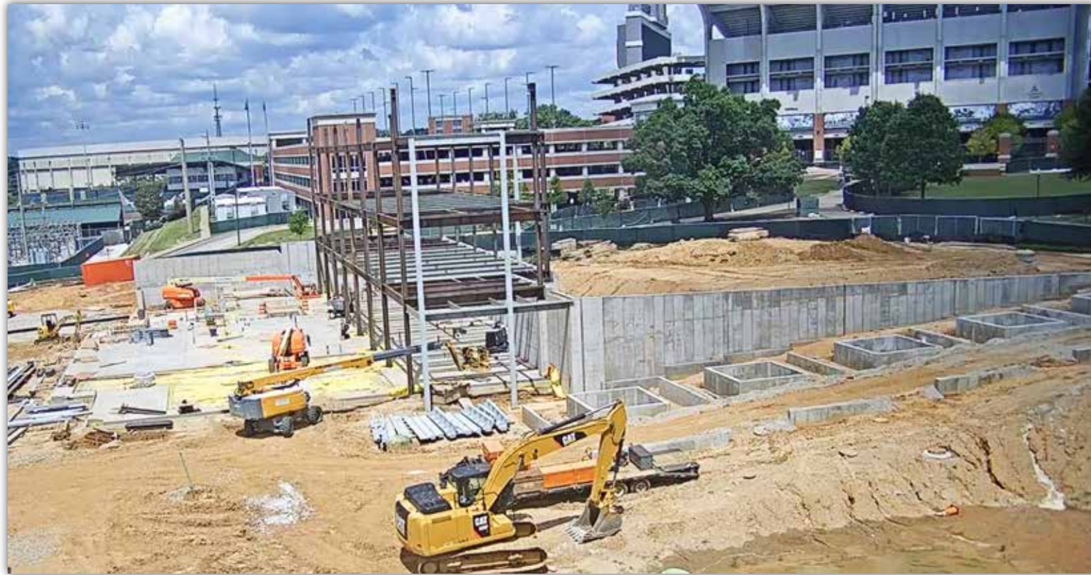
Concrete basement walls are being formed, and the building's steel frame is starting to take shape.
