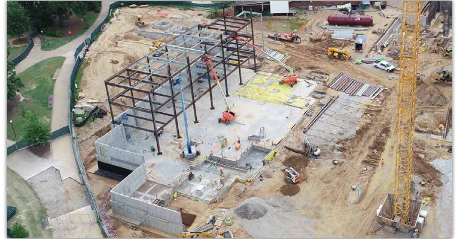
Concrete basement walls are being formed, and the building's steel frame is starting to take shape.
