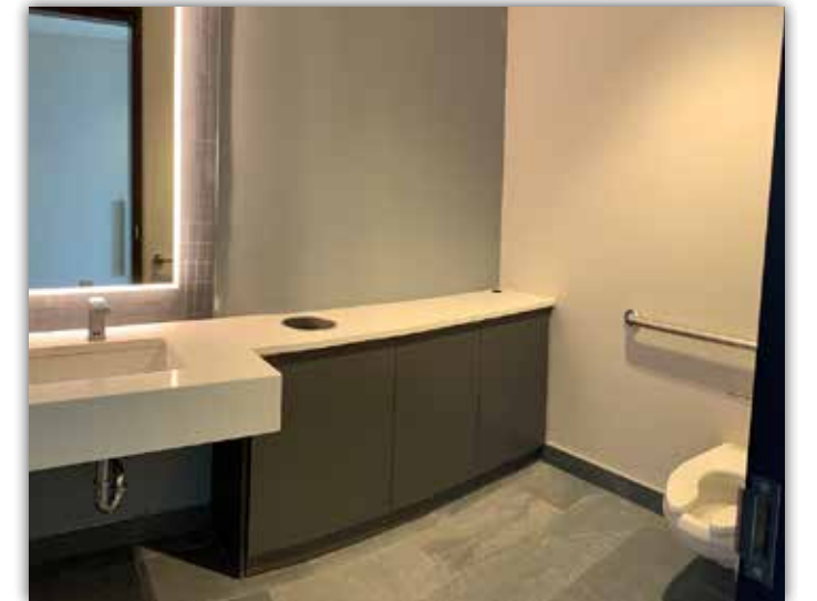
The restrooms also received finish upgrades, including new cabinets and counter tops.
