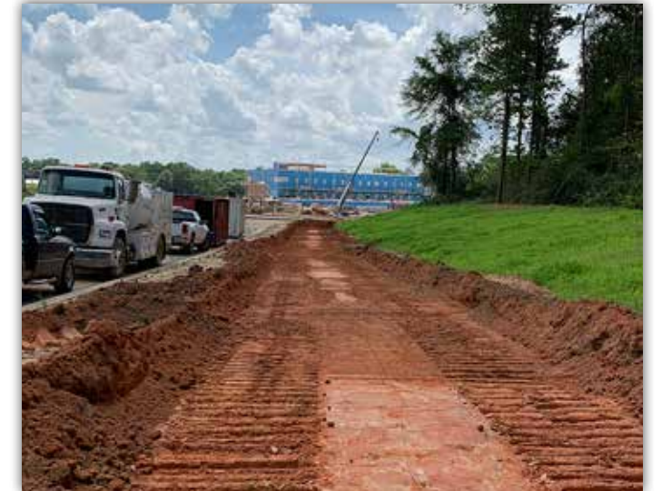
Grading work continues in preparation for new sidewalks.
