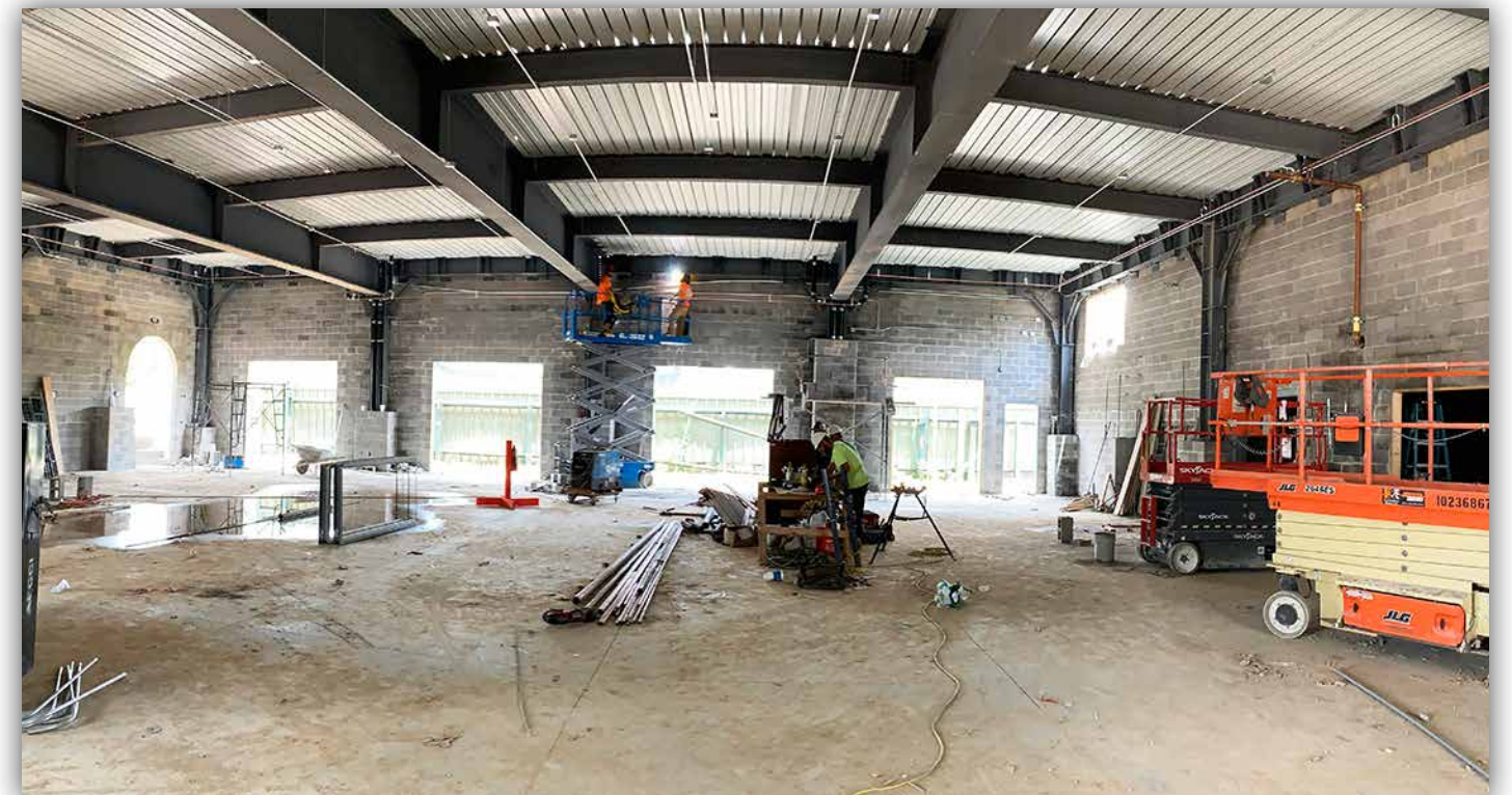
Electrical and mechanical work continues inside the new building.
