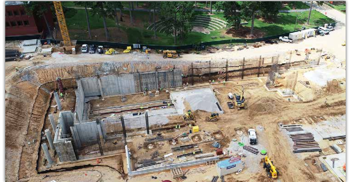
Concrete walls are being formed for the ACLC's storm shelter.
