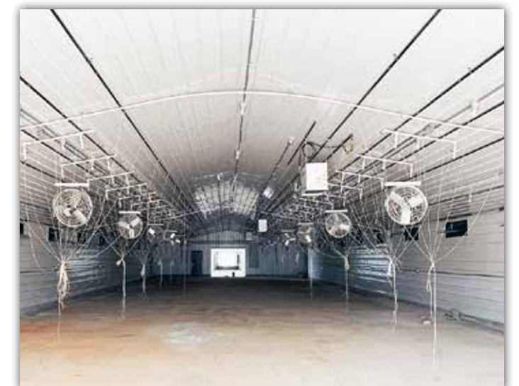
The pen houses are outfitted with ceiling mounted fans and automated controls to regulate internal temperatures.
