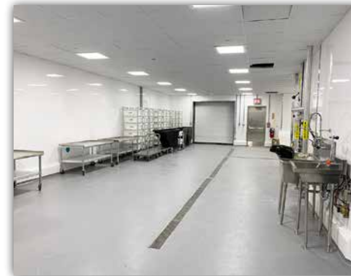
Equipment has been placed in the processing plant.
