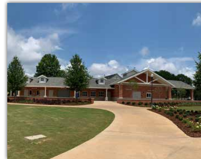
There are several walkways leading from the field house to the five new fields.
