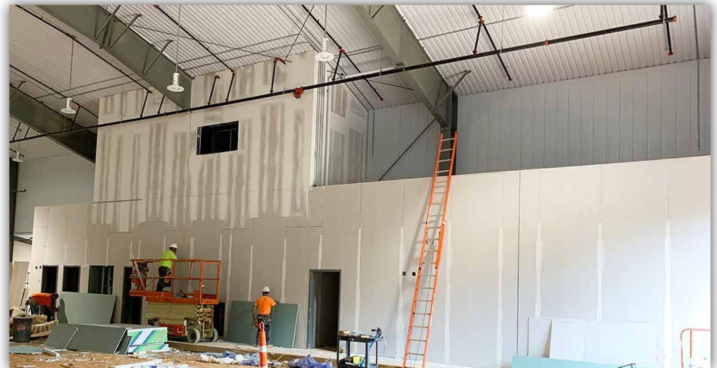
The walls for the administrative offices are being prepared for paint.
