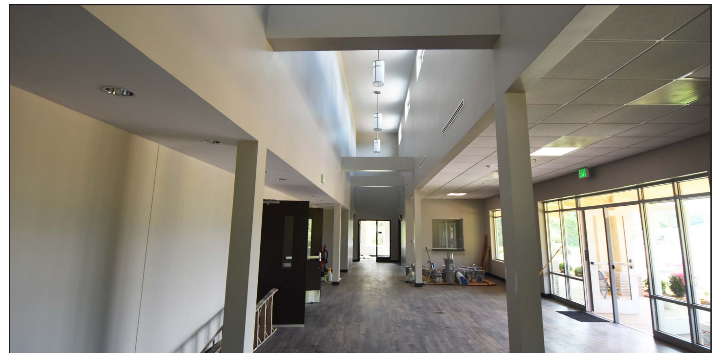
Final cleaning is taking place for the main entry.
