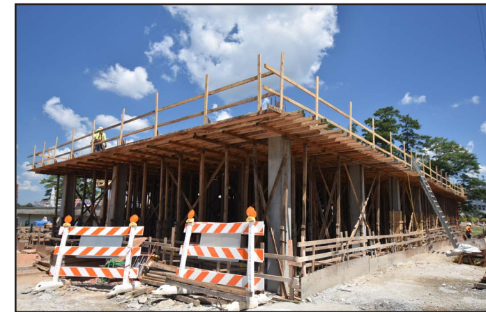
Concrete columns are being erected for the addition.
