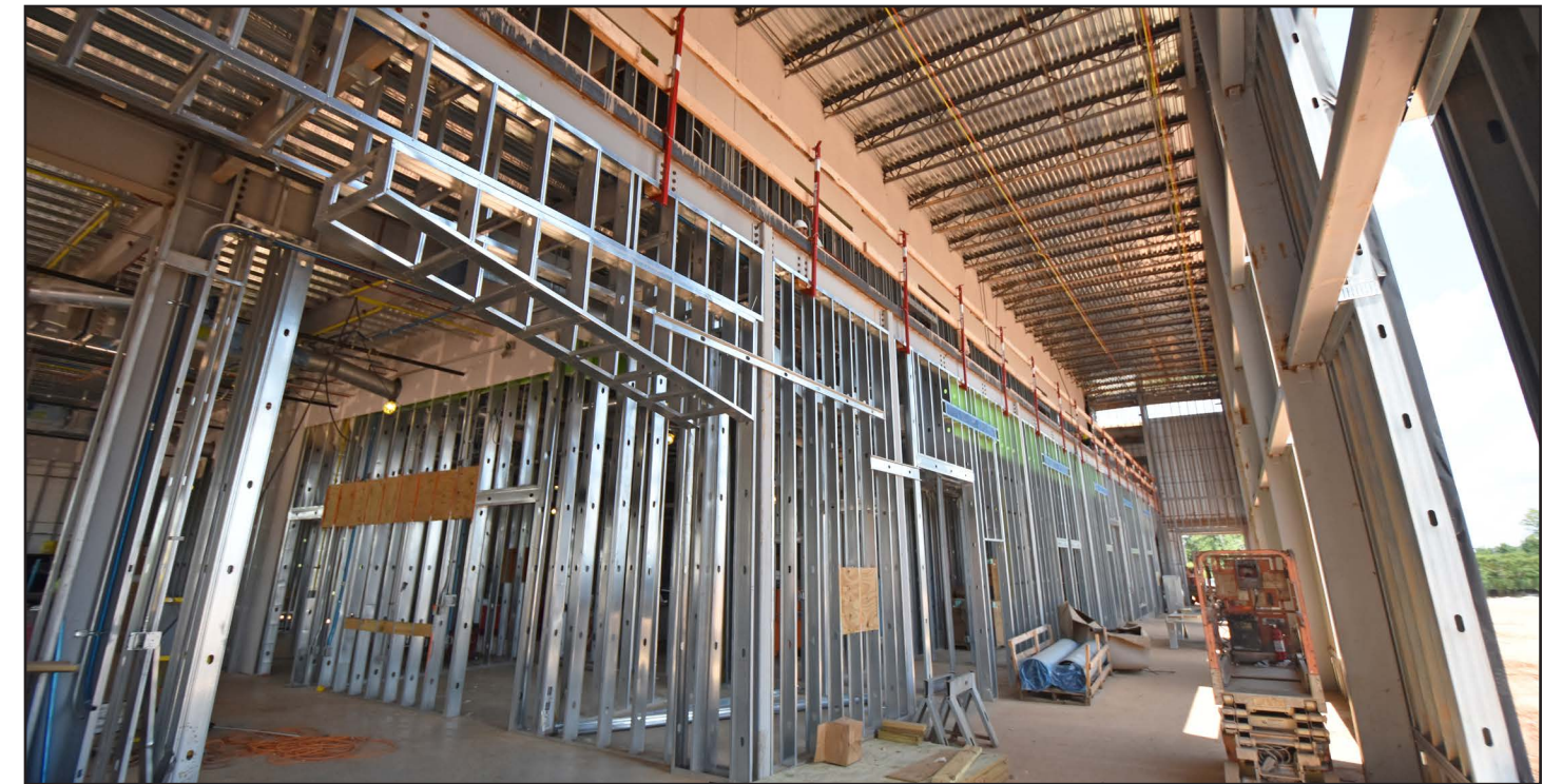
Interior framing continues for the classroom spaces.
