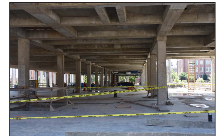
The building's interior is now ready for steel studs.
