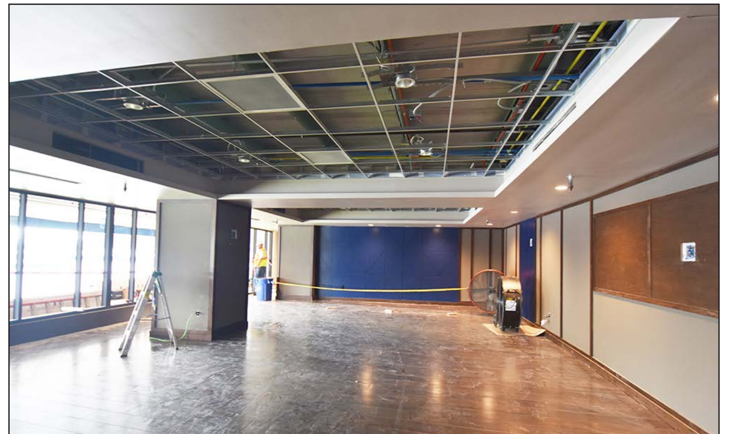
Wood flooring has been installed in the lobby area.
