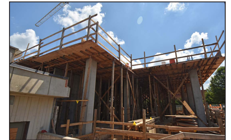
Columns are being formed for the second floor.
