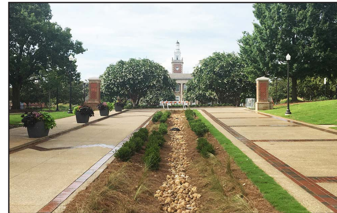
A completed section of the Mell Corridor shows the eco swale, bike lane, sidewalks and entrance portals.
