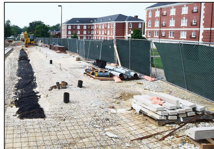
Work on Phase IV concourse construction is underway.
