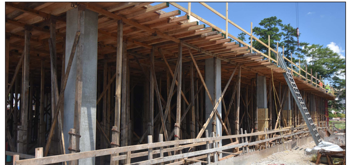
The second floor is beginning to take shape.
