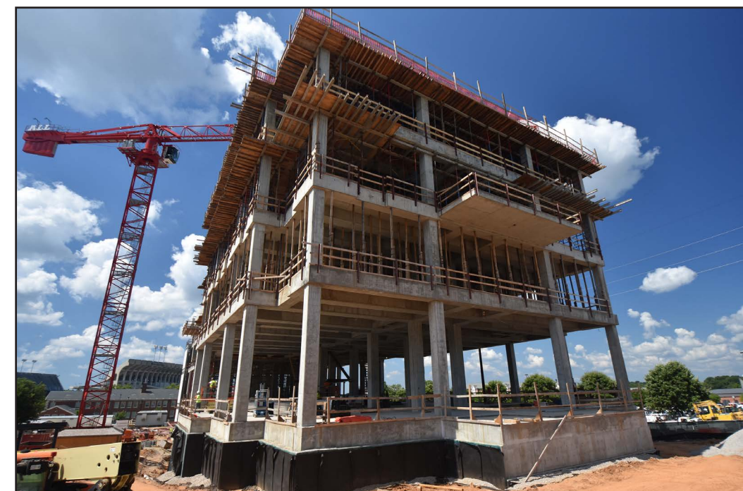
Structural steel work on the roof to begin later this month.
