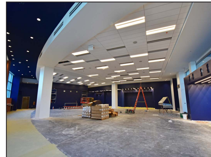
Painting has begun inside the recruiting lounge.
