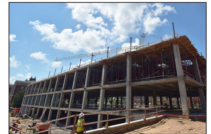
A view of the building's completed concrete structure.
