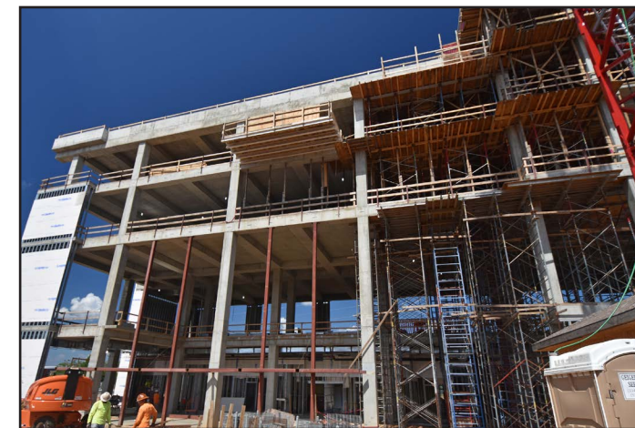
This atrium, bottom left, will house the student commons area.
