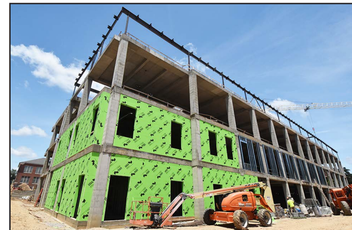
Exterior insulation is being installed.
