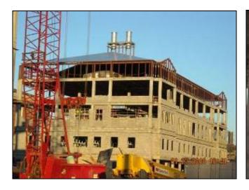
Concrete frame, exterior block and roof structure underway.
