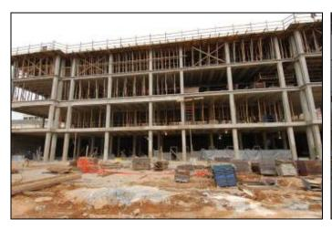
Exterior view of reinforced concrete frame construction. #
