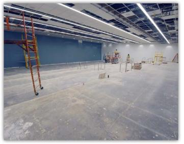
This ground floor tiered lecture hall is being prepared for wood wall features, ceiling tiles and floor finishes.
