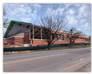
*Installation of precast brick wall panels continues on the indoor practice facility.*
