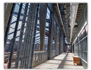
Metal wall framing is nearing completion in this hallway overlooking the indoor practice facility.
