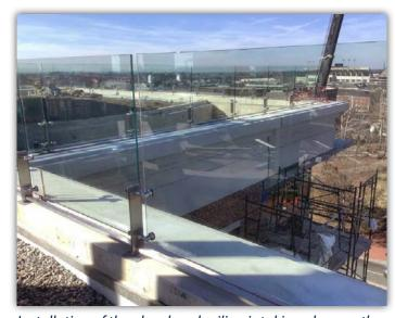
Installation of the glass hand railing is taking place on the rooftop terrace.
