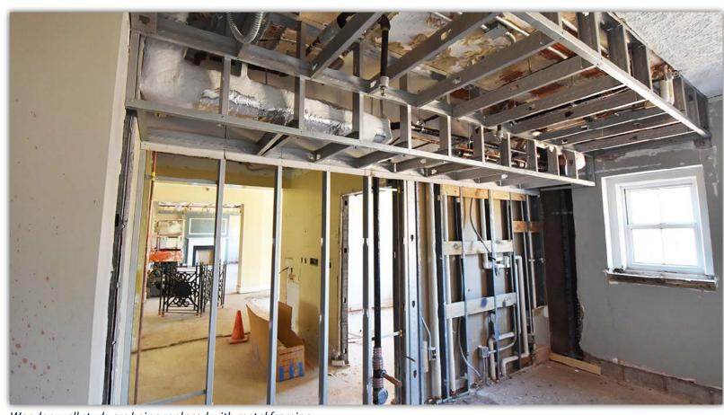
Wooden wall studs are being replaced with metal framing.
