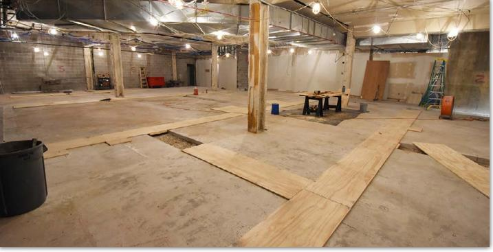
Interior demolition is complete, and trenches have been drilled for placement of electrical wiring.
