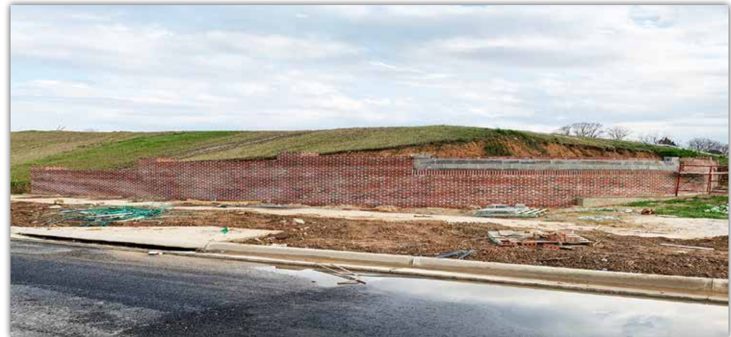
Brick entrance structures are being constructed at Shug Jordan Parkway.
