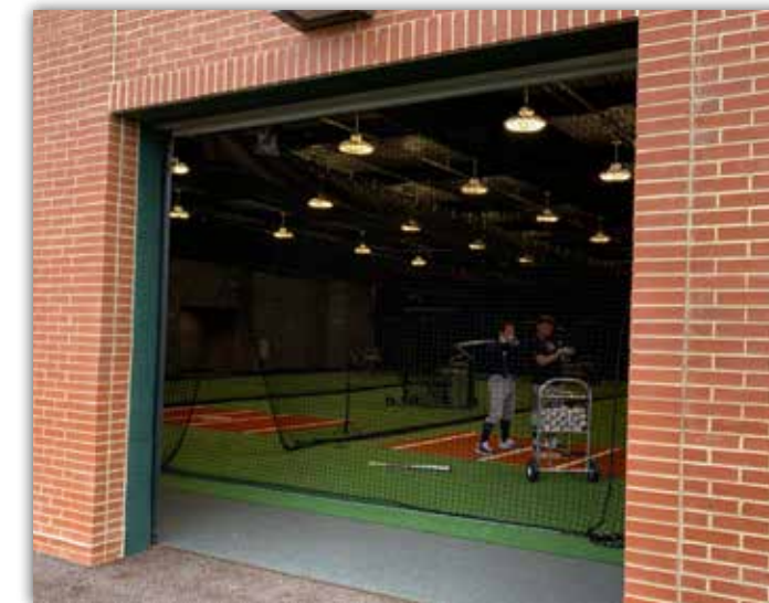
Several large garage doors like this one are used to provide cross ventilation.
