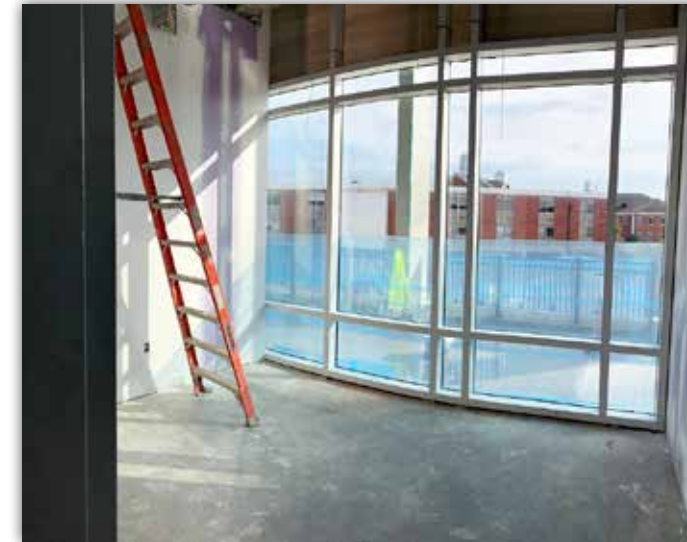
Painting has begun in this dining area on the first floor.
