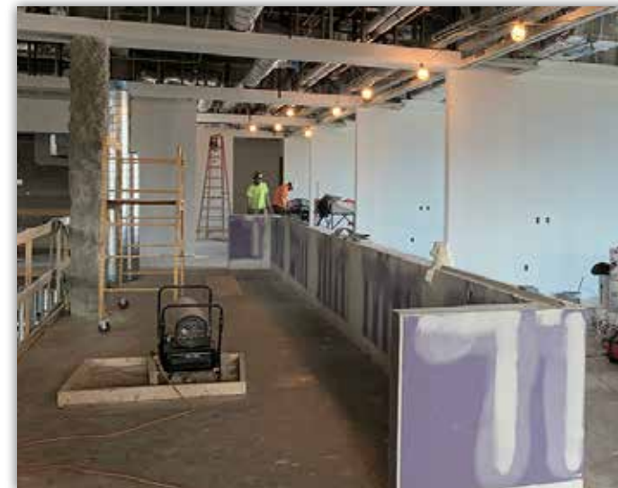
This open area on the second floor will provide access to the reservable dining/study rooms. The low wall, for booth seating, is almost ready for a coat of paint.
