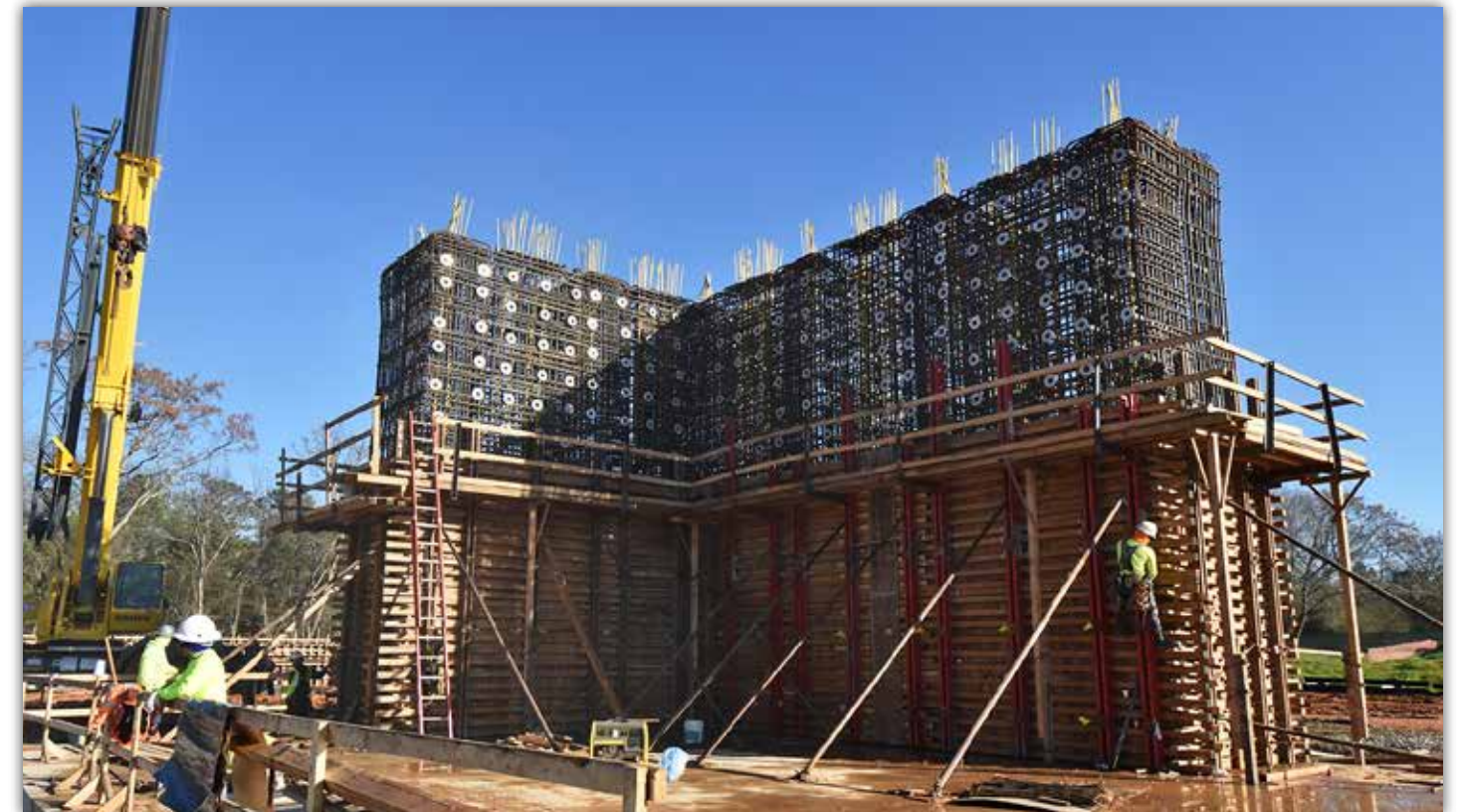
Wood framing secures concrete recently poured for the strong wall.
