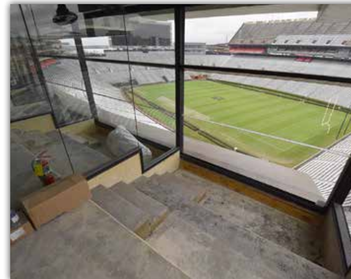
The tiered section of this suite is ready for new carpeting and fixed seating.
