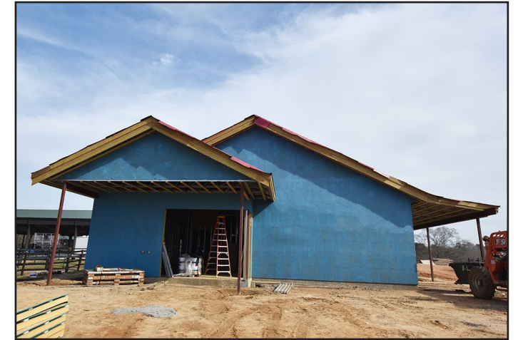
The team support building will soon be ready for concrete siding.
