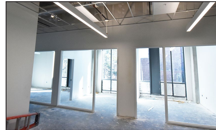
Staff offices located on the second floor.
