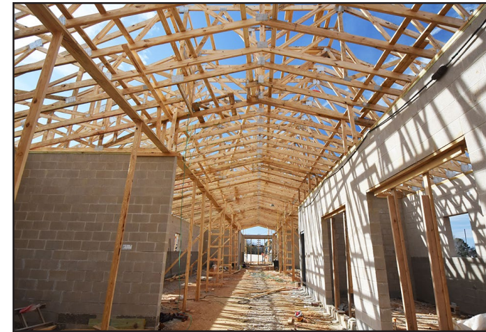
Wood roof trusses have been installed on the barn.
