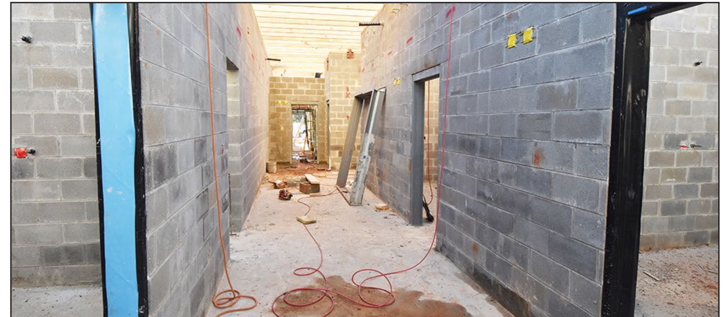
Framing for the interior walls and doorways is underway.
