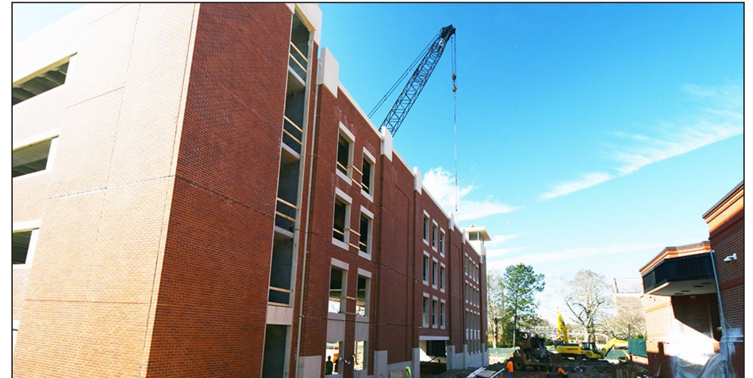
A northeast view of the parking deck showing precast concrete panels.
