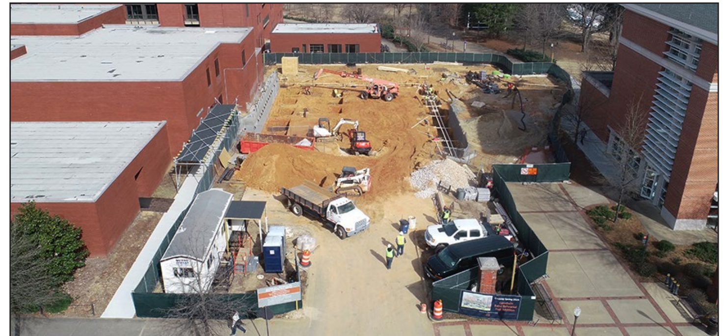
An aerial view of the site and utility work currently underway.
