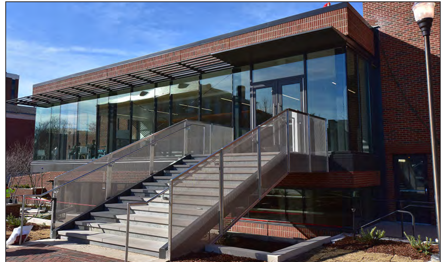
The new pavilion provides a new entrance and additional lighting to the front of Broun Hall.
