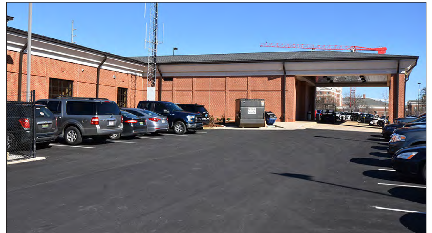
The building expansion and additional parking spaces created during construction.
