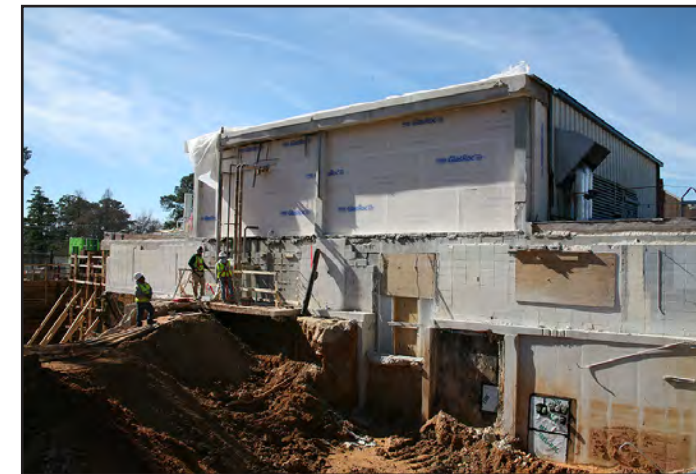
Work continues on the addition's basement excavation.
