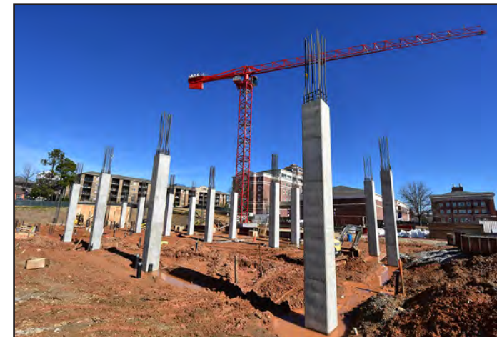
These concrete columns will support the building's first floor.
