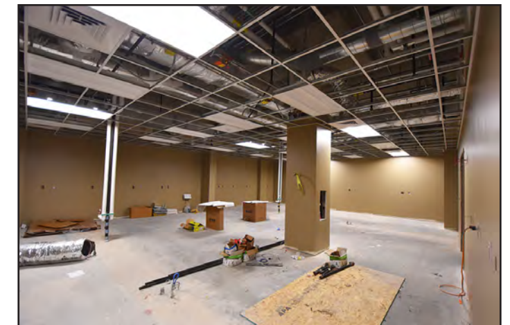
Ceiling lights are complete with ceiling tile to follow.
