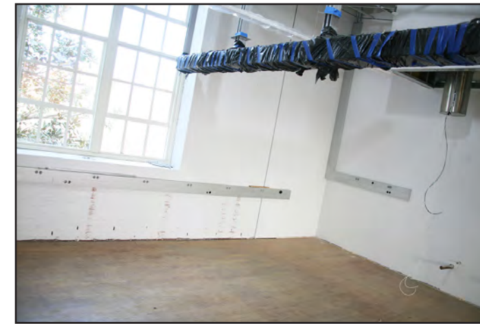
Drywall installation continues.
