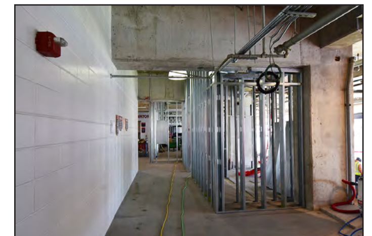
Interior wall framing is well underway for the new club space and coaches' booths.
