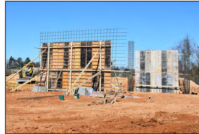
Concrete walls are going up for the safe room.
