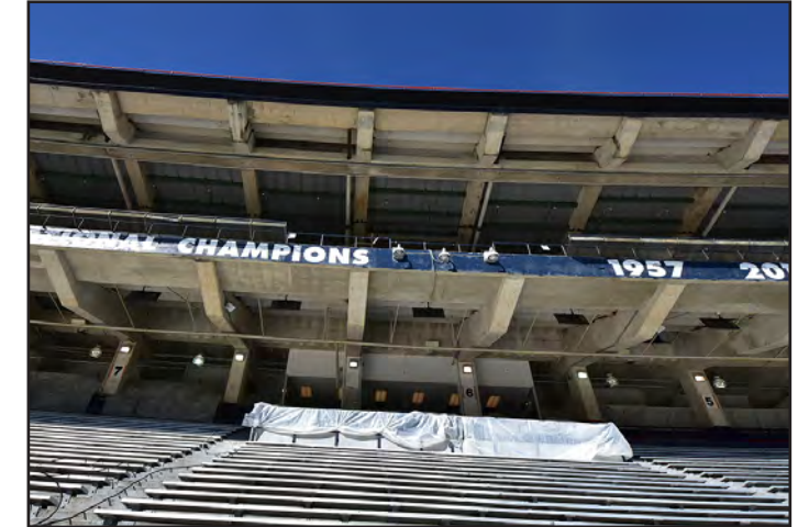
A view of the construction site from within the stadium.
