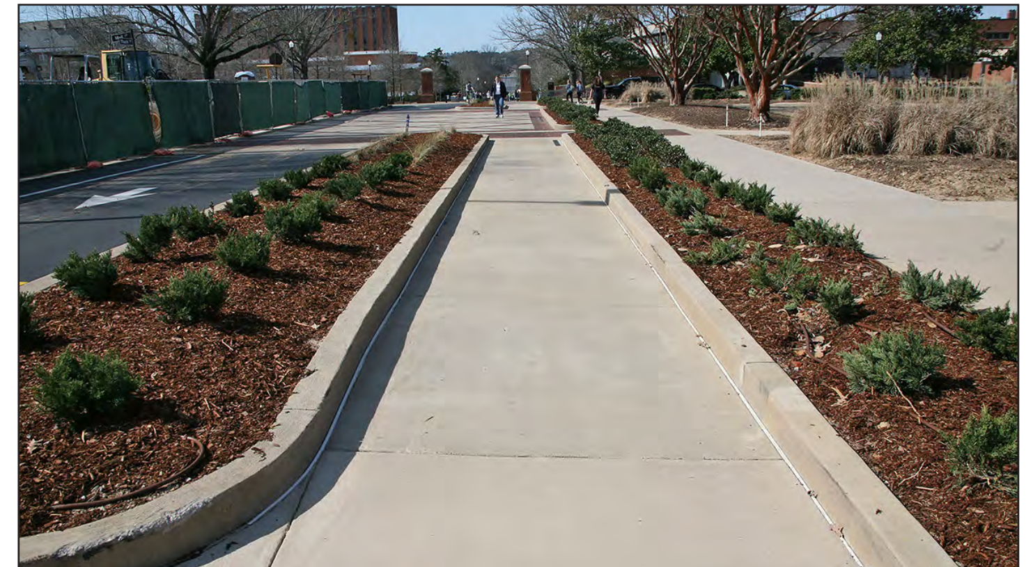
Phase I included the addition of a bicycle only lane.
