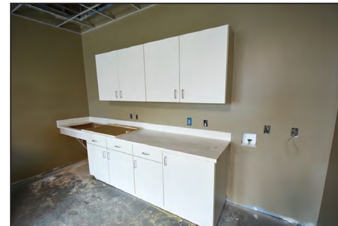
Cabinet installation in a support space.
