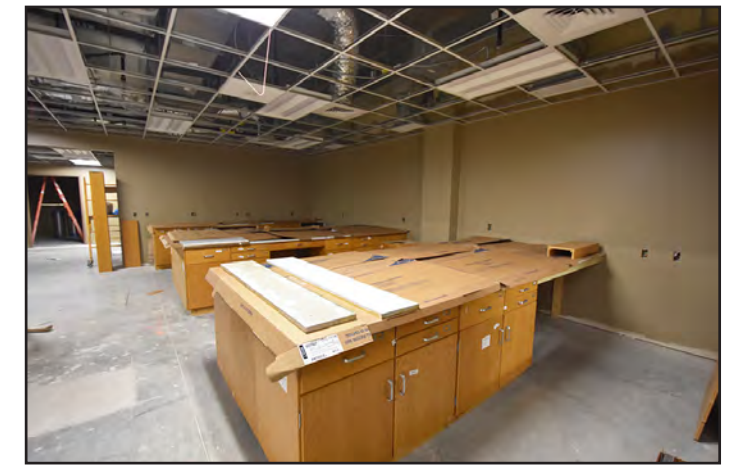
Laboratory cabinet installation nears completion.
