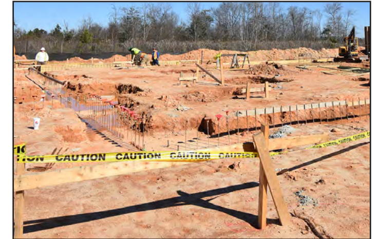
The building foundation work has begun.
