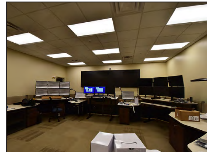
Installation of the new operations center equipment.
