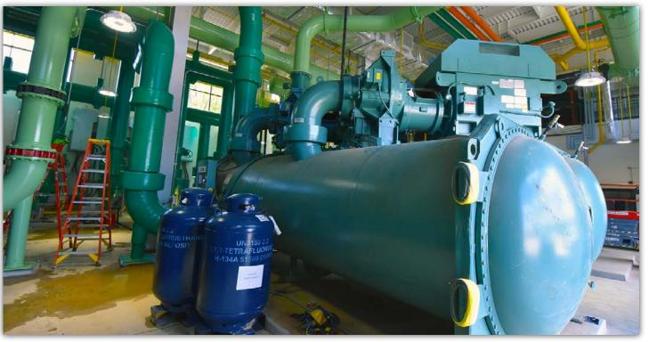
The two 2.500-ton chiller units have been installed.
