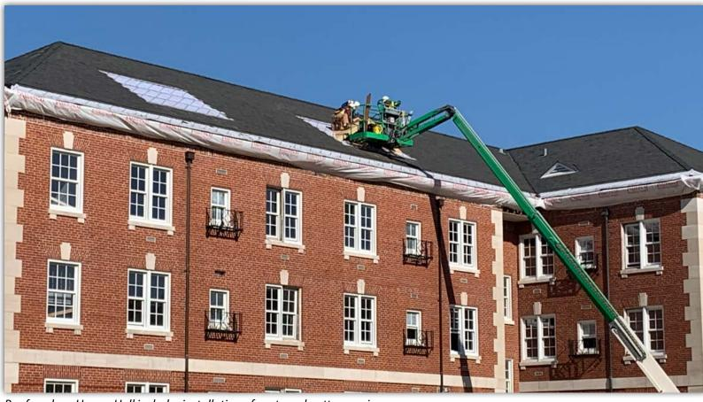
Roof work on Harper Hall includes installation of vents and gutter repairs.
