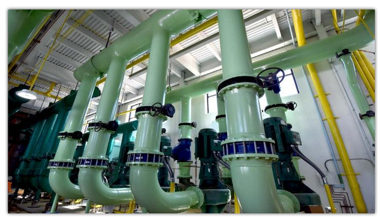
Installation of chilled water system piping, which will distribute chilled water to facilities across campus, is complete.
