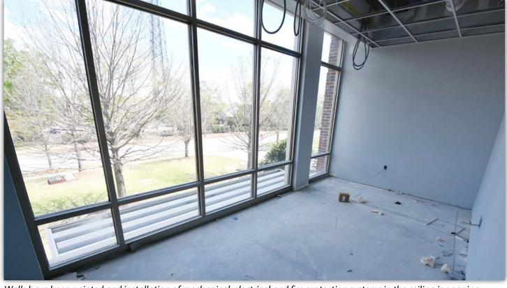
Walls have been painted and installation of mechanical, electrical and fire protection systems in the ceiling is ongoing.
