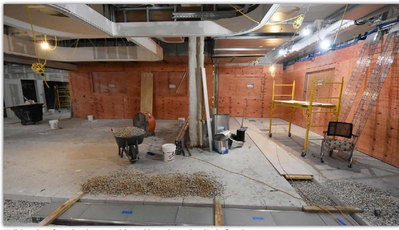
Walls have been framed, and power and data cables are being placed in the floor ducts.
