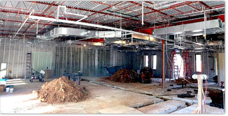
Installation of overhead mechanical, electrical and fire protection systems is underway inside the Dawson Building.
