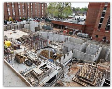
Concrete formwork is ongoing at the underground loading dock along with preparations for the future food hall concrete slab.
