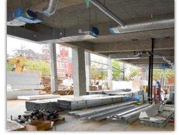
Overhead mechanical duct work is being installed in the future 1856 Restaurant and Dining Room.
