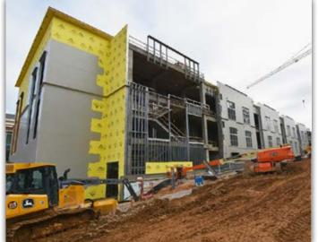
Waterproofing is nearing completion on the south side of the ACLC.
