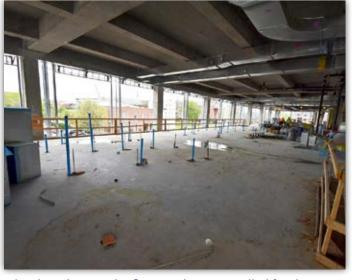
Plumbing lines in the floor are being installed for the distilled spirits and wine appreciation labs.
