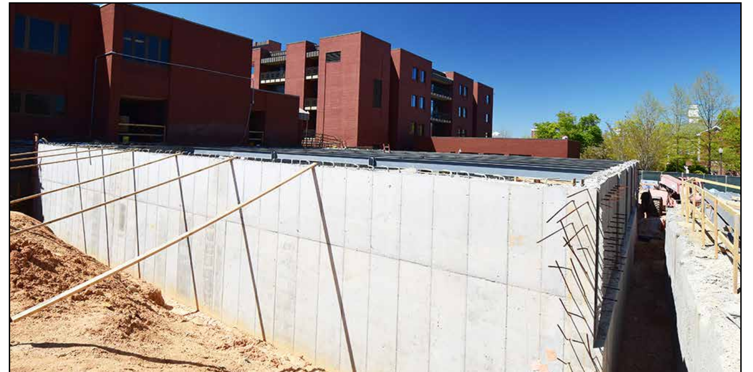
A view of the completed concrete basement walls.
