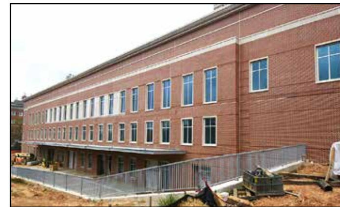
A view of the back of the building, which faces Foy and Tichenor Hall.
