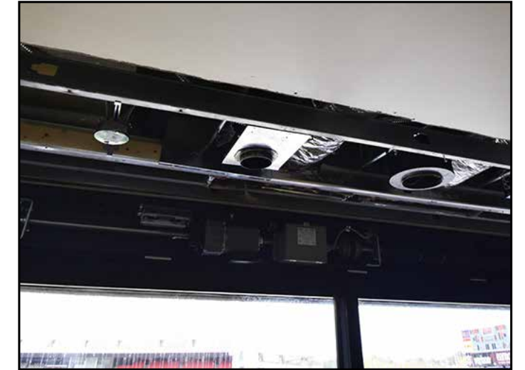
Overhead mechanical work continues on the fourth level.
