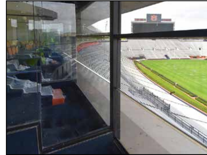
A close-up view of an open window on the third level.
