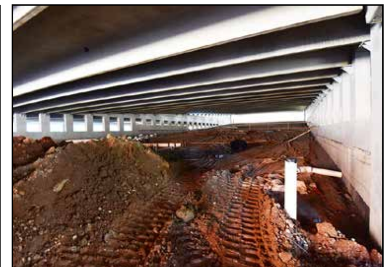
Construction of the ramps within the parking deck are underway.
