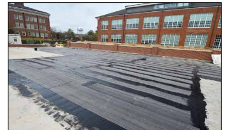
Waterproofing is underway as part of the elevated plaza.
