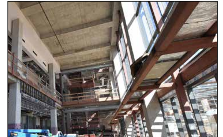
The two-story atrium includes a glass curtain wall facing the Lowder Courtyard and Lowder Business Building.
