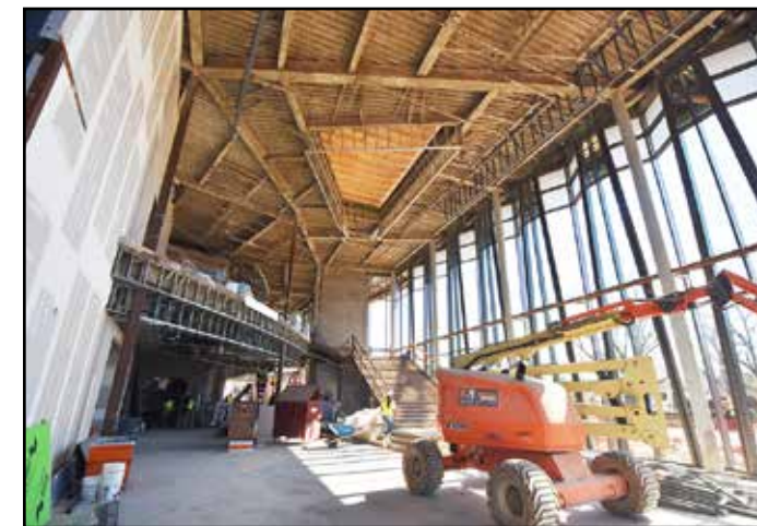
Window installation takes place in the main lobby area.
