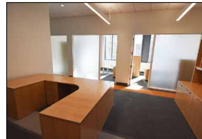
Furniture is being installed in the administrative offices.
