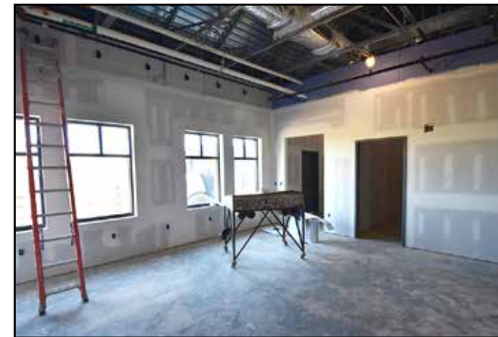
The team training room located inside the new support building.
