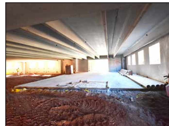
The concrete floor is being poured on the ground level.
