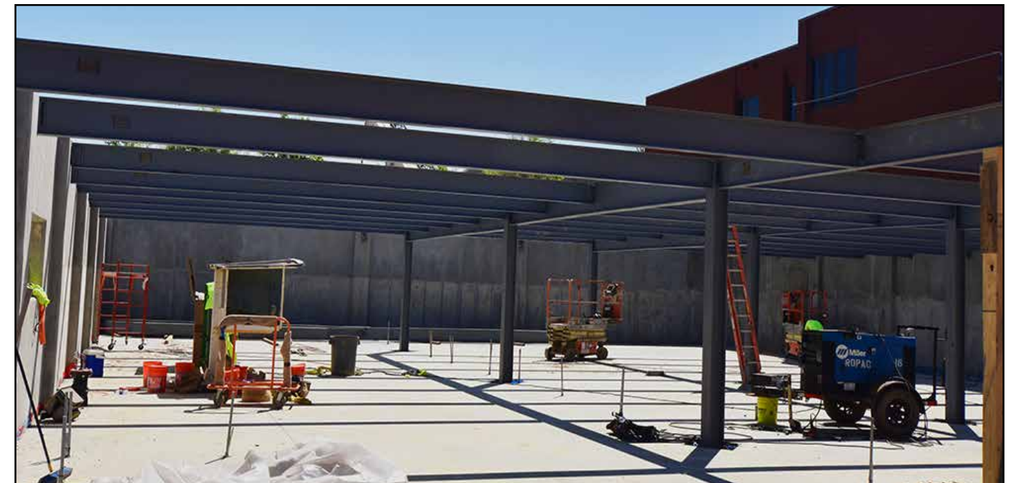
Steel beams are being installed for the basement ceiling.
