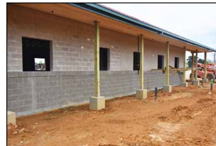
Exterior finish work on the barn is underway.
