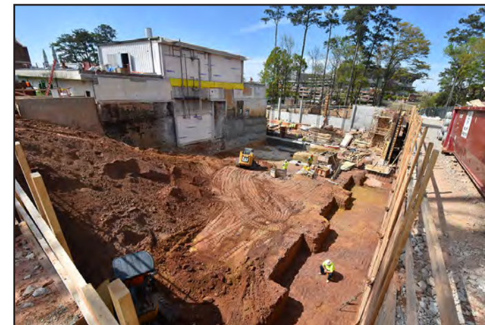
Work continues on the addition's basement excavation.
