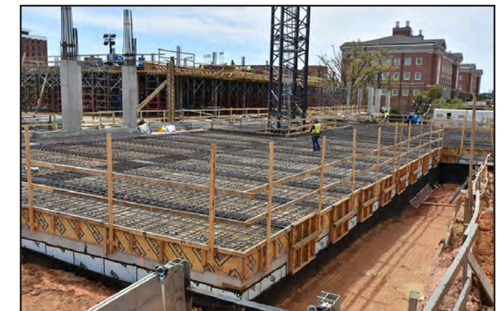
The plaza level is being prepared for concrete.
