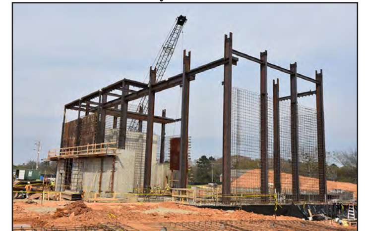
Structural steel installation continues for this project.
