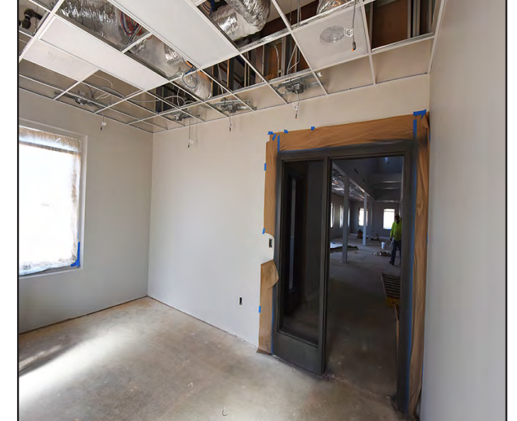
Ceiling tile installation continues.
