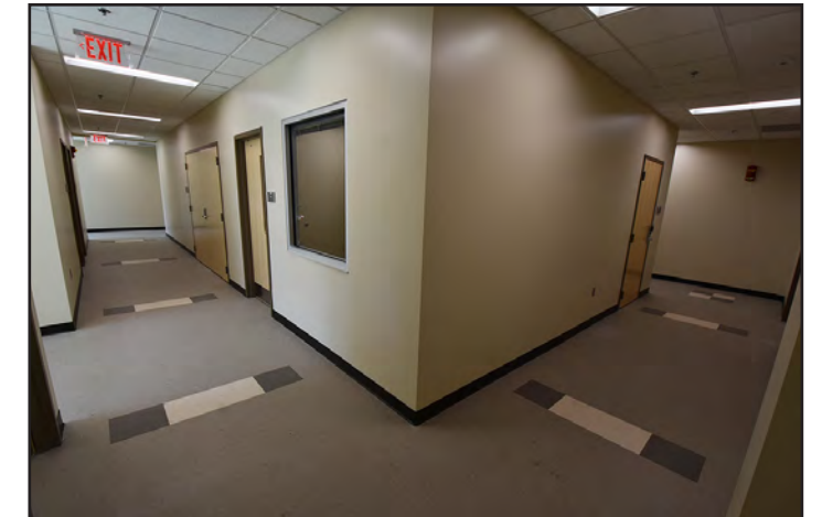
New walls create departmental and office space.
