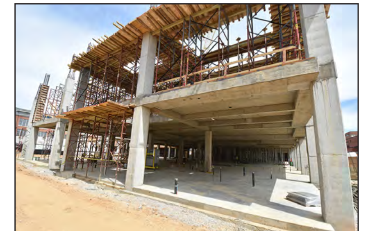
The first floor concrete is making progress.
