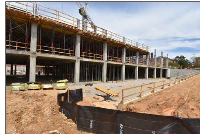
The second floor is beginning to take shape.
