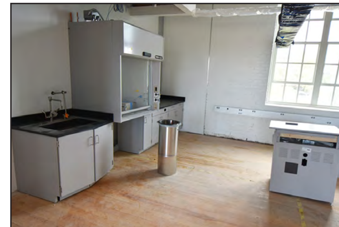
Installation of laboratory casework.
