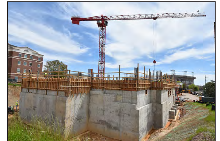
Reinforced concrete walls for the storm shelter.
