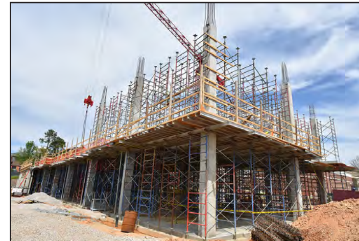
The second level concrete slab currently is being formed.
