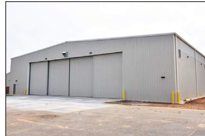
An exterior view of where the planes access the hangar.
