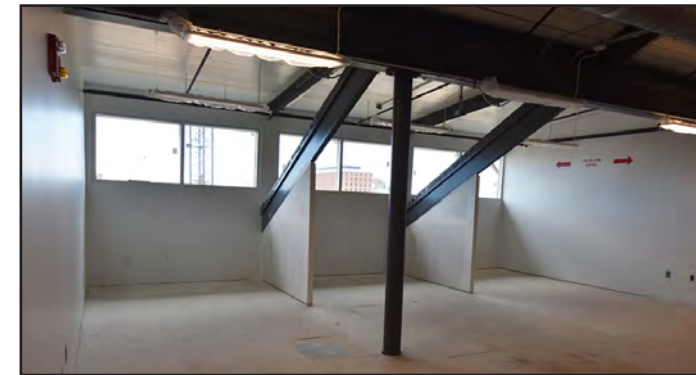
New attic office space is nearing completion.
