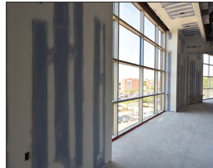
Sheetrock installation continues throughout.
