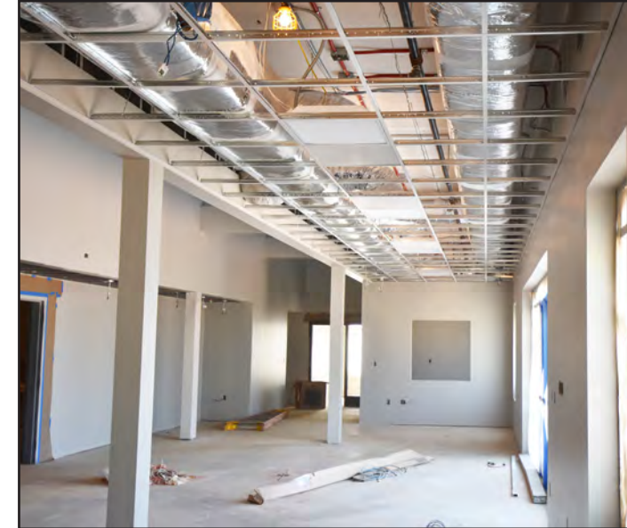
Interior painting is almost complete.
