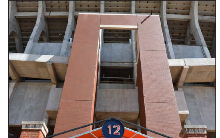
The new club space elevators are enclosed by concrete and brick.
