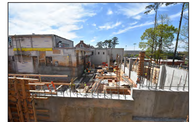
Reinforced concrete form the basement walls.
