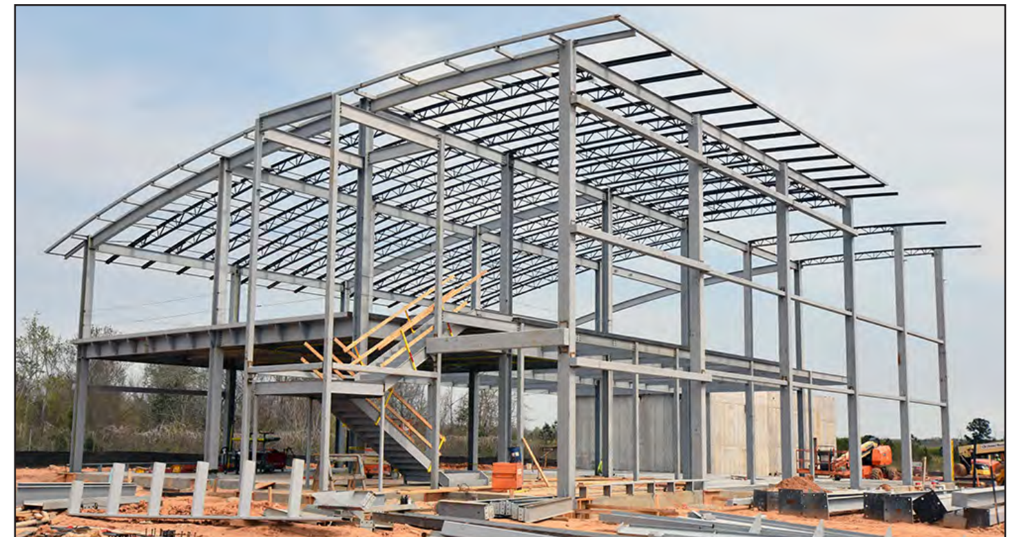
The building's structural frame is 60 percent complete.
