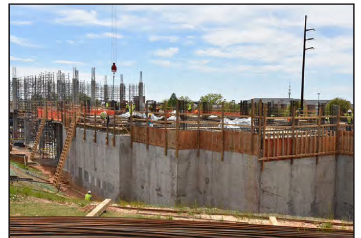
A view of the project from Magnolia Avenue.
