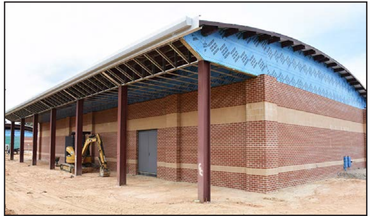
Brick masonry is complete on the storage building.
