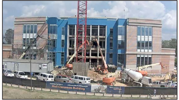
View from the Mell Classroom construction webcam.
