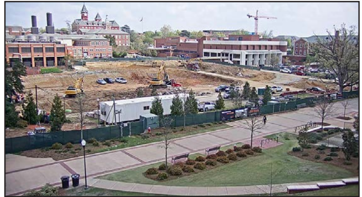
View of the demolition site from the Shelby Center webcam.
