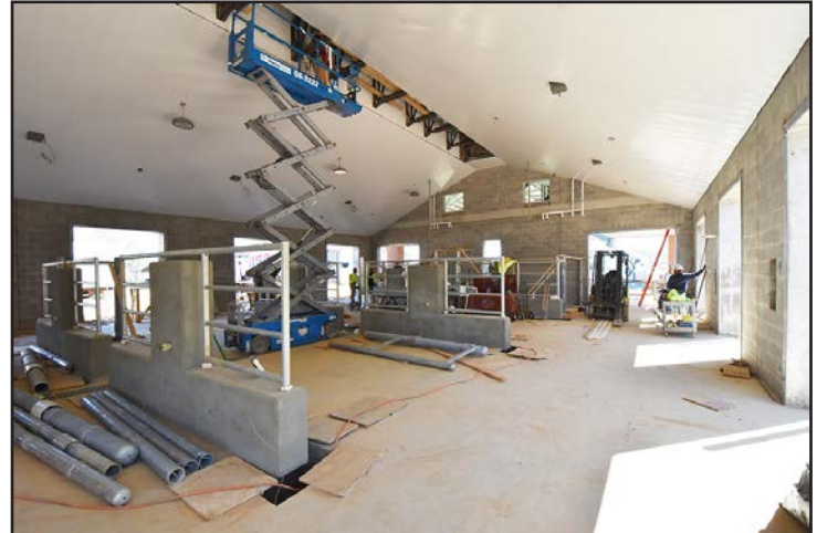
View of the interior fence panels for the food animal stalls.
