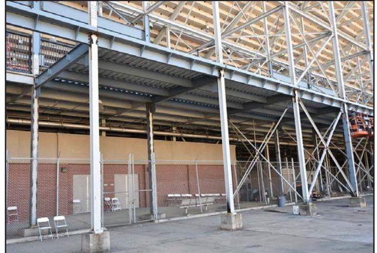
Underside view of the concourse expansion's metal decking.
