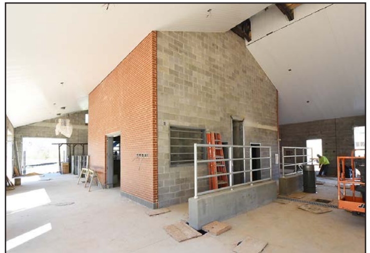
View of the tack room.
