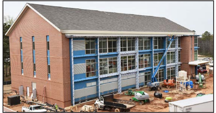
Metal panel installation has begun on the front of the building.
