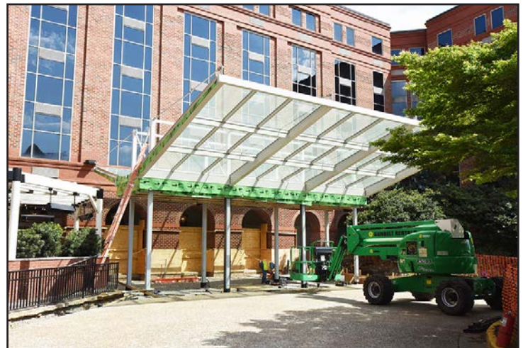
Northern view of the porte cochere construction site.
