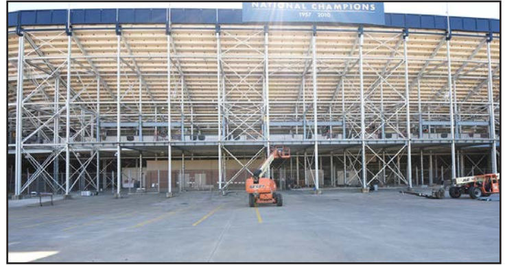
Concourse widening construction site.
