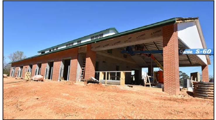
Exterior brick masonry is complete for the Food Animal Research Facility.
