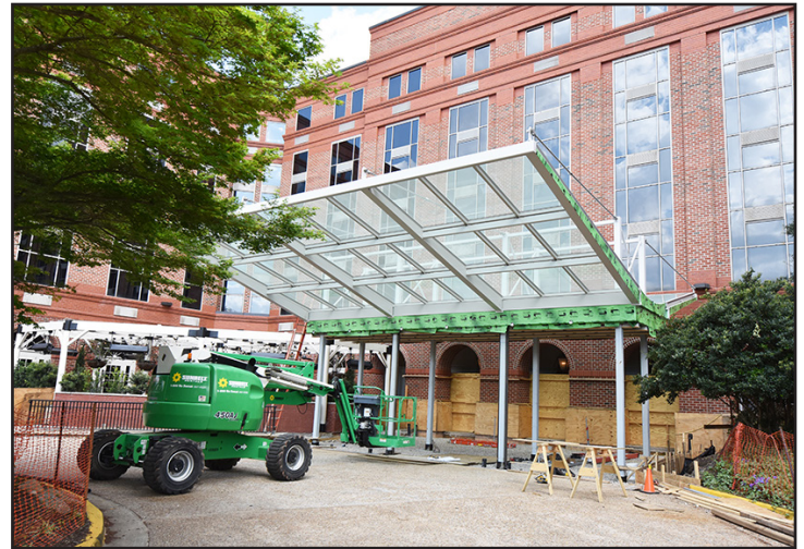
Glass installation is in progress.
