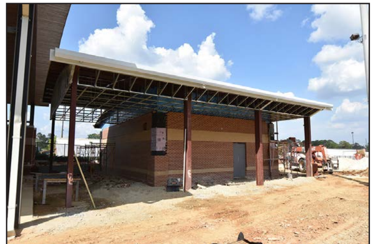
Brick masonry continues on the men's dressing room.
