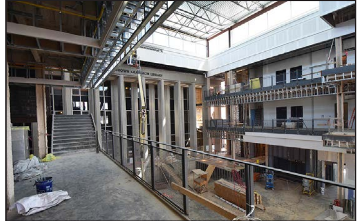
Rail installation is underway in the central atrium.
