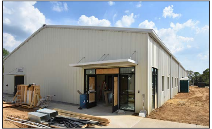
Entrance to the Risk Management and Safety Building.
