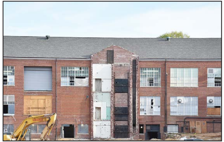
A stairwell once located behind Gavin has been removed.
