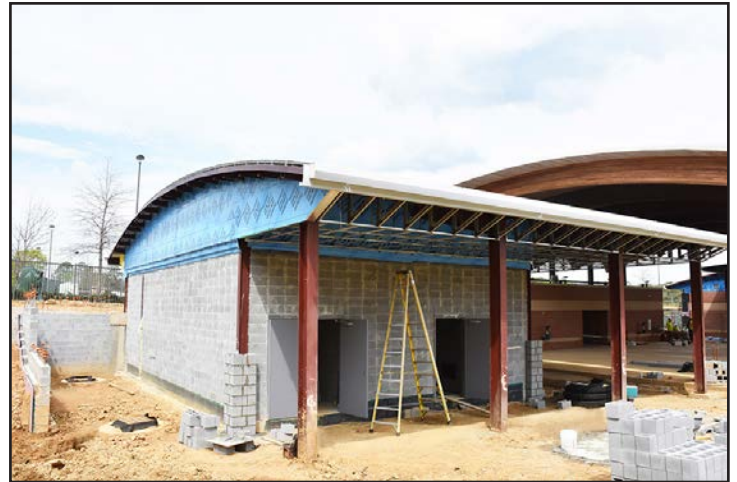
Block masonry continues on the women's dressing room.
