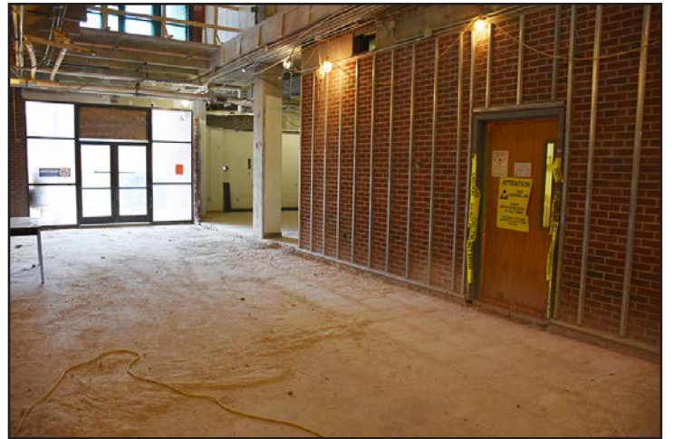
Construction on the ground floor.
