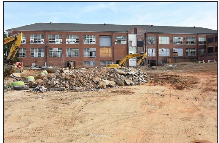
Remaining concrete and masonry demolition waste.
