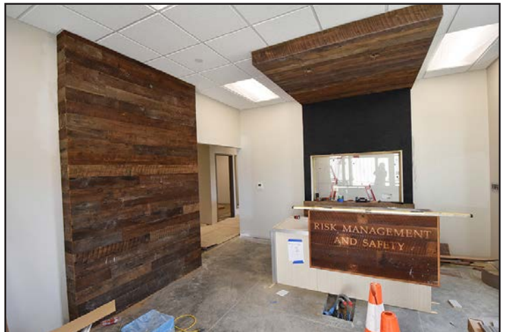
Installation of reclaimed wood within the lobby area is complete.
