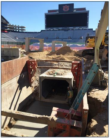
Six-by-8 box culvert being installed underneath the north end zone.
