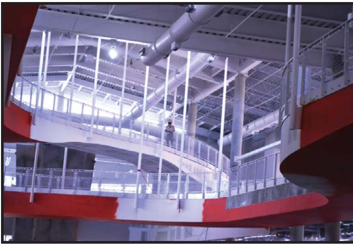
Elevated indoor track
