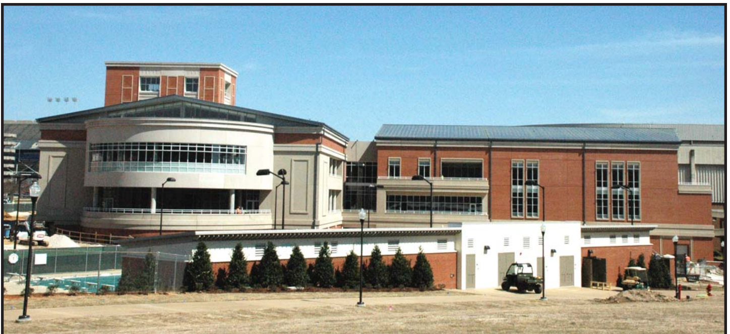
Aerial view of west elevation
