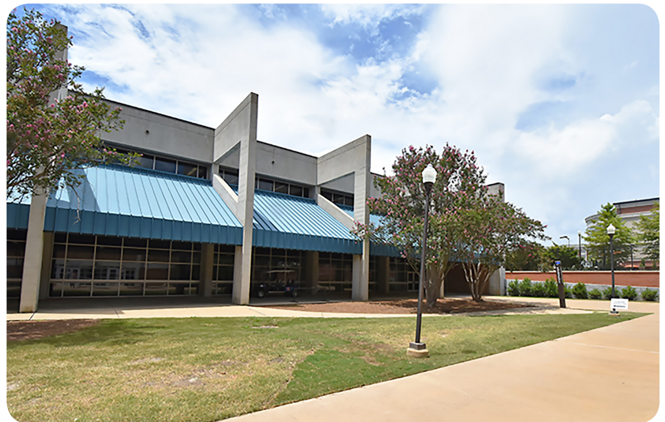
The area of the Student Activities Center where concessions will be built.
