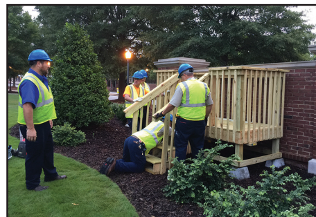
Platforms were set on bases in order to preserve the ground below.
