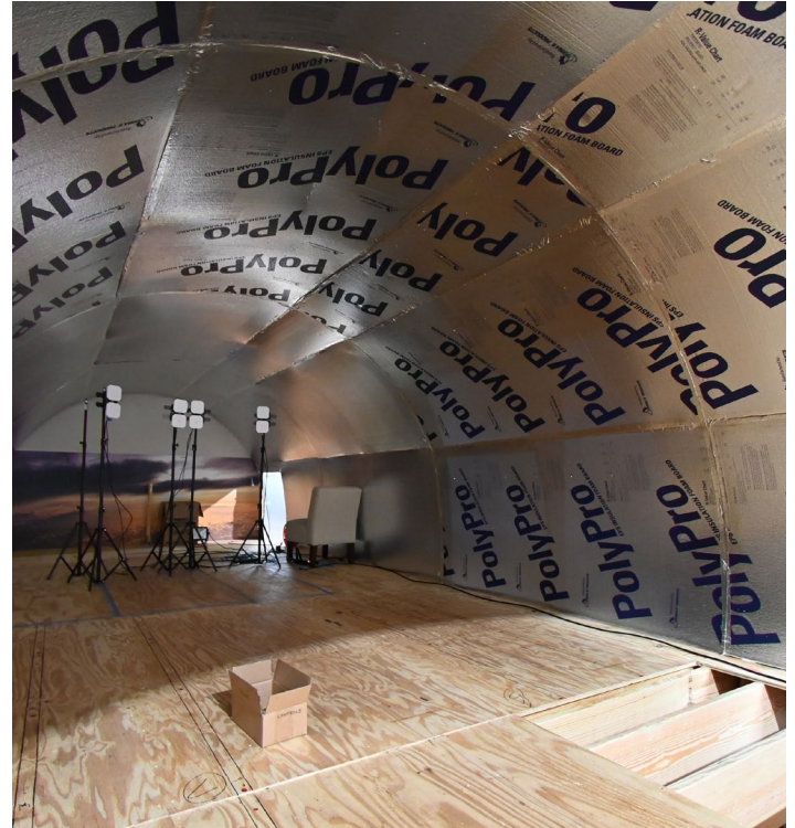
Insulation panels act as the skin of the fuselage. Next step—installing airplane seats.
