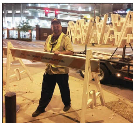
Johnny Brooks , Heavy Construction, placing barricades around campus. Heavy Construction begins placing barricades and cones at 5:30 a.m. on Friday mornings.
