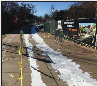
The solution was painted onto the concourse and left for two days.
