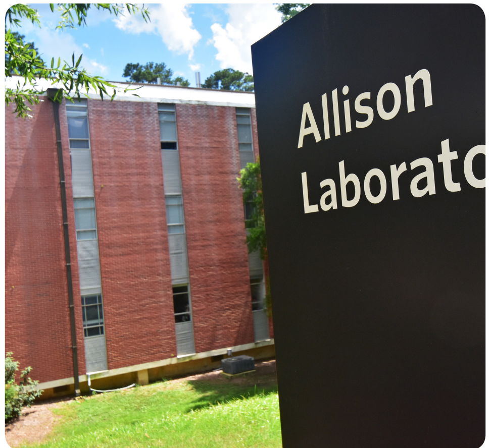
Allison Laboratory is scheduled to be demolished by May 2019.
