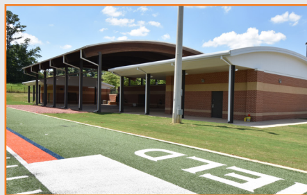
The Band Practice Complex project is ready for the Auburn University Marching Band to practice for the upcoming football season.
