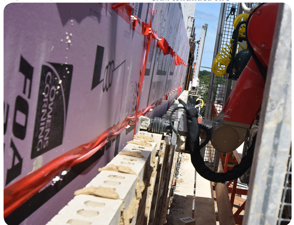
SAM has the ability to lay more than 3,000 bricks per day.
