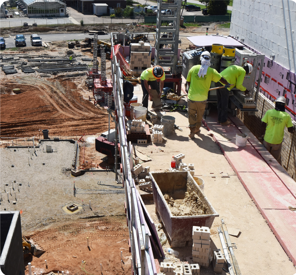
A small team allow SAM to continue working without requiring anyone to do anything too strenuous.
